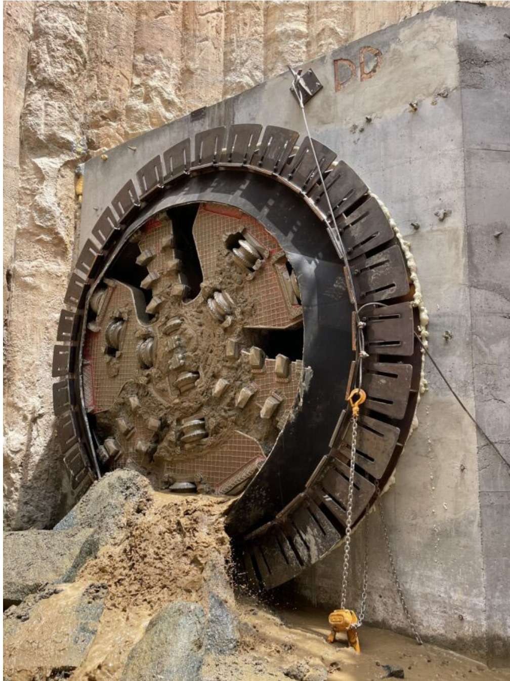
Perris Valley Pipeline—Hole-through TBM at second shaft
