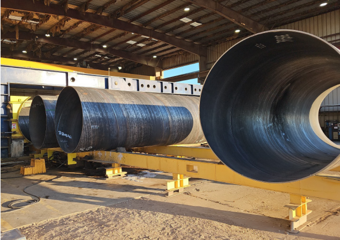
Sepulveda Feeder PCCP Rehabilitation Reach 2 81-inch Steel Liners in Line to be Hydro Tested
