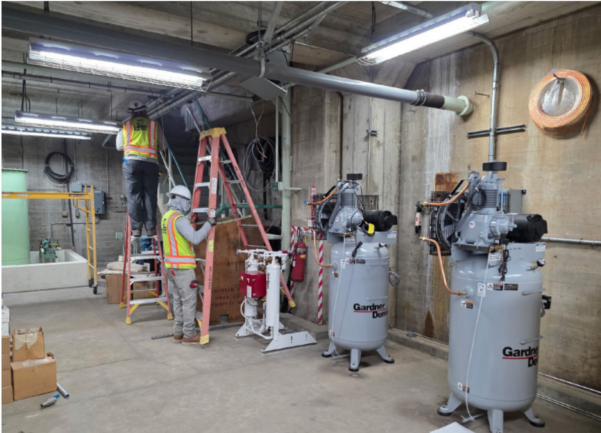
CRA Domestic Water Treatment System — Intake Pumping Plant Electrical Installation of Air Compressor and Dryer
