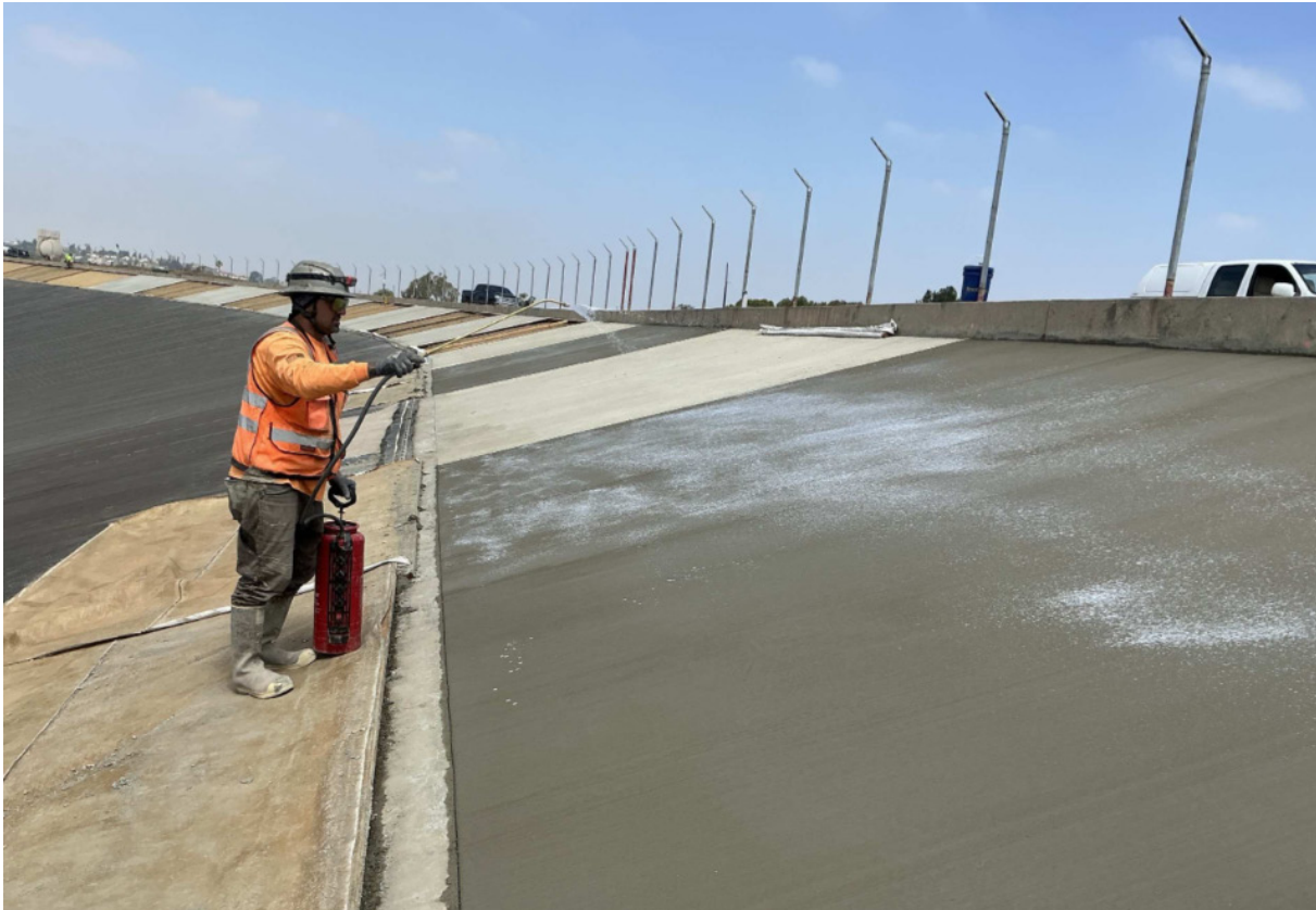
Garvey Reservoir Rehabilitation Applying Curing Compound on New Concrete Ribbon, Looking West
