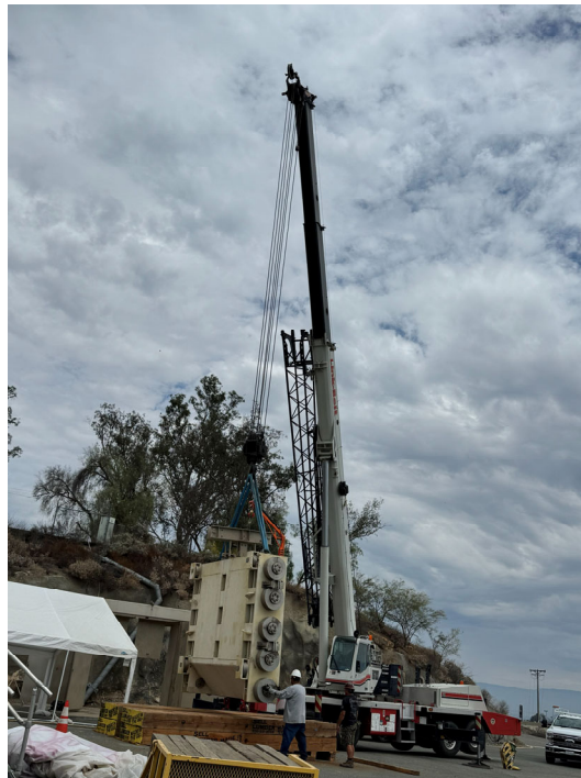
Staff positioning the gate after removal from the junction shaft at Lake Mathews.
