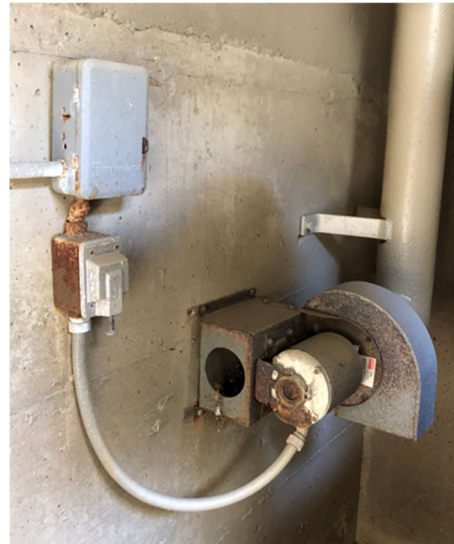
Power panel (left), and blower prior to repair (right).
