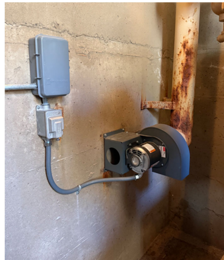
Newly installed power distribution panel (left), and blower after repair (right).
