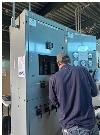
Staff installing the new HMI screen.
