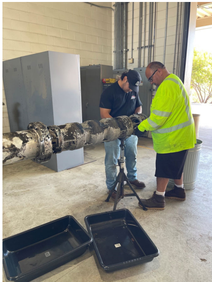
Staff rebuilding a vertical turbine pump at the Diemer plant.
