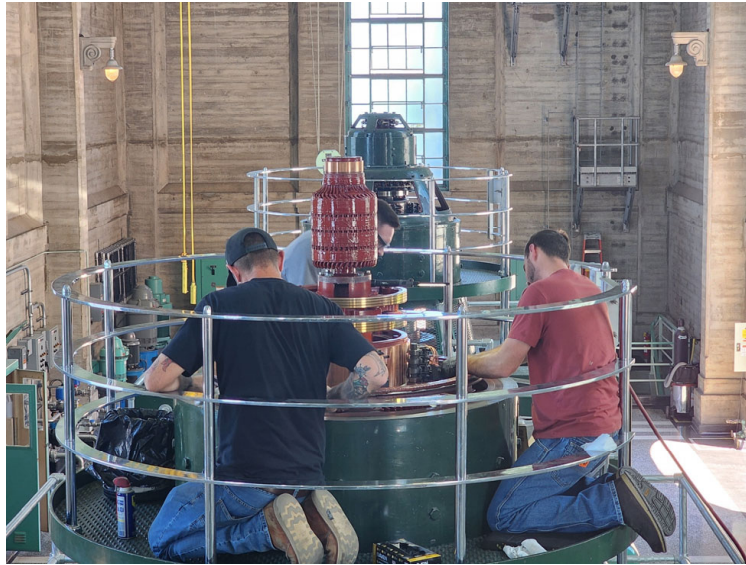
Staff installing a new exciter armature on Intake Unit 2.
