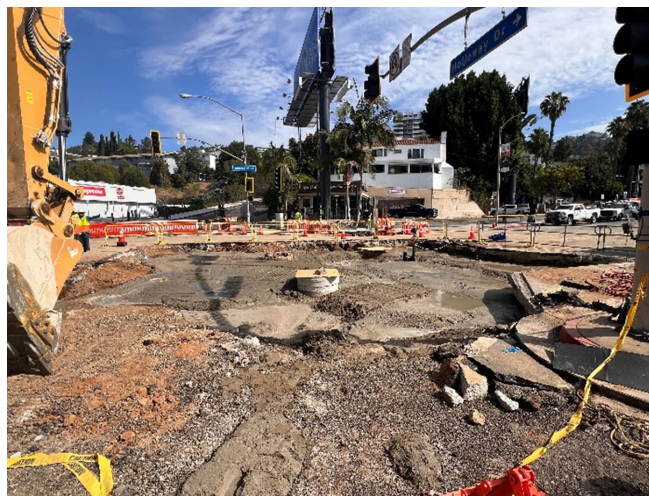
Completion of the slurry backfill of the excavation area over the Santa Monica Feeder in West Hollywood.
