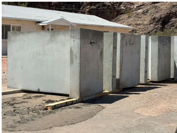
Concrete barrier sections being installed as a security upgrade.
