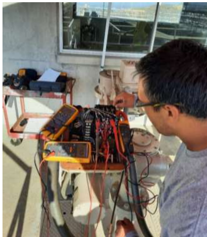
Staff troubleshooting an intermittent fault on a filter surface wash valve at the Diemer plant
