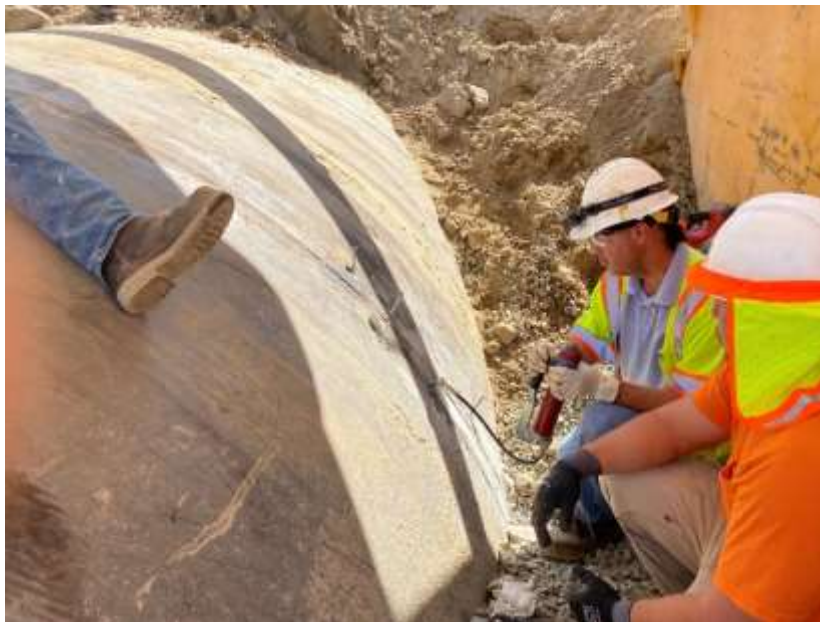
Staff injecting hydrophilic material into pipe joints on the Upper Feeder
