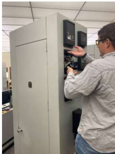
Desert staff calibrating a CRA motor relay
