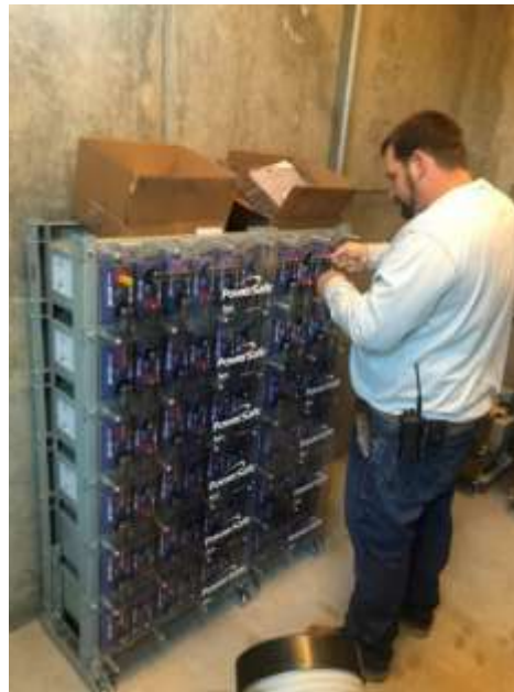
Staff installing new 120-volt DC battery system for the main electrical switchgear at the Skinner plant
