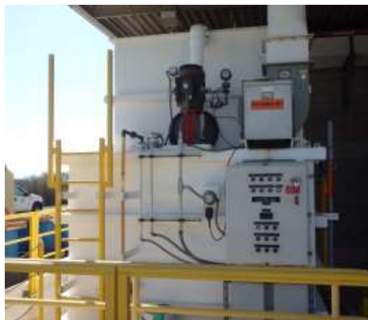
Chlorine scrubber at the Diemer plant
