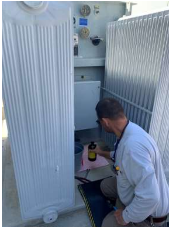
Staff taking an oil sample from a 4,160V transformer at the Skinner plant
