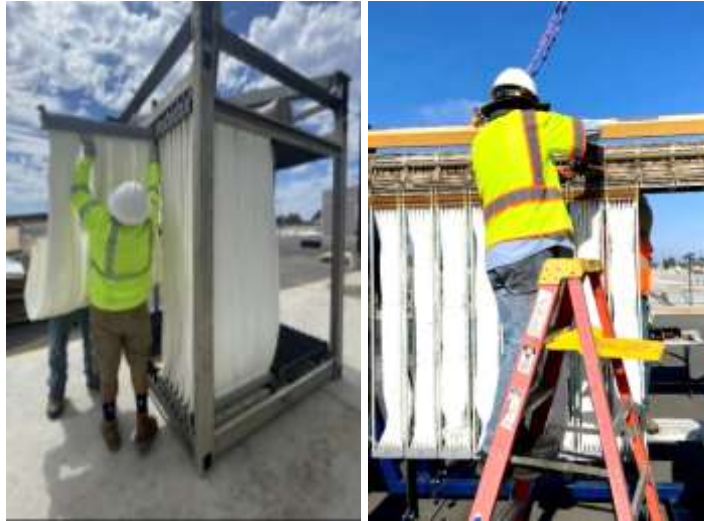
Staff installing new membranes in the bioreactors at the Pure Water Southern California demonstration plant
