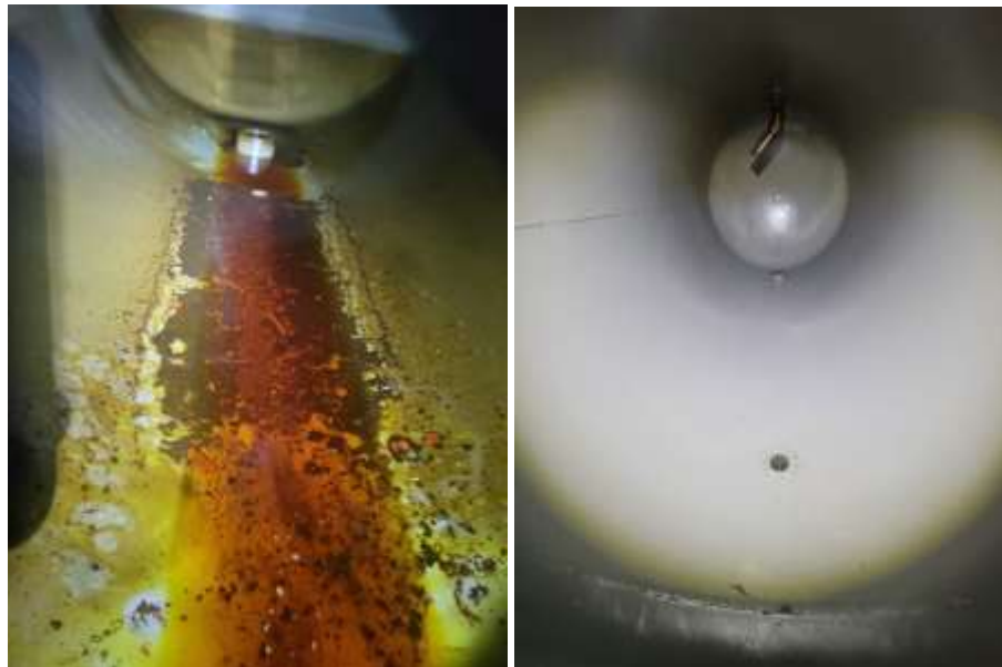
A lube oil sump tank before (left) and after (right) cleaning at Iron Mountain pumping plant
