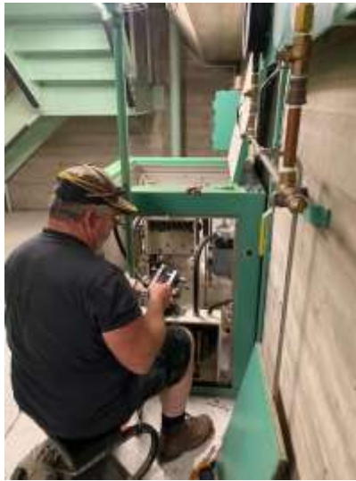
Staff troubleshooting a CRA main pump unit discharge valve pressure governor
