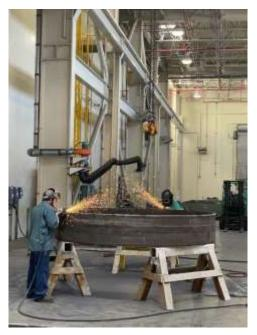
Staff welding new slip joint ring for Upper Feeder repairs
