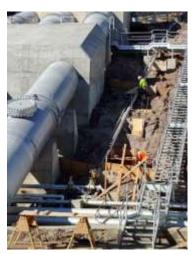
**CRA Domestic Water Treatment Plant System Replacement**—Contractor staff excavate for pipe rack concrete supports at Intake Pump Plant
