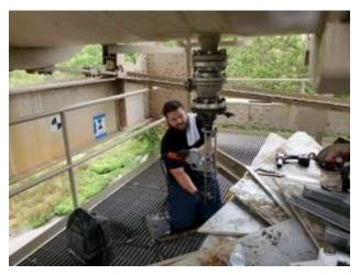
Contractor performing final hot tap of a flange and valve assembly on the Upper Feeder at the Santa Ana River bridge
