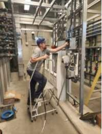
Staff installing SCADA cables (left) and power cables (right) for an additional chlorinator at the Weymouth plant
