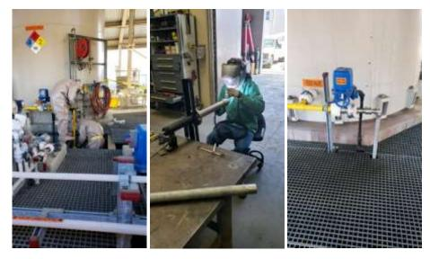
Staff removing damaged piping (left) and fabricating new piping (center); and new piping installed (right) for a chemical feed system at the Weymouth plant
