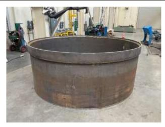
Fabrication of new 113-inch slip joint to replace leaky bellows joint on Upper Feeder
