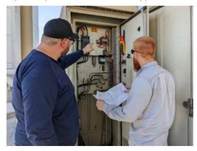
Electrical apprentice and journey installing a new variable frequency drive at the Diemer plant Objective #13 Ensure Accurate Billing Infrastructure.
