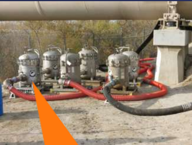
Quagga Filters for Dewatering
