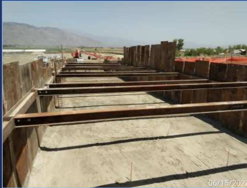
Supported Excavation for ERDIP Pipe
