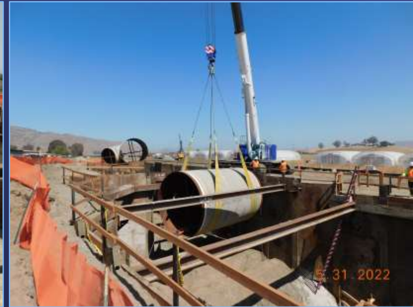
Placement of Steel Transition Pipe
