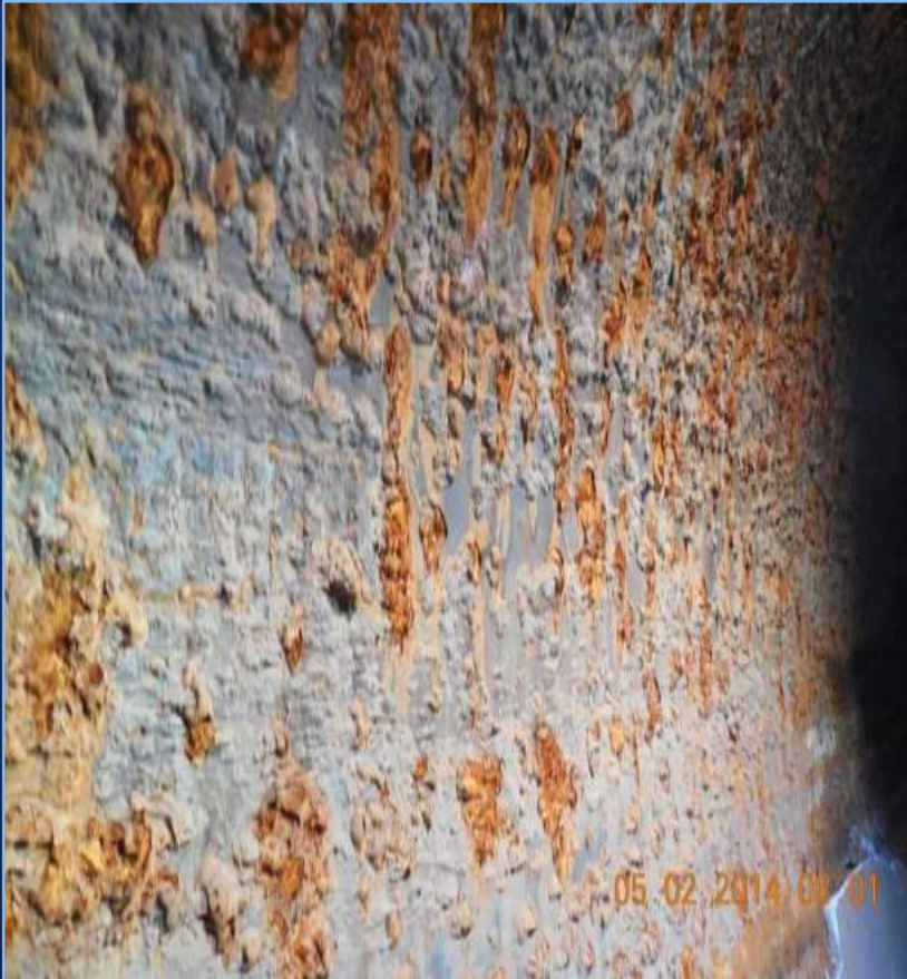
Condition Before Abrasive Blasting
