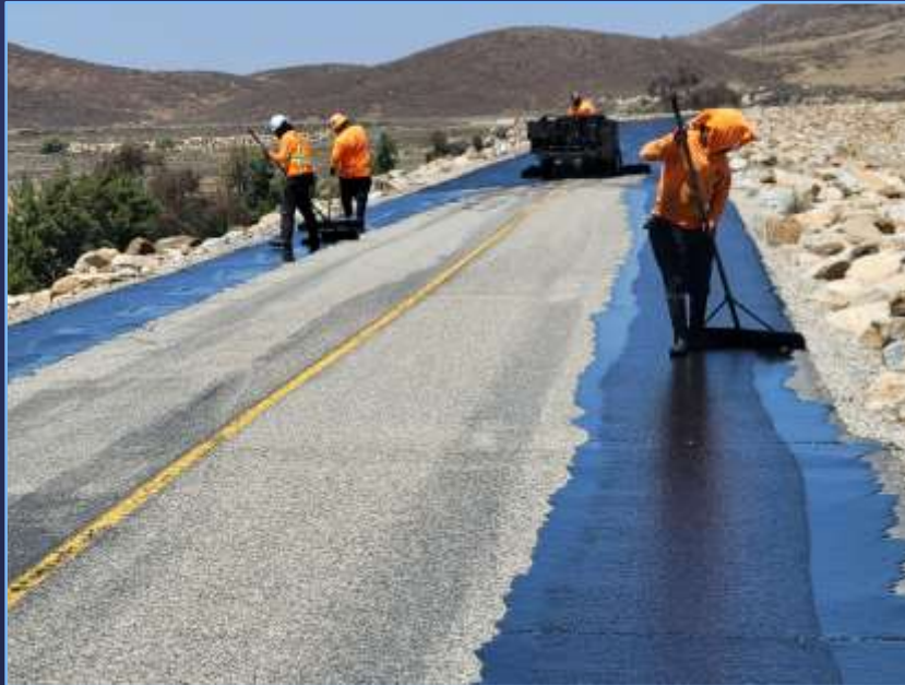
Slurry Paving of Dam Access Road
