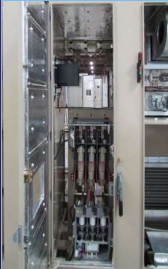
Disconnect Switch with Fuses
