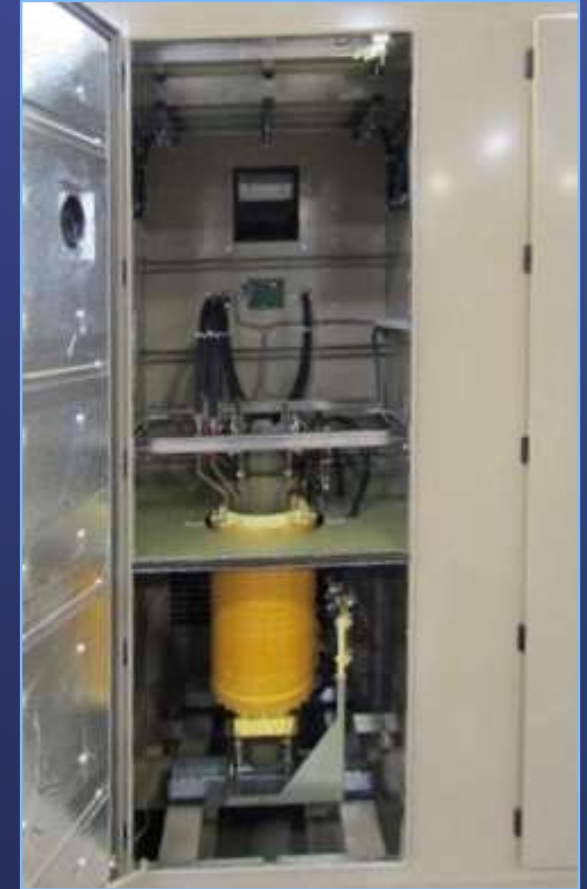
High Voltage Transformer
