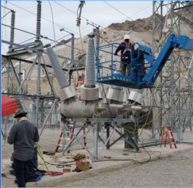
Staff performing electrical coordination on a 230kV circuit breaker
