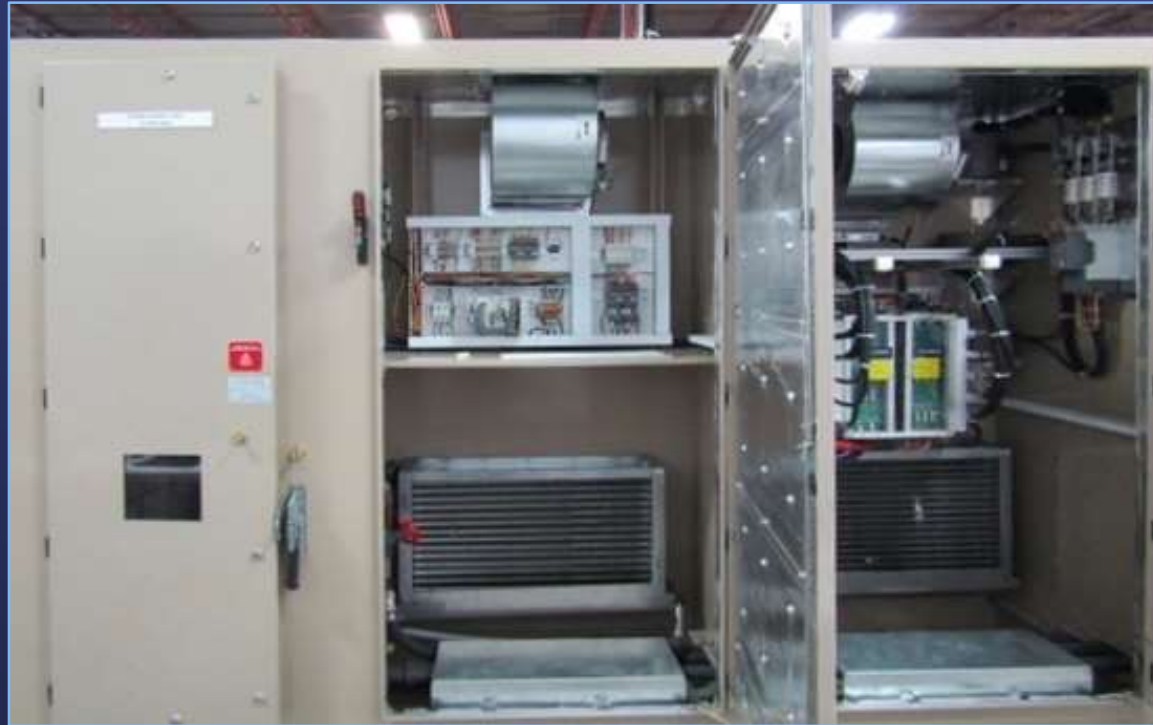
Cooling Water & Feed Section
