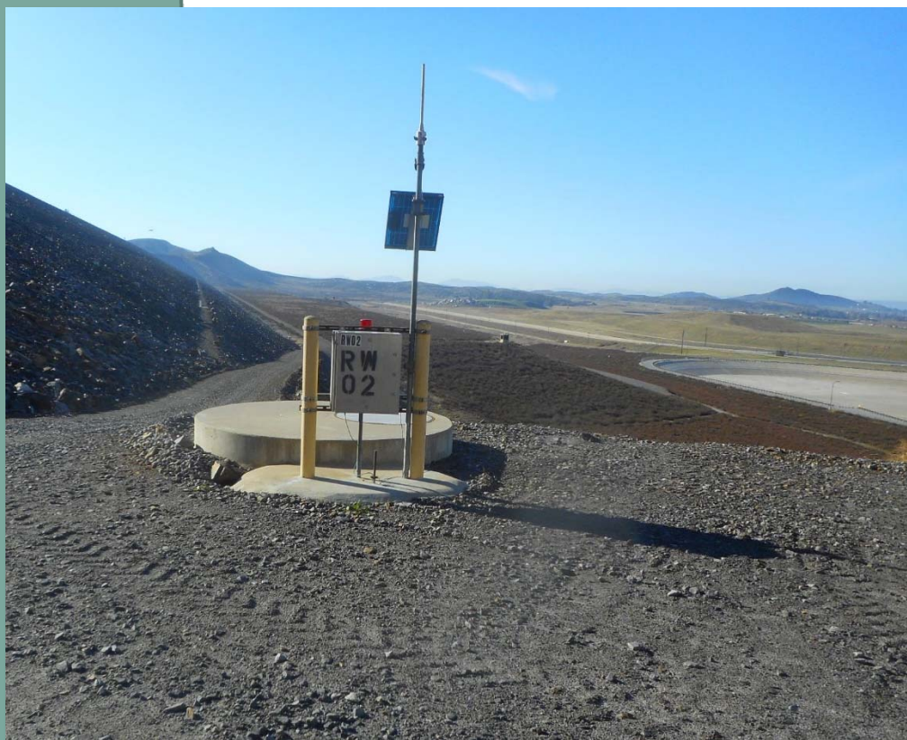
Existing Diamond Valley Lake west dam remote monitoring station
