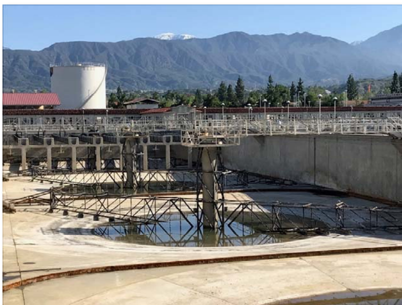
Example of major mechanical equipment to be replaced including mechanical rotating rake at Basin 6 of the Weymouth plant
