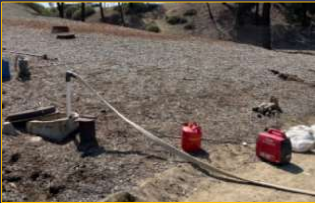
Small portable generator for dewatering at Skinner Water Treatment Plant
