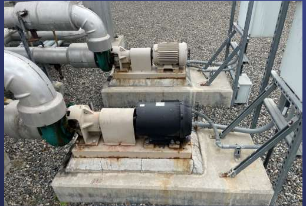
Existing chilled water pumps
