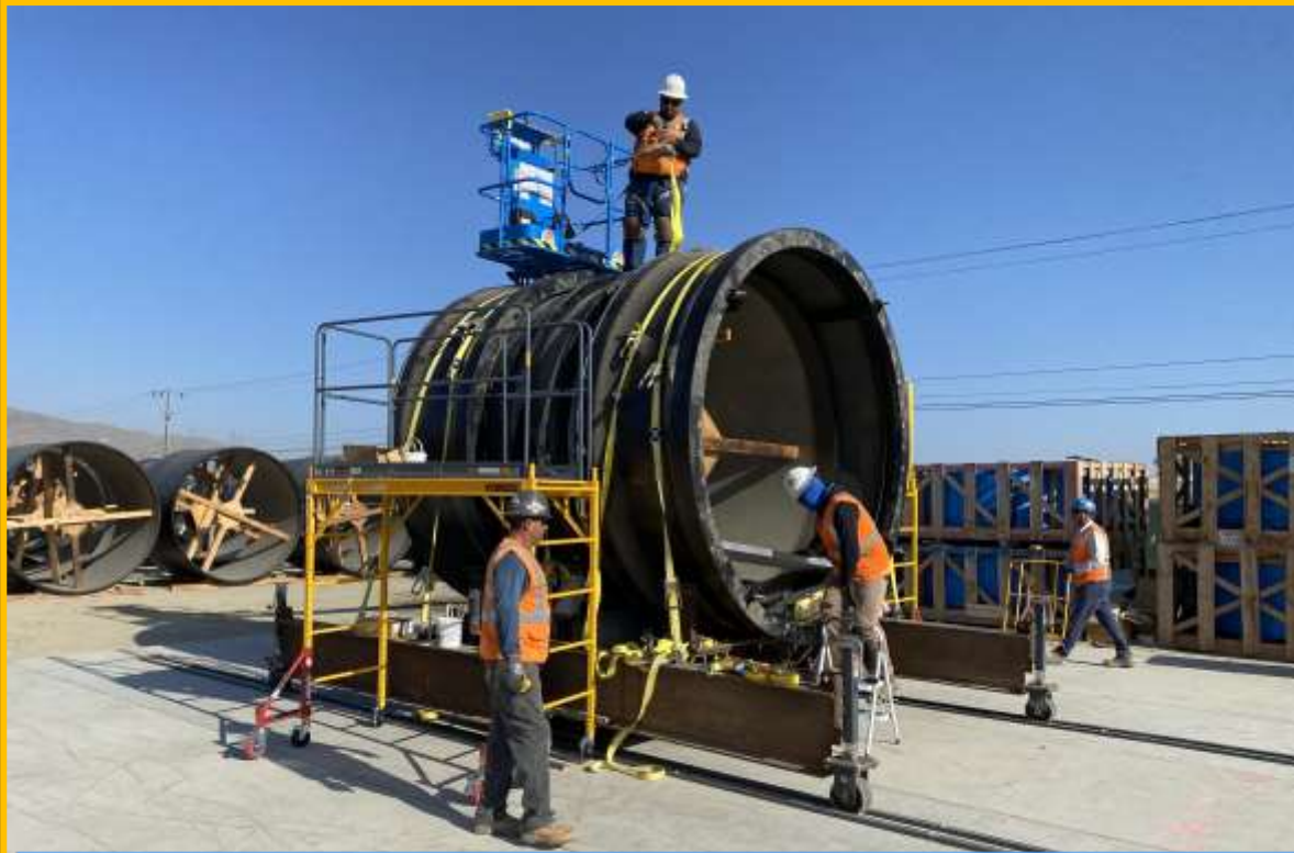
Field Assembly of Kubota ERDIP Sections
