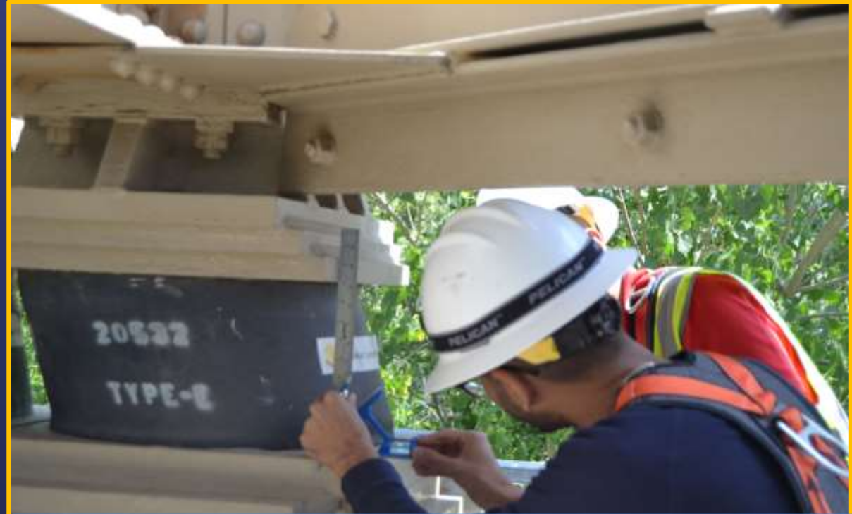
Bridge Base Isolator Inspection
