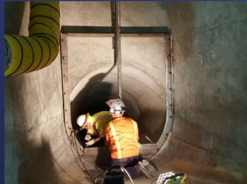
Palos Verdes Reservoir Bulkhead Installations
