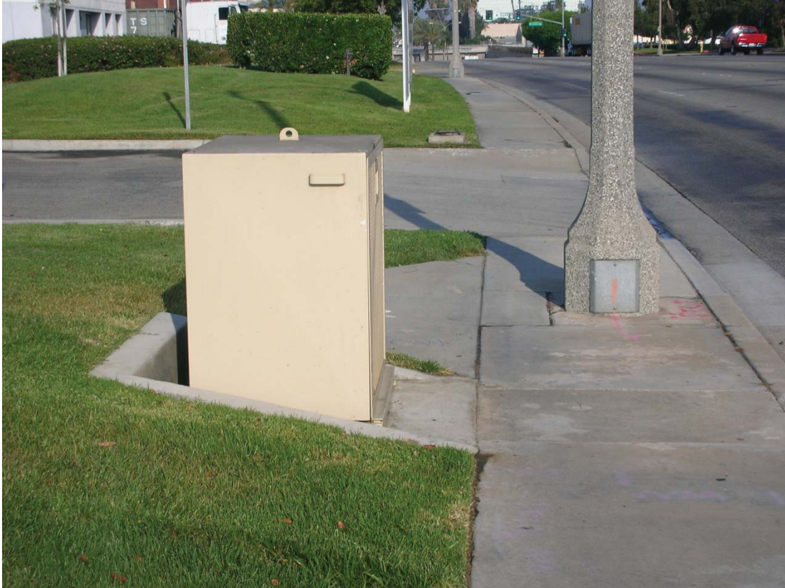
Figure 3-6. Typical Above-ground Valve Enclosure
