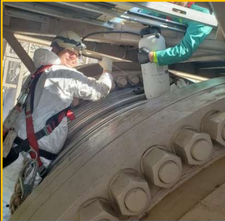
Liquid Penetrant Tests
