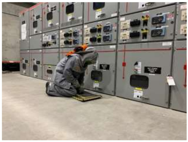
Staff isolating equipment for maintenance at Skinner WTP
