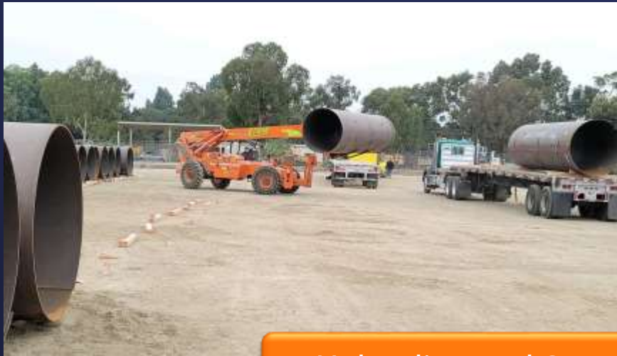
Unloading and Storage of steel liner for Reaches 3A and 3B
