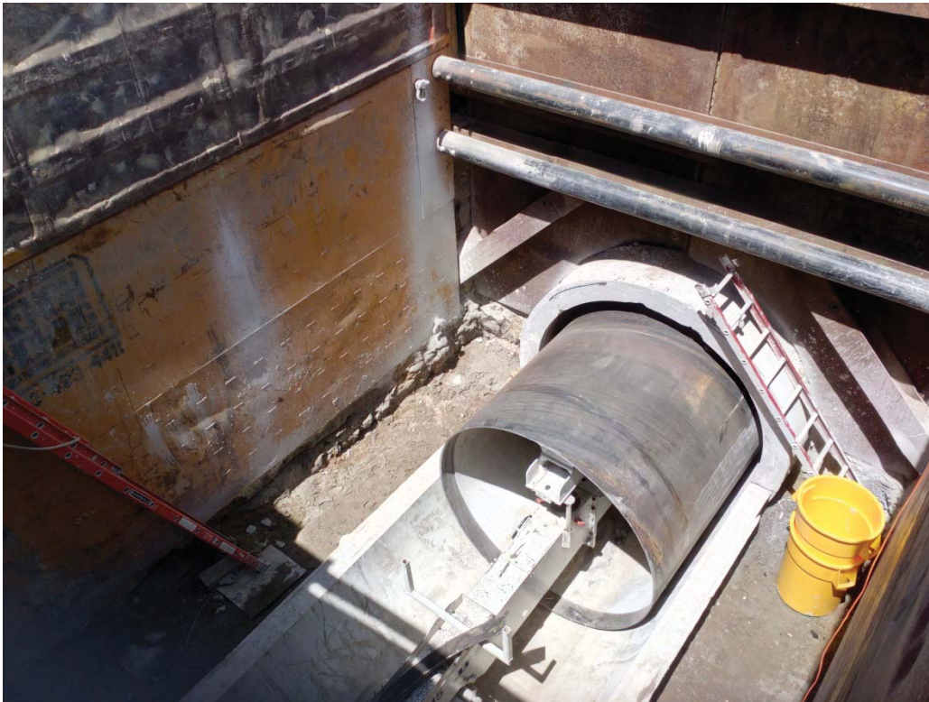
Figure 3-4. Steel Sliplining with Non-Collapsed Pipe in Progress
