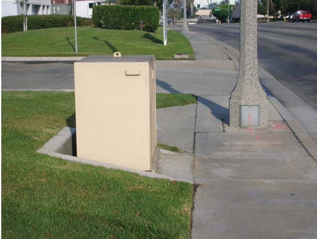
Figure 4. Typical Aboveground Valve Enclosure
