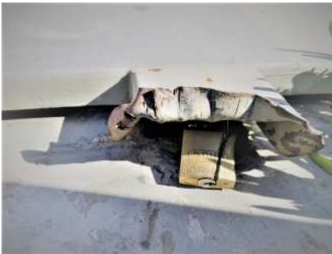
Problem: Vandals attacked substructure lid & lock
