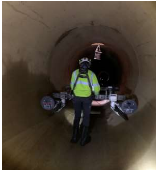
Staff performing an electromagnetic inspection of the Sepulveda Feeder
