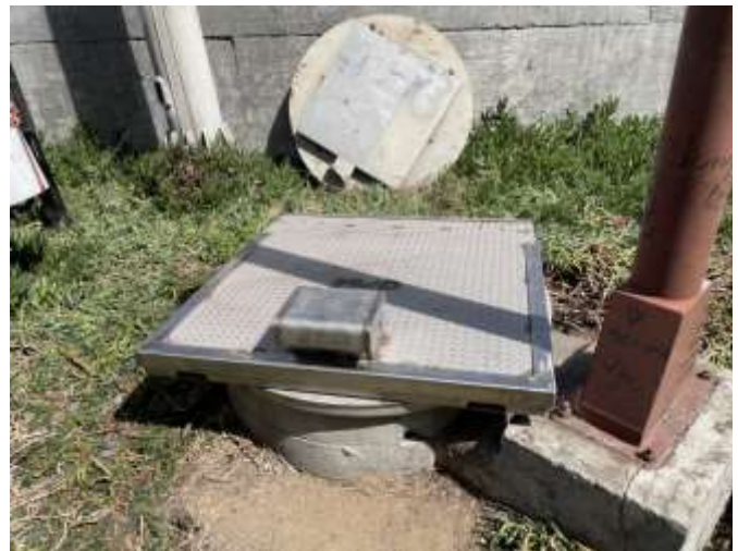
Solution: Stainless-steel, reinforced, double-lock lid
