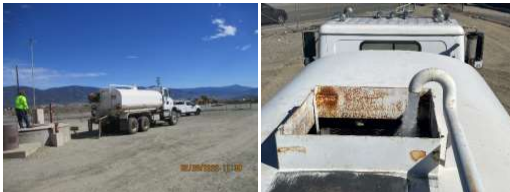
Staff filling water truck from manhole structure (left) and applying air gap for filling water truck (right) in the field
