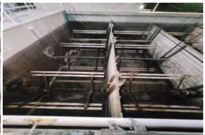
Accumulated solids before cleaning (left) and after removal (right) from the WWRP at the Jensen plant
