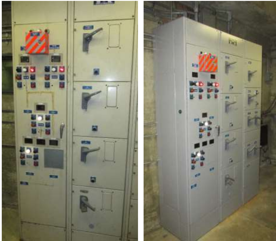
Control cabinet before (left) and after (right) coating at Irvine Pressure Regulating Structure on the Orange County Feeder
