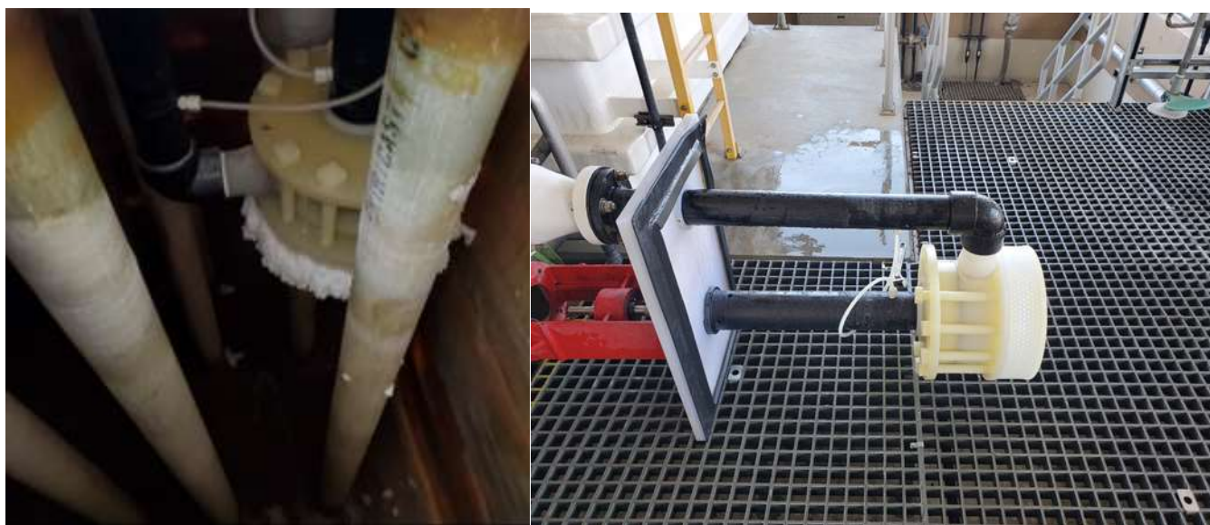
Chlorine scrubber pump before (left) and after (right) acid wash cleaning at the Skinner Plant
