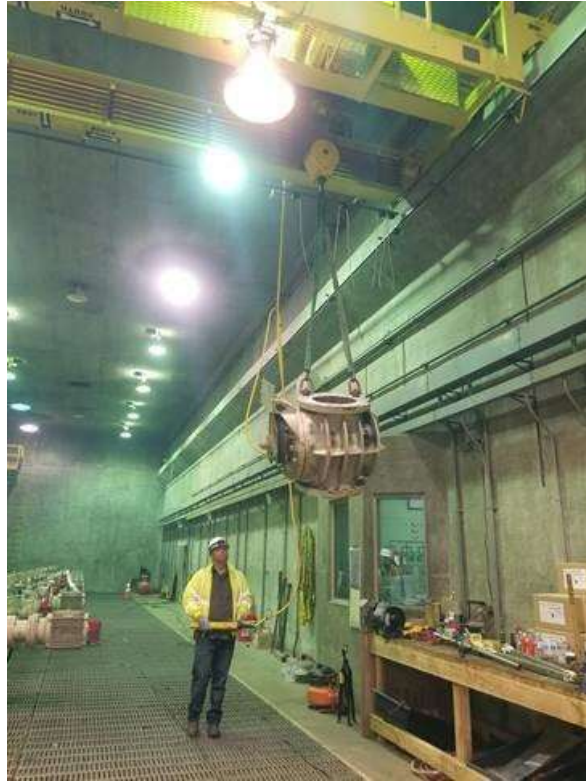
Staff removing the existing plug valve at the Venice PCS
