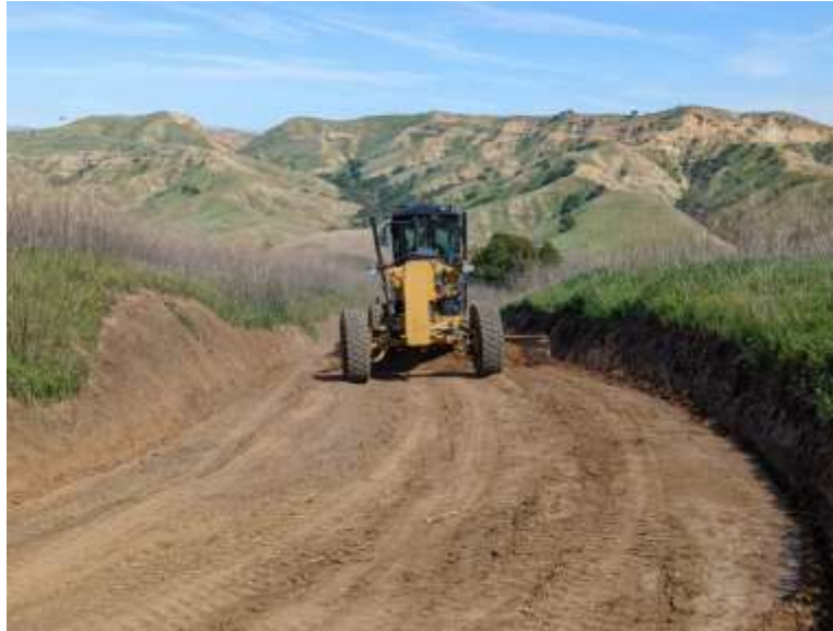
Staff using a motor grader for patrol road grading along the Lower Feeder
