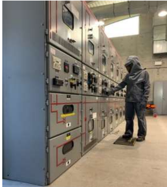
Staff performing high-voltage switching wearing an arc flash protection suit at the Skinner plant
