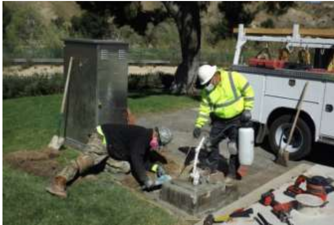
Staff removing damaged sections of concrete base for repairs to cathodic protection equipment along the Lower Feeder
