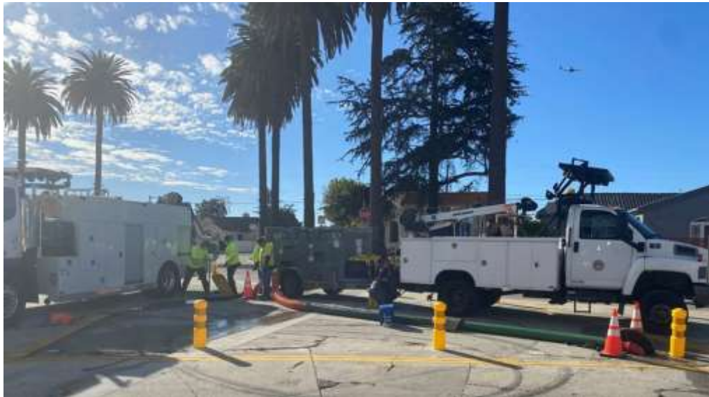
Staff dewatering a pump-well structure during the Sepulveda Feeder shutdown
