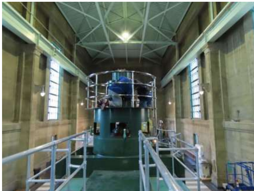
Staff performing exciter maintenance on a 12,500 hp pump during the CRA shutdown
