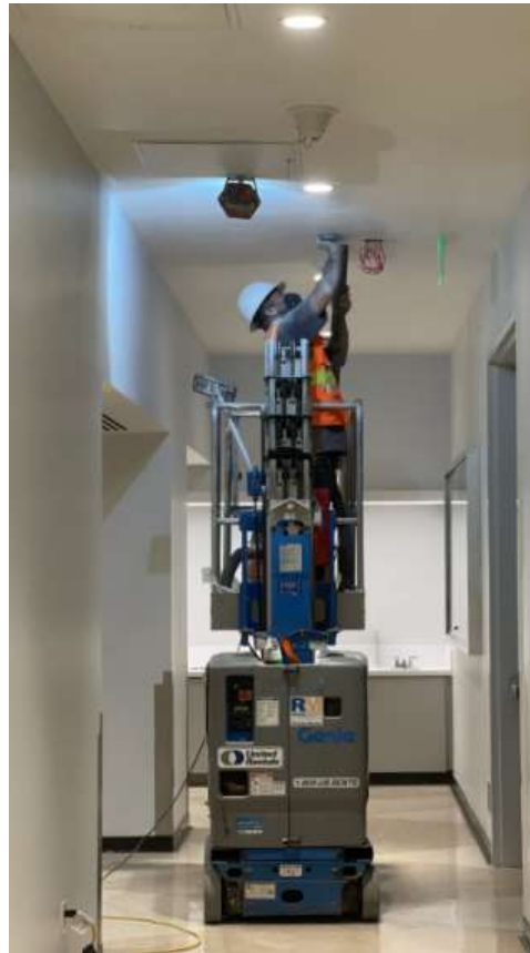
Headquarters Building Improvements Installation of fire alarm devices in cafeteria
