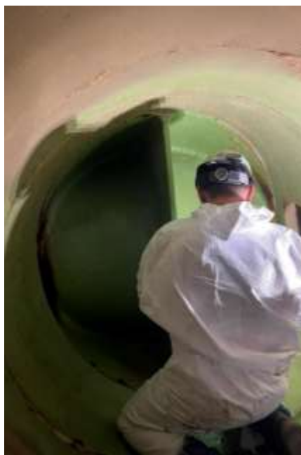
Staff disassembling a large conical plug valve for the CRAMPR project
