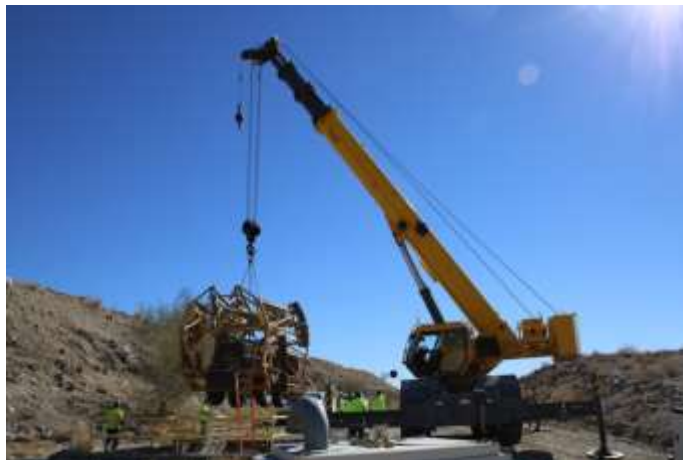
Tunnel Cleaning Machine being lowered into the CRA
