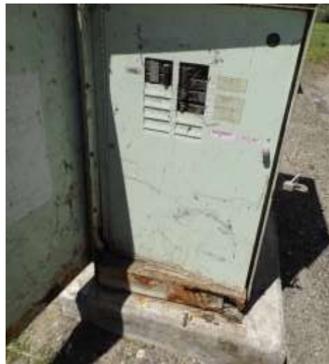
Damaged metering pedestal and concrete base along the Lower Feeder
