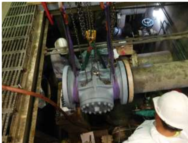
Staff installing the new plug valve at the Venice PCS
