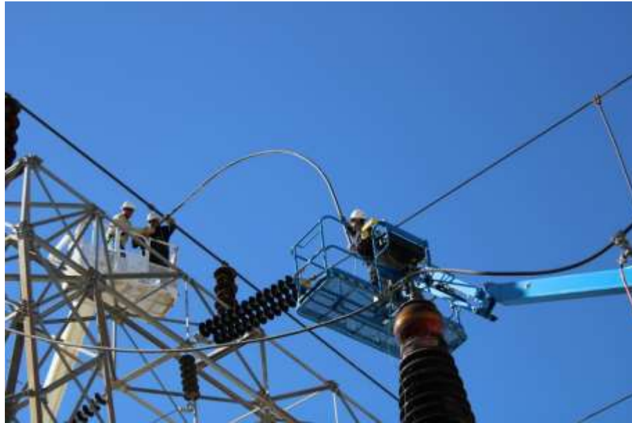
Staff removing the 230kV feed to the spare transformer at the Gene pumping plant
