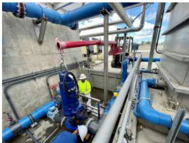
Reinstalling a repaired return activated sludge pump at the RRWAPC demonstration plant
