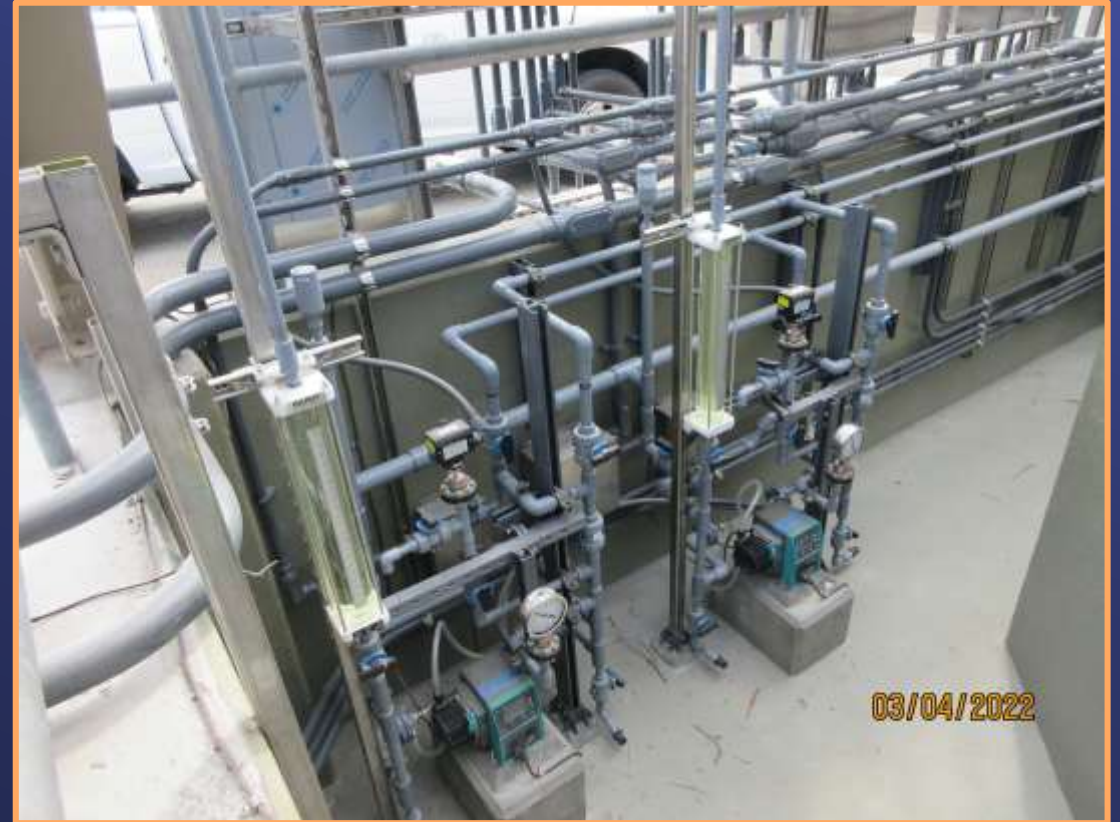
Temporary Hypochlorite Feed System Installed and Operational
