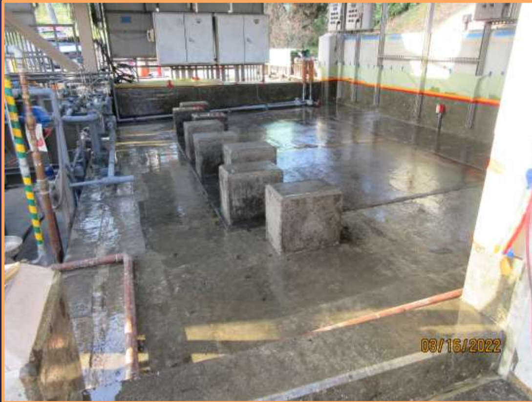
New Pump Pedestals and Control Panels Installed and Coated
