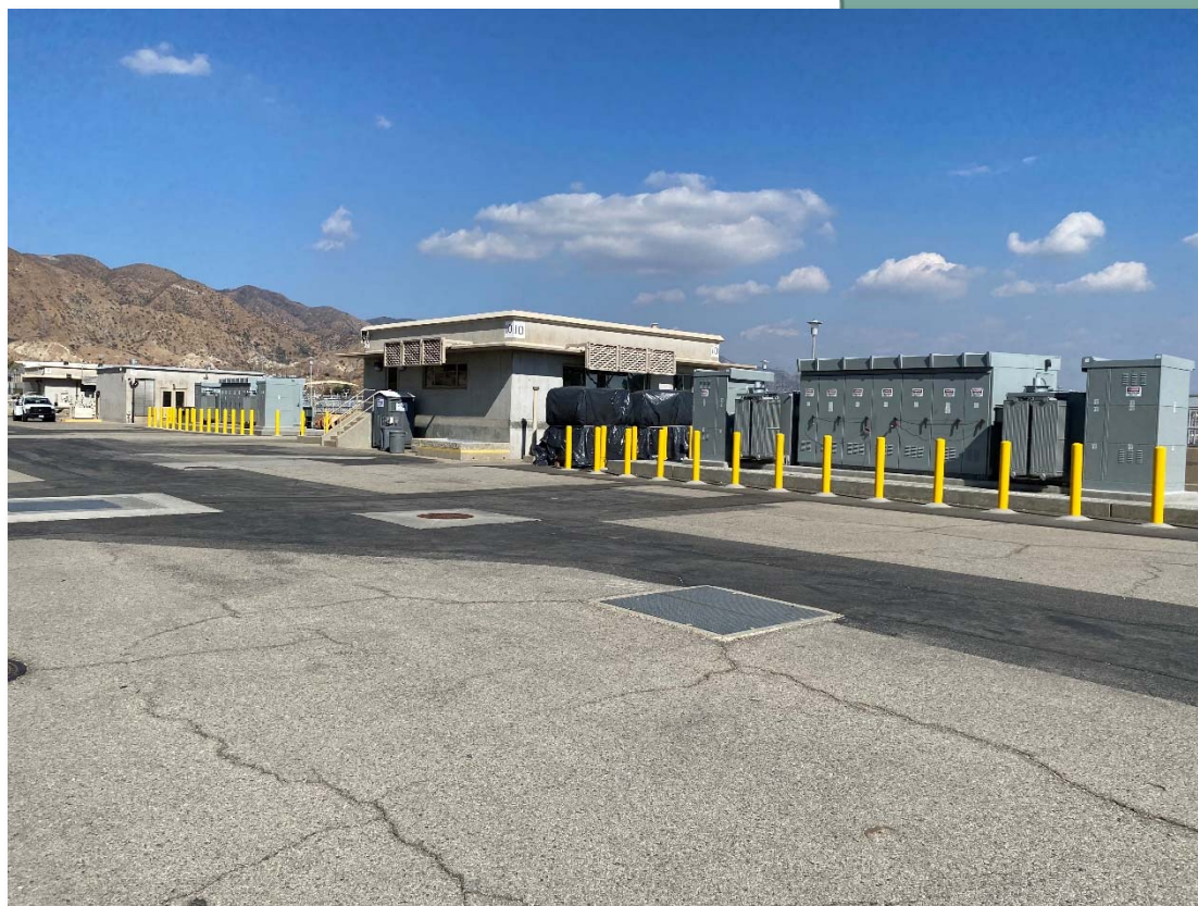
Completed unit substations at the Jensen plant
