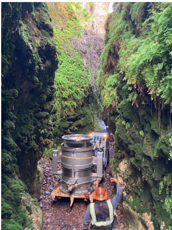
New fixed cone discharge valve being transported to the Gene Wash Dam Valve House
