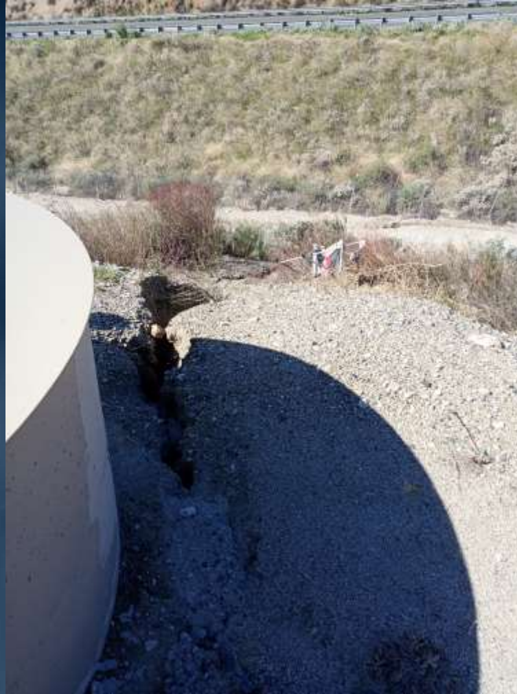
Erosion Adjacent to Accessway
