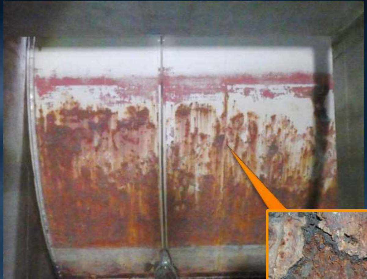
Corrosion on the V-06 radial gate
