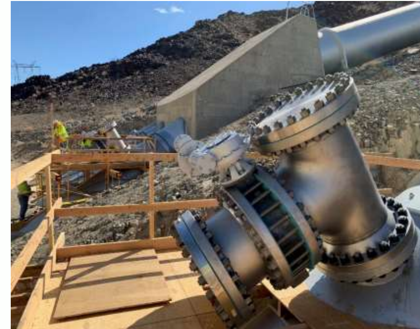
Branch tee installation at the Eagle Mountain Pumping Plant
