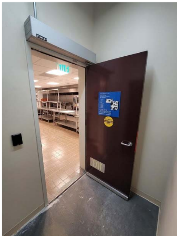
Completed power door assist mechanism
