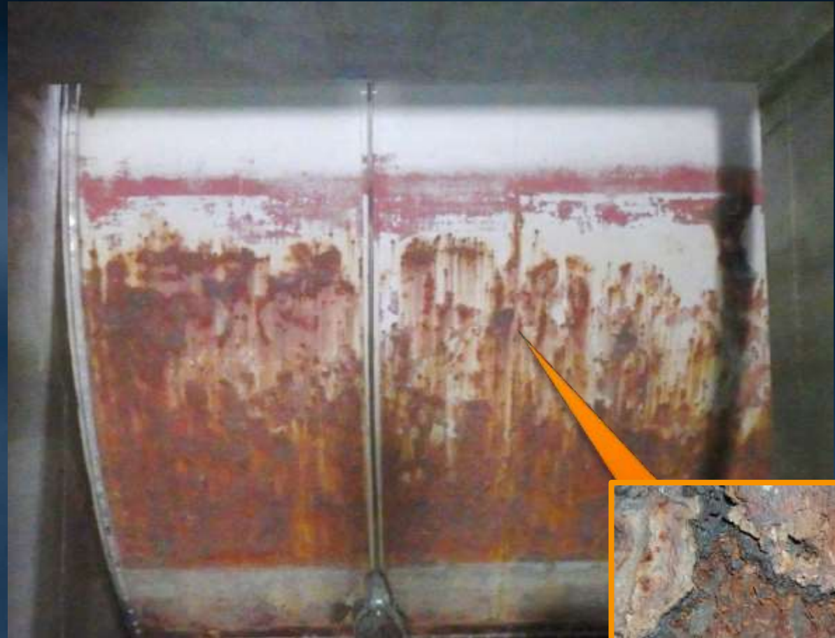
Corrosion on the V-06 radial gate
