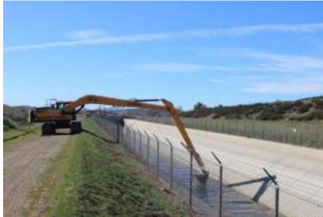
Staff removing silt and debris from the San Diego Canal
