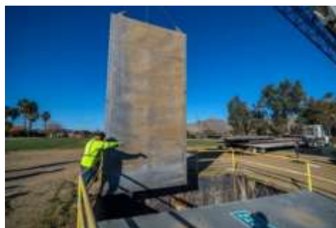
Staff removing lids at Lakeview Siphon inlet transition to install isolation gate
