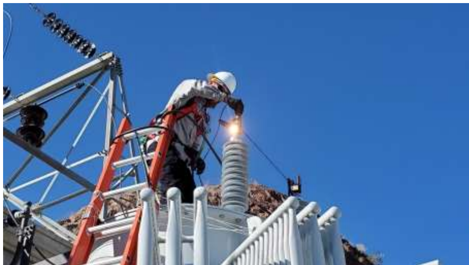
Class of 2023 electrical apprentice performing routine high-voltage maintenance test at Whitsett pumping plant (Note: The light is sun's reflection, not electrical arc)
