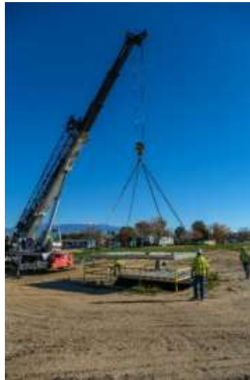
Staff lifting gate to be installed for safe isolation of the work zone in the Lakeview Siphon
