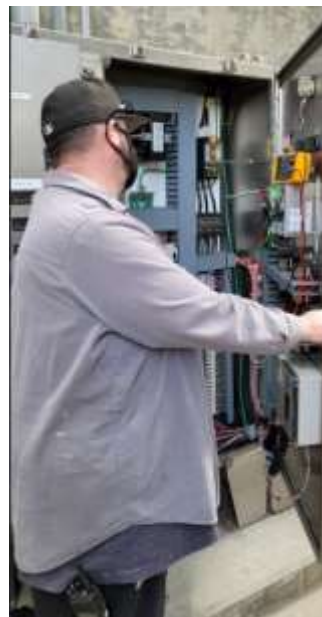
Staff verifying signal output for the solids hopper at the Weymouth plant
