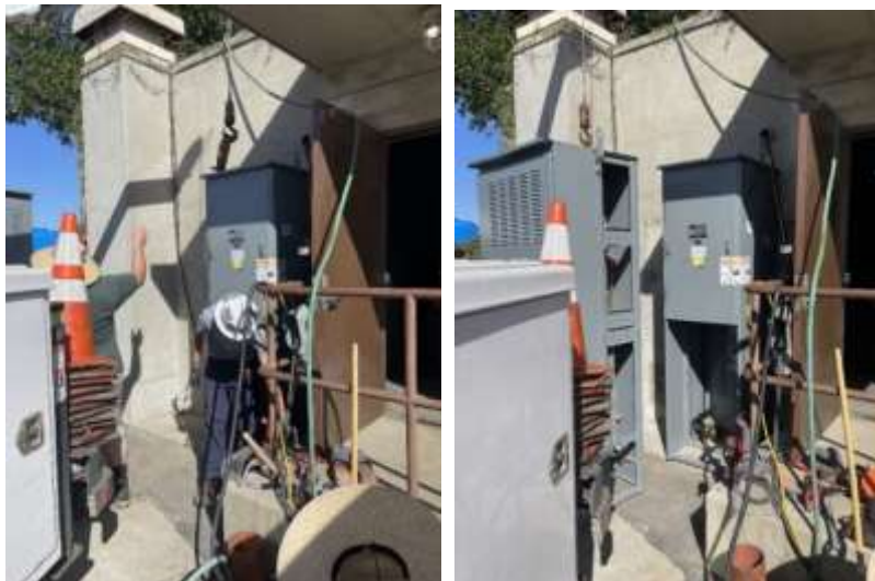
Staff setting new utility pull section (left) and completed pull section and 480-volt panel (right) at San Gabriel PCS
