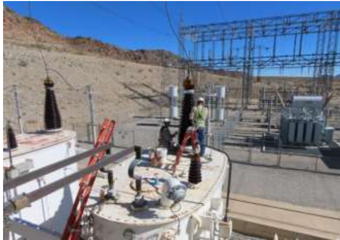
Staff performing transformer bushing maintenance at Hinds pumping plant
