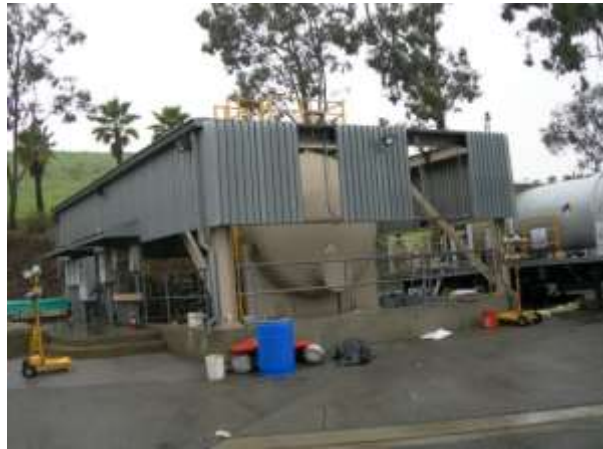
Temporary sodium hypochlorite feed system at Garvey Reservoir
