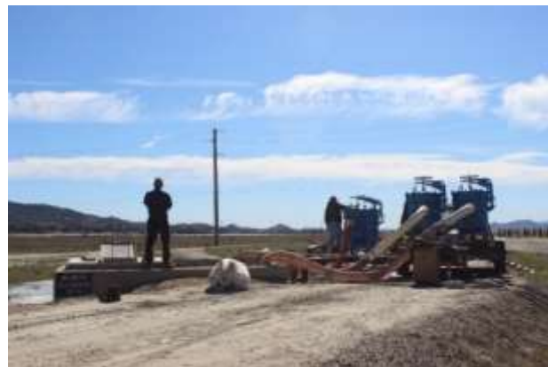
Staff monitoring quagga mussel filters during discharge of raw CRA water ahead of Lakeview Siphon work
