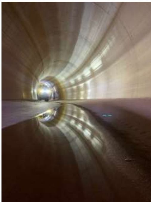
Clean, smooth canal walls after the tunnel cleaning machine passes
