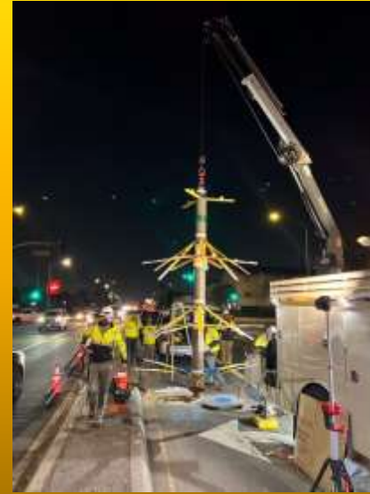
PCCP Inspection Equipment
