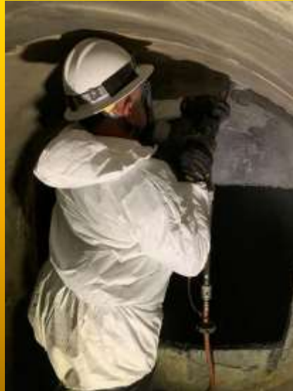
Staff Removing Bulkhead
