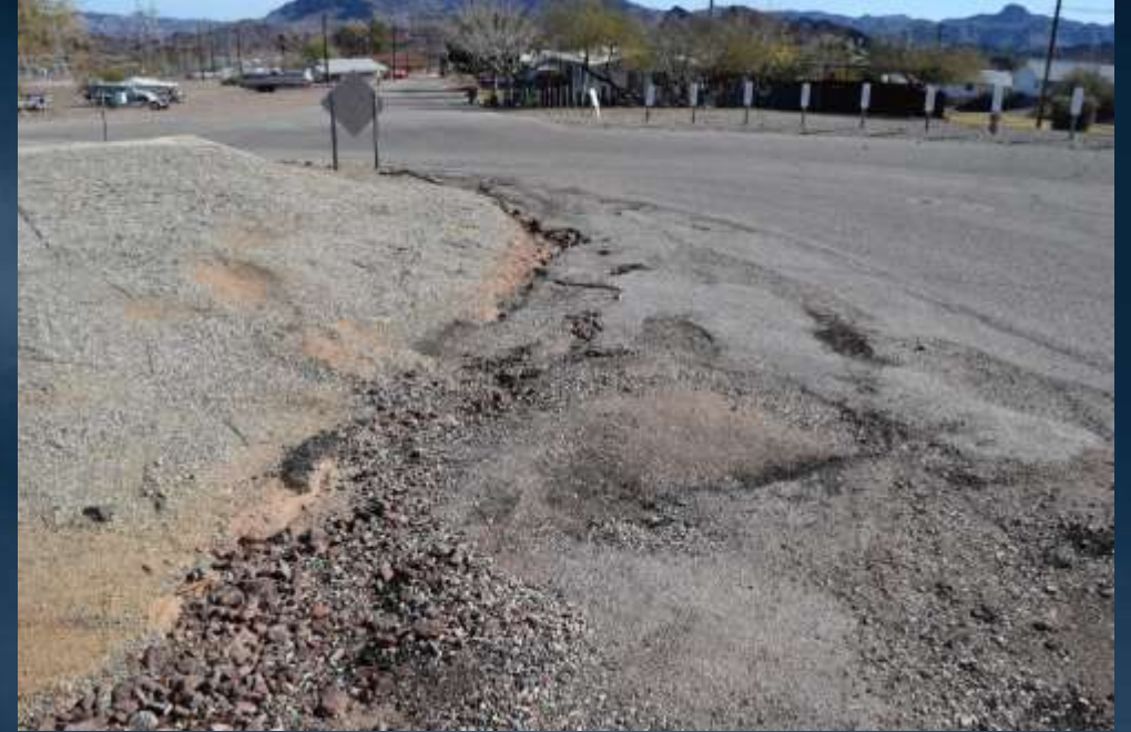
Deteriorated asphalt pavement at Gene Pumping Plant
