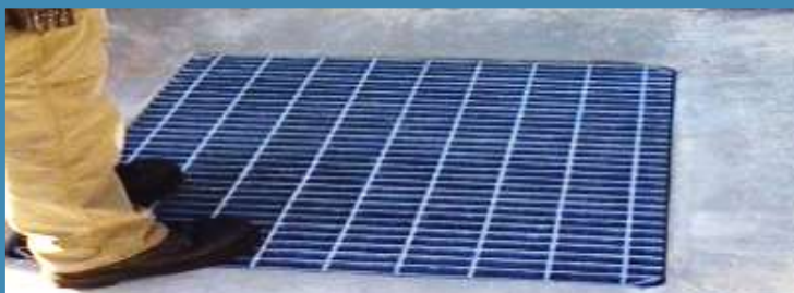
Mills Replaced Plastic Grate with Steel Grating
