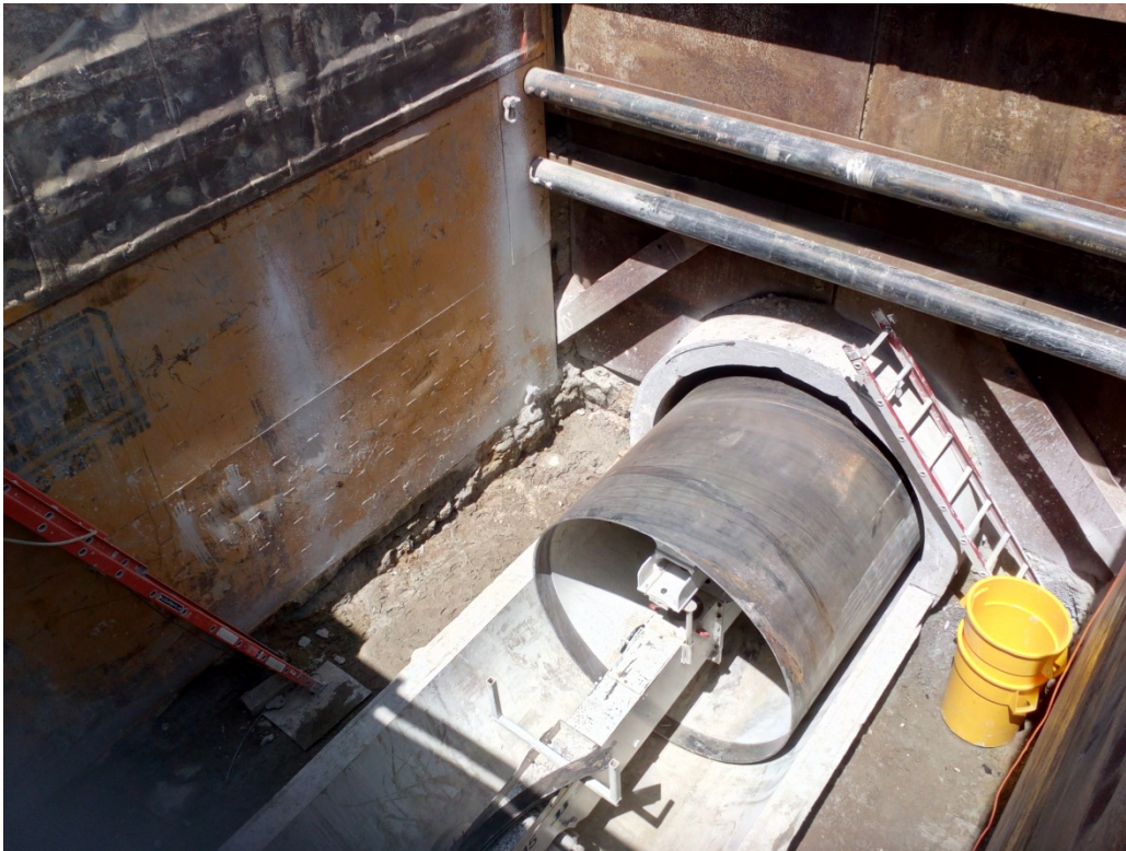
Figure 3-4. Steel Sliplining with Non-Collapsed Pipe in Progress
