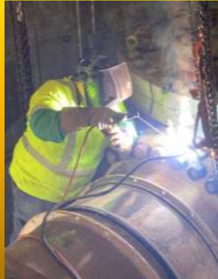
Staff Welding Lifting Eyes
