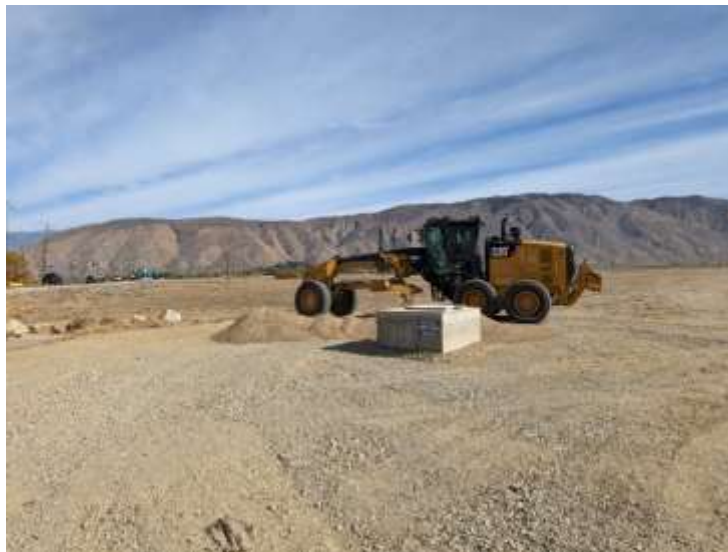
Motor grader placing material around structure along CRA patrol roads in San Jacinto
