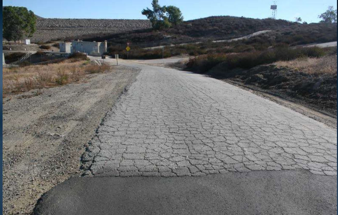
Skinner Plant Lower Patrol Road Deterioration
