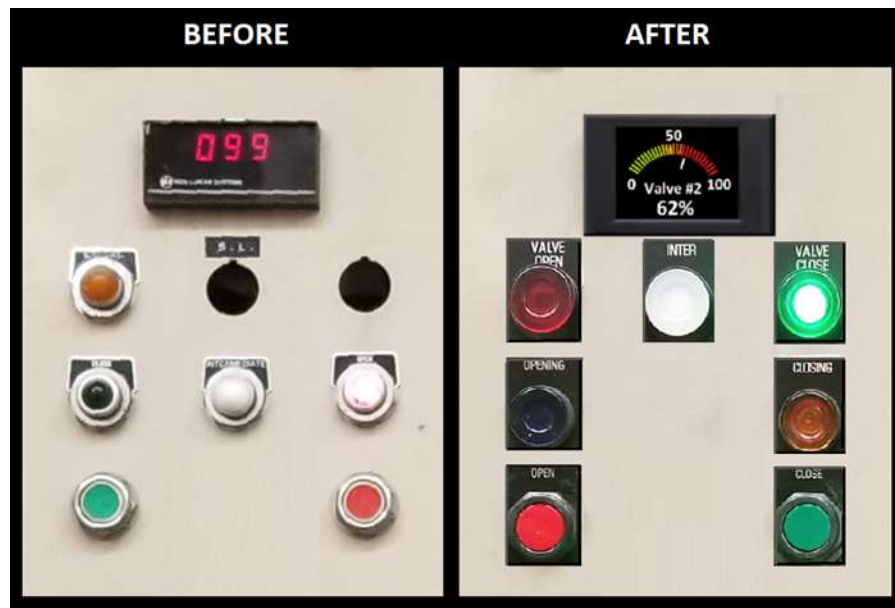
Santiago Control Tower monitoring instrumentation before (left) and after (right) replacement
