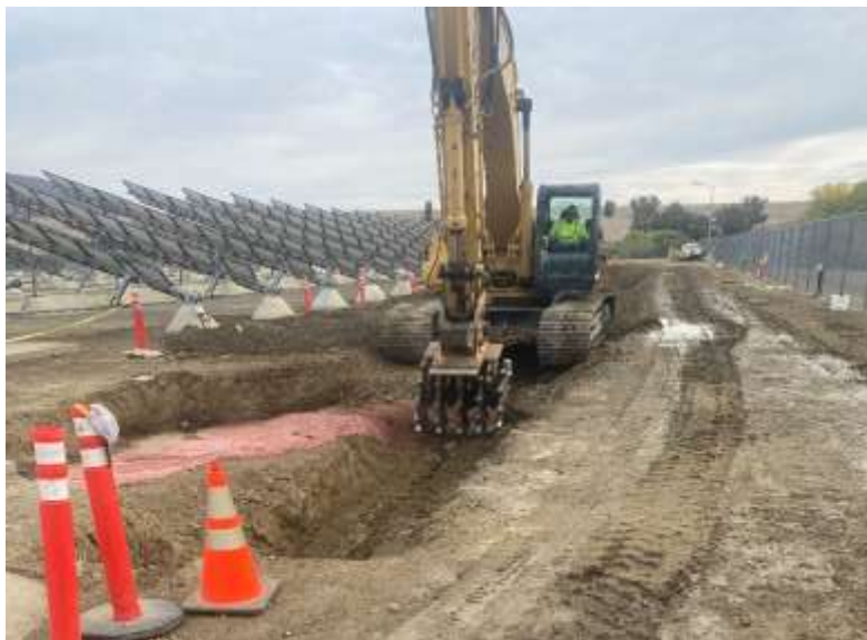
Excavator with compaction wheel backfilling trench at the Skinner plant
