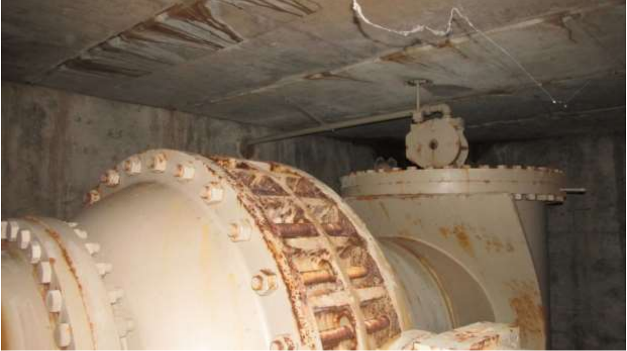
Service connections OC-68 and OC-69 structure before coating maintenance
