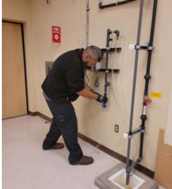
Staff installing sample and drain lines for a particle counter at the Weymouth plant
