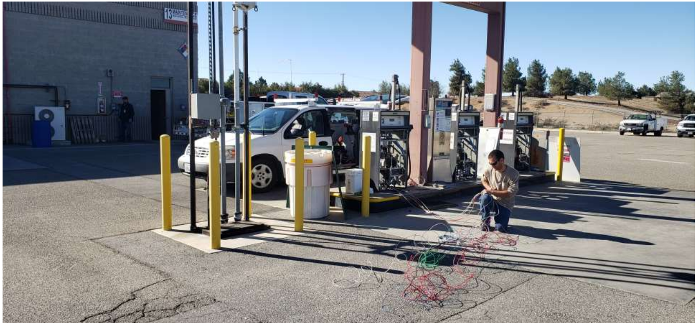
Staff pulling wire for dedicated circuits for new card readers at the Mills plant fuel island
