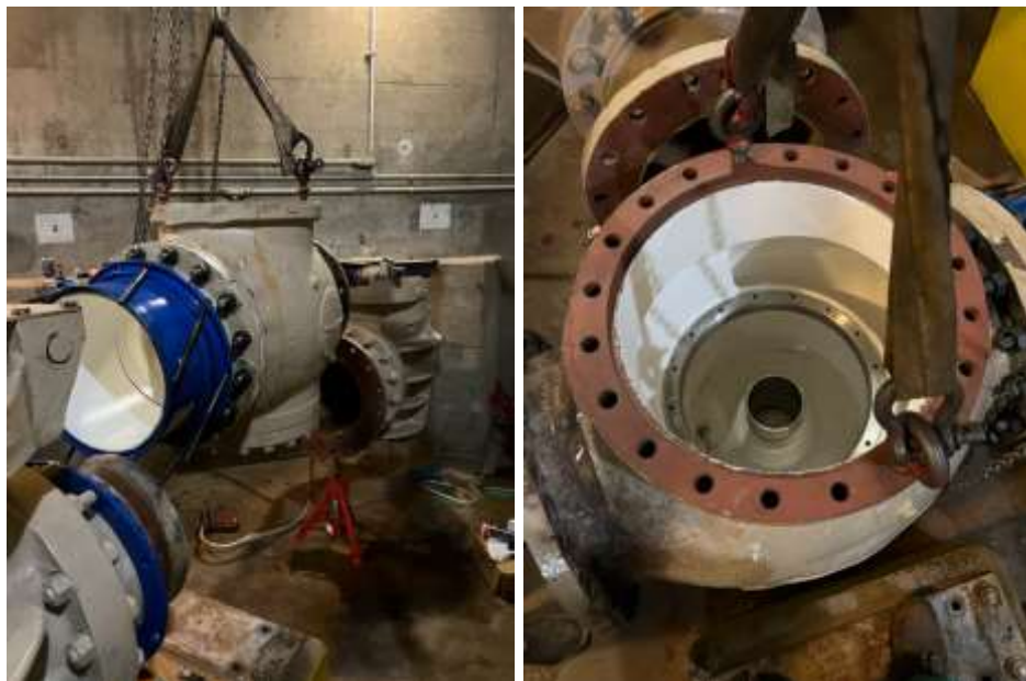
Installed globe valve body with refurbished internal coatings at the Cohasset PRS on the East Valley Feeder
