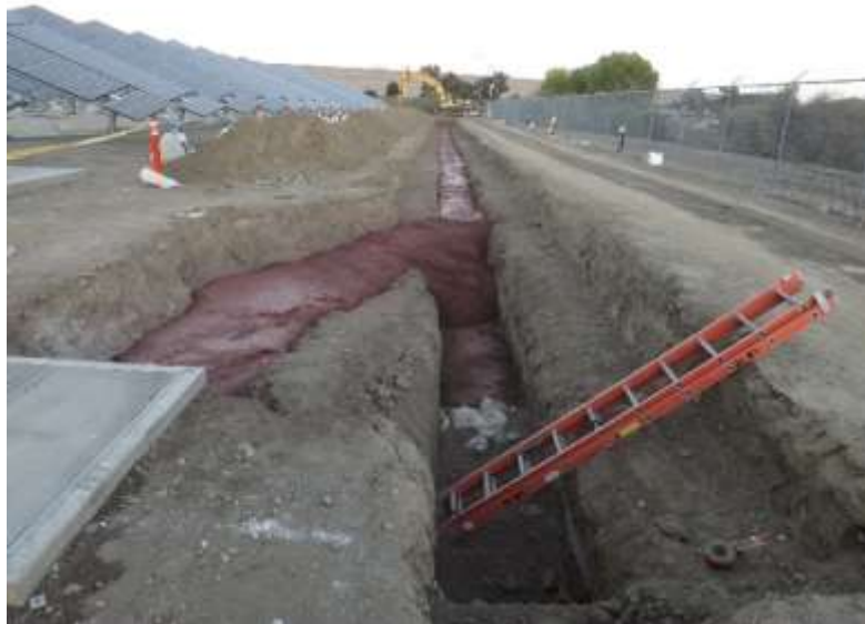
Electrical duct bank encased in red concrete at the Skinner plant
