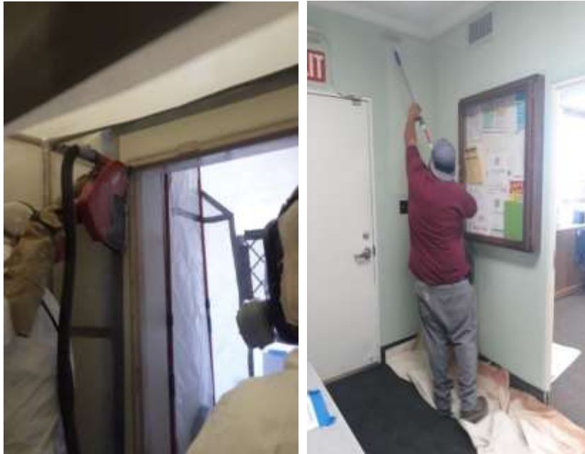
Staff enlarging the door frame for a new security door (left) and repainting the control room (right) at Eagle Mountain pumping plant
