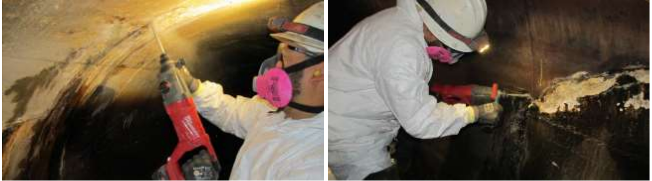
Staff preparing for hydrophilic injection repairs of the Rainbow Tunnel during shutdown of San Diego Pipelines 1 and 2
