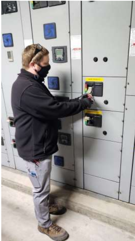
Staff performing lockout/blockout of a pump for maintenance (left) and staff performing a pump oil change at the Weymouth plant
