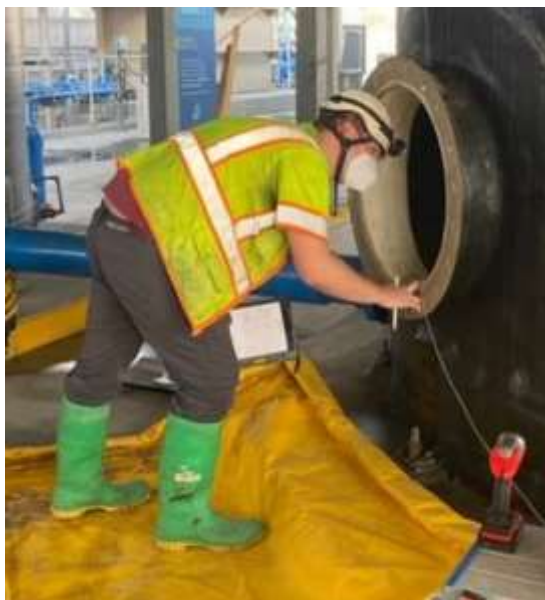
Staff inspecting the reverse osmosis feed tank at the demonstration facility
