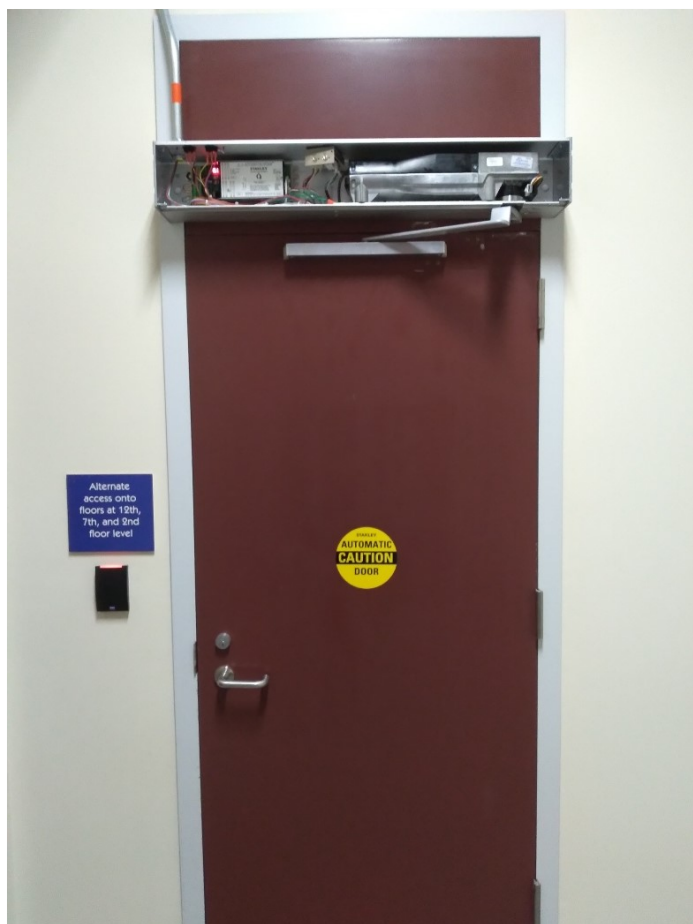
Installation of power door assist mechanisms
