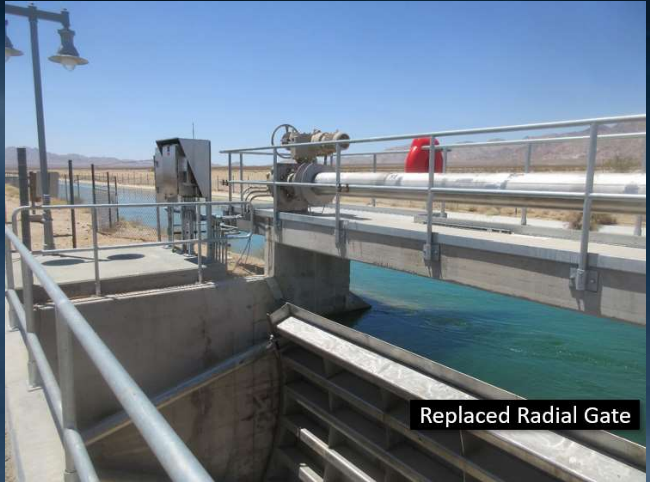
Completed radial gate in operation at Iron Mountain Wasteway
