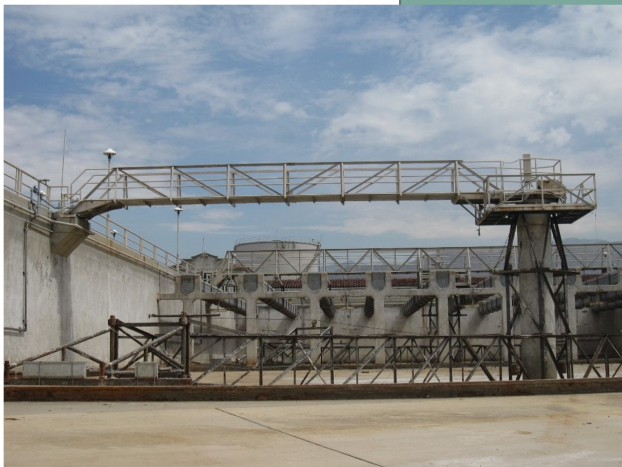
Example of major mechanical equipment to be replaced including rotating circular rake at Basin 5 of the Weymouth plant
