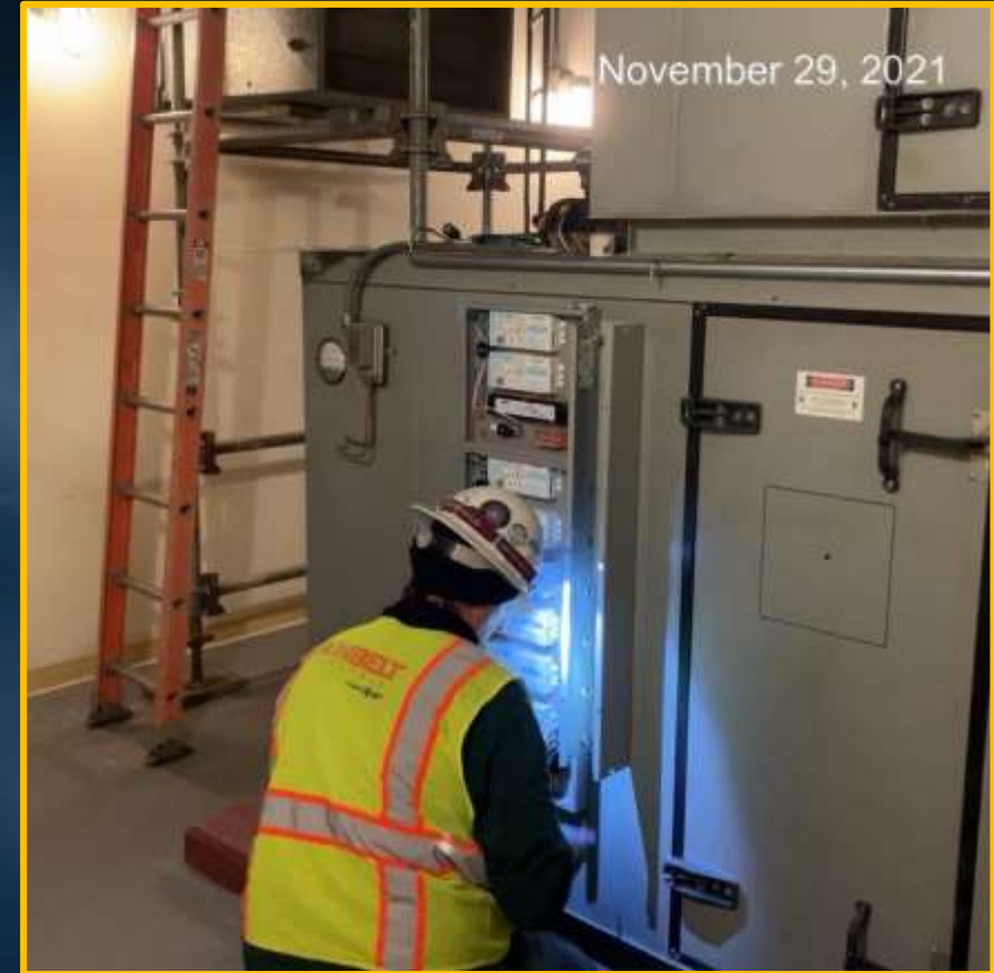
UVC controls in Mechanical Room, 1st Floor
