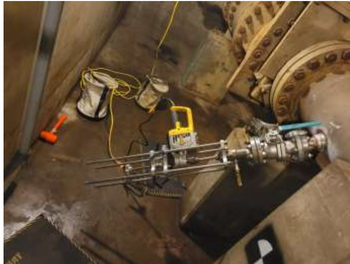
Completed hot tap with ball valve at the Sepulveda Feeder-West Basin Feeder interconnection
