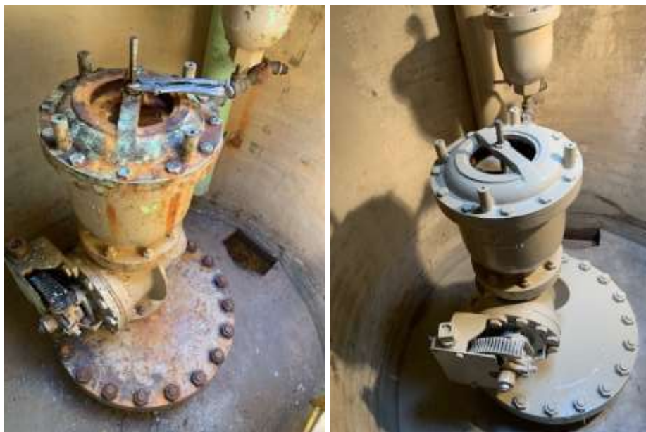
Rialto Feeder air release vacuum valve assembly before (left) and after (right) coating repair work
