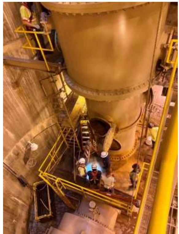
Staff being lowered into the structure (left) and inspecting (right) the secondary inlet sleeve valve at DVL
