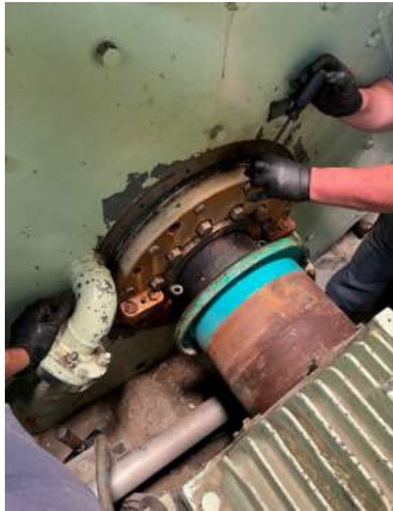
Staff disassembling turbine shaft seal at Temescal HEP
