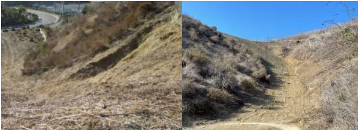
Erosion along the west edge (left) and completed slope repair (right) at the Diemer plant
