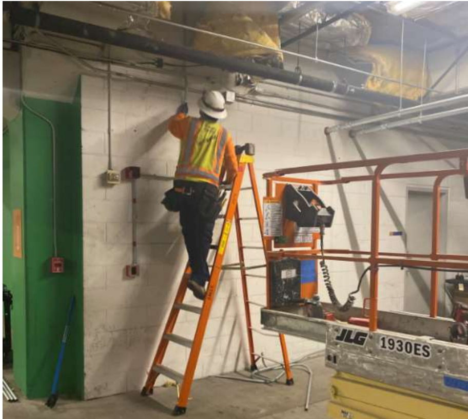
Headquarters Building Improvements —Installation of electrical conduit for Fire Alarm and Smoke Control Improvements in parking level P1.
