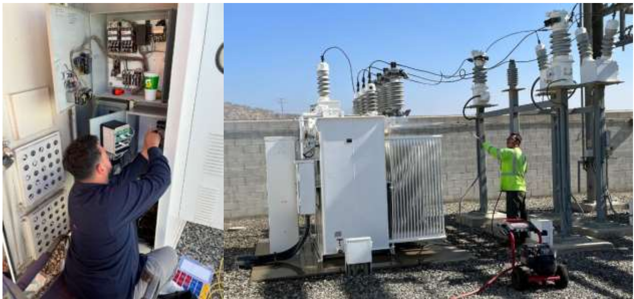
Staff installing new capacitor bank protection relays (left), and performing switchyard maintenance cleaning (right) at Temescal HEP
