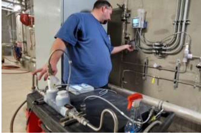
Control technician adding the instrument output loop modification at the Weymouth plant
