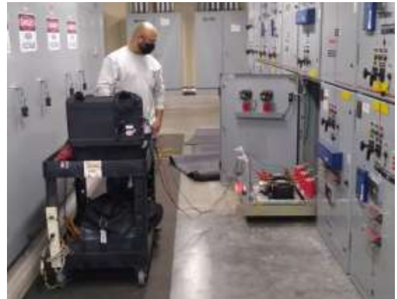
Staff performing high-voltage testing on vacuum-style circuit breakers (left) and electrical testing on instrument transformers (right) at the Weymouth plant
