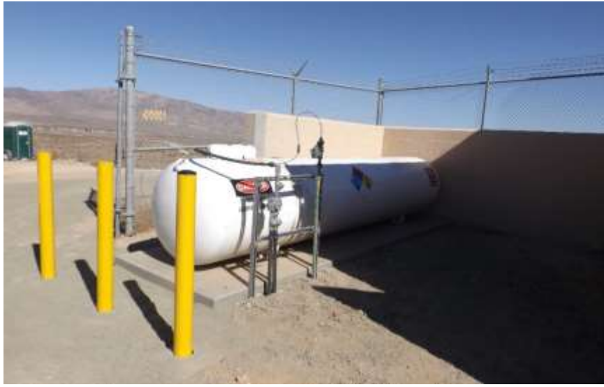
Installation of new 1,150 gallon propane tank at the Cactus City communication site
