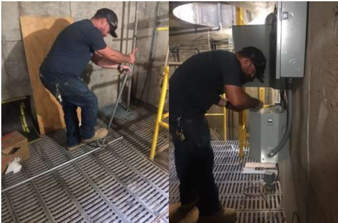
Staff bending conduit (left) and making low-voltage connections (right) at the transformer at the Palos Verdes Feeder-West Coast Feeder interconnection
