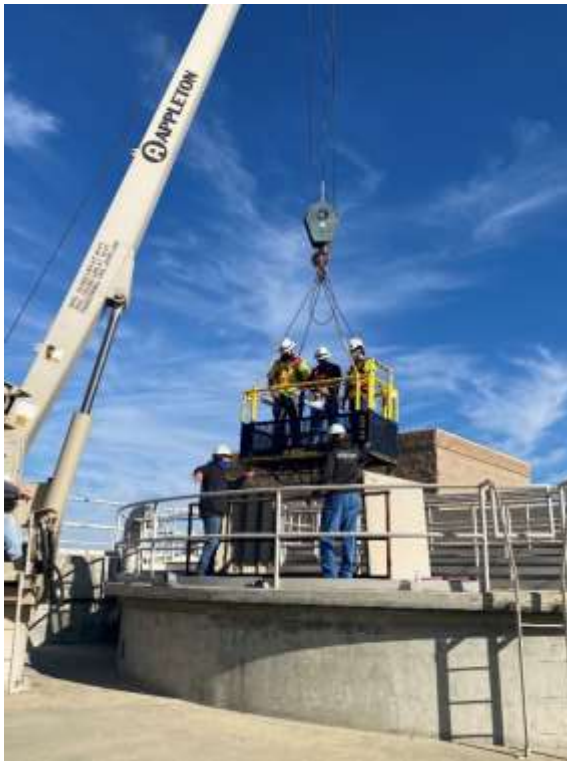
Staff being lowered into the structure (left) and inspecting (right) the secondary inlet sleeve valve at DVL
