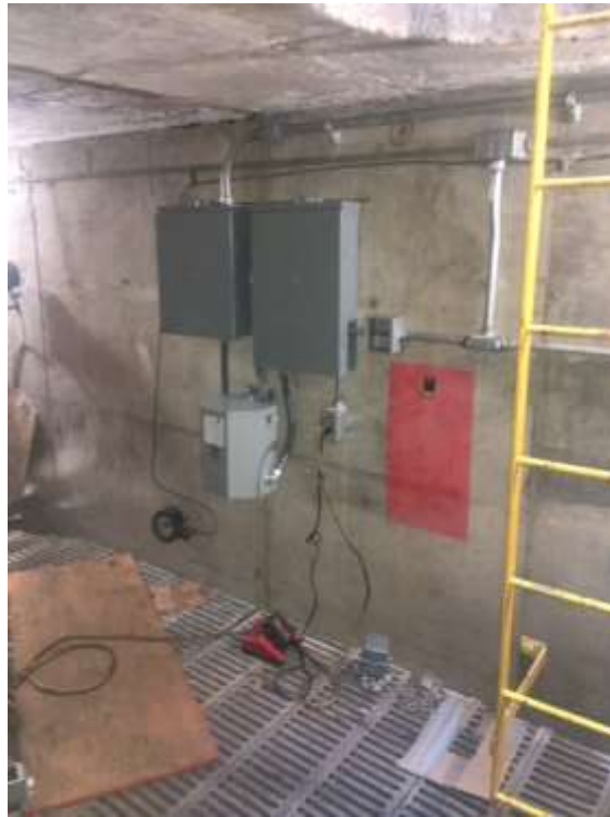
New electrical panels and transformer at the interconnection structure
