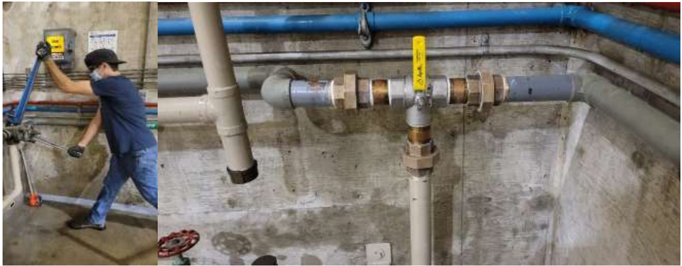
Staff removing damaged plug valve (left) and new ball valve installed (right) at Coastal Junction PCS
