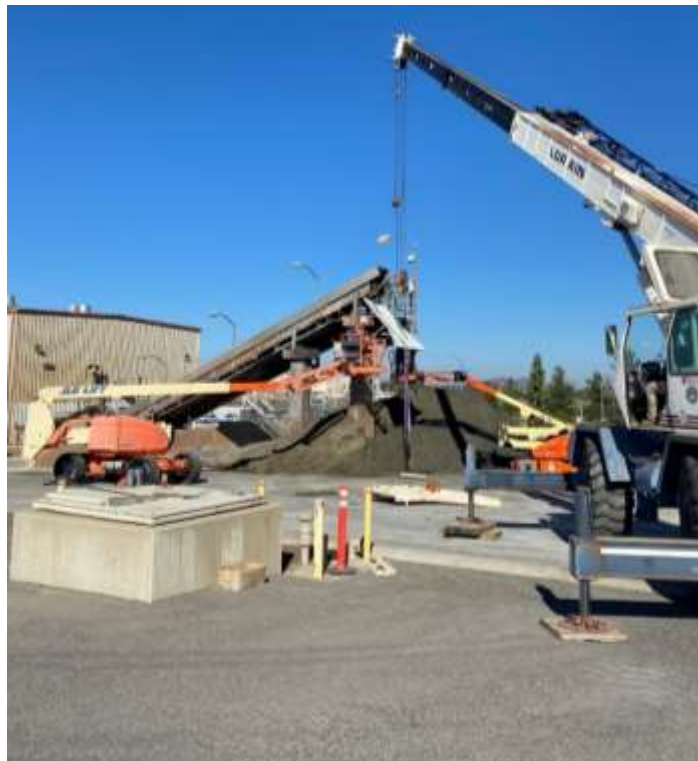
Conveyor chute being installed at the Skinner plant
