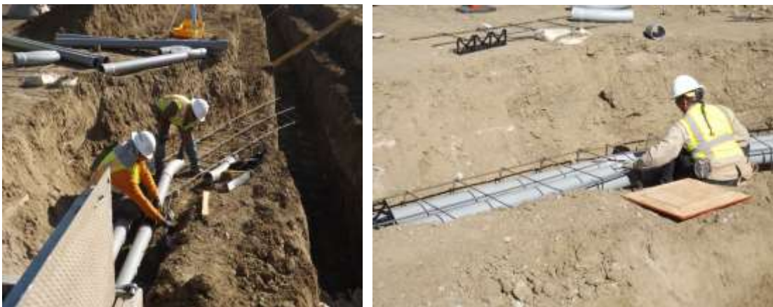
Staff installing conduit (left) and tying steel reinforcement cage (right) to support a battery energy storage system project at the Skinner plant
