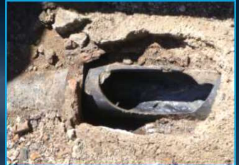
Damaged Wastewater Line
