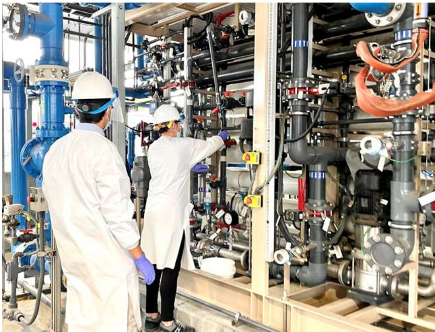
Samples of reverse osmosis permeate being collected at the demonstration facility
