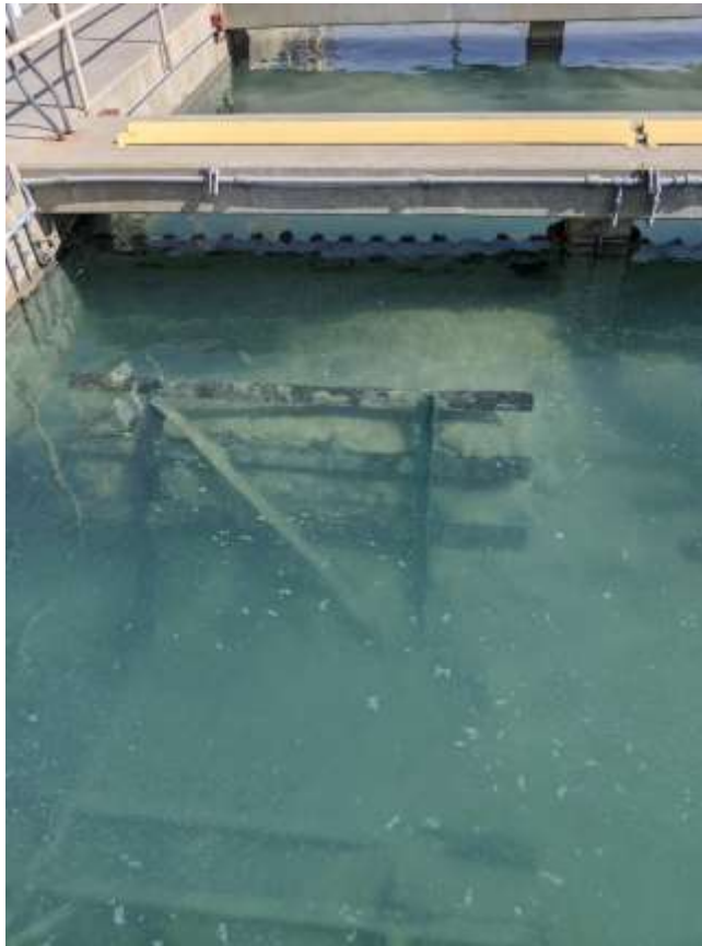
Filter media buildup on wastewater reclamation plant flocculator at the Diemer plant
