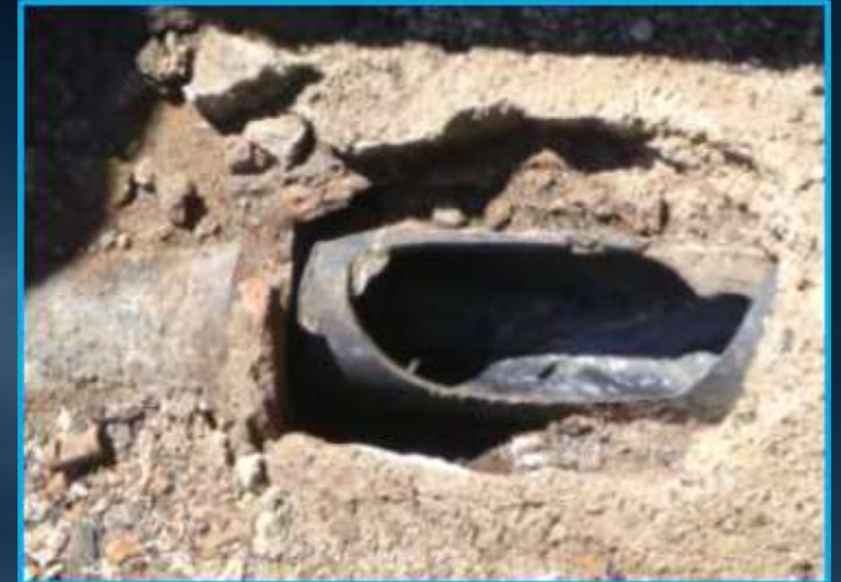
Damaged Wastewater Line
