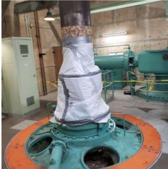
Pump headcover prepared for coating repairs at Eagle Mountain pumping plant
