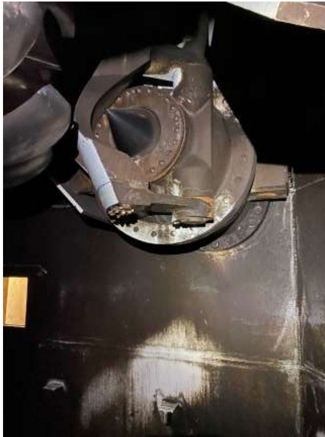
Etiwanda HEP needle valve inspection
