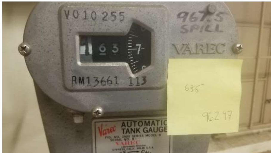
Fifty-year-old water level monitoring equipment before replacement at the OC-11 service connection
