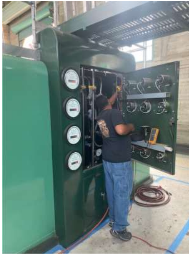
Desert staff calibrating a pump unit's oil instrumentation at Intake pumping plant
