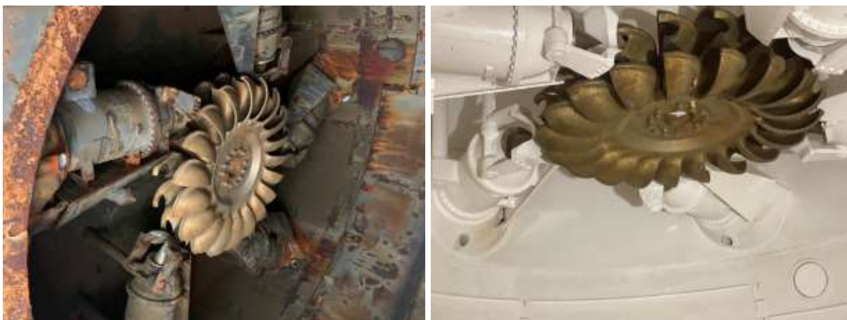
Tailrace before (left) and after (right) coating work at Sepulveda Canyon HEP
