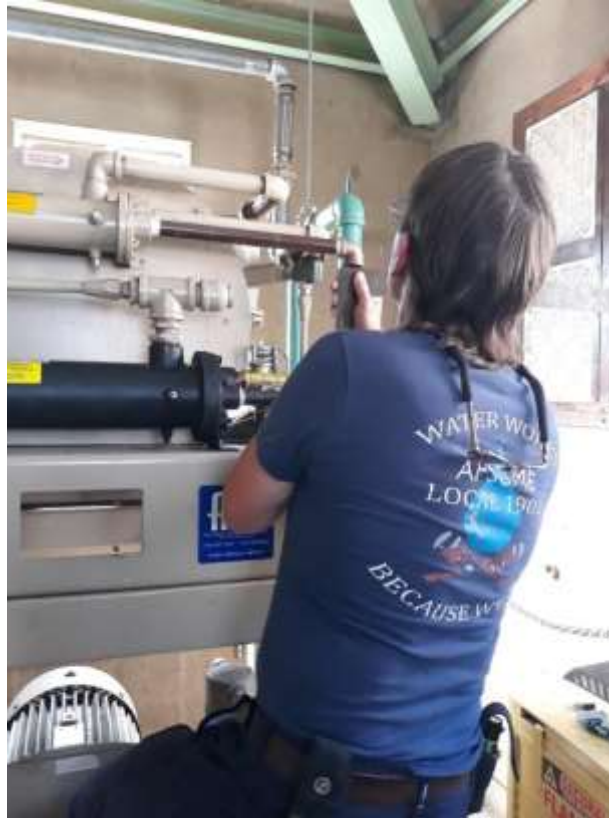
Staff replacing corroded air compressor piping at Eagle Mountain pumping plant
