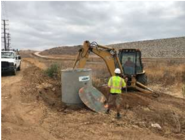
Staff installing accessway ring (left) and installed accessway and gravel (right) at Lake Mathews
