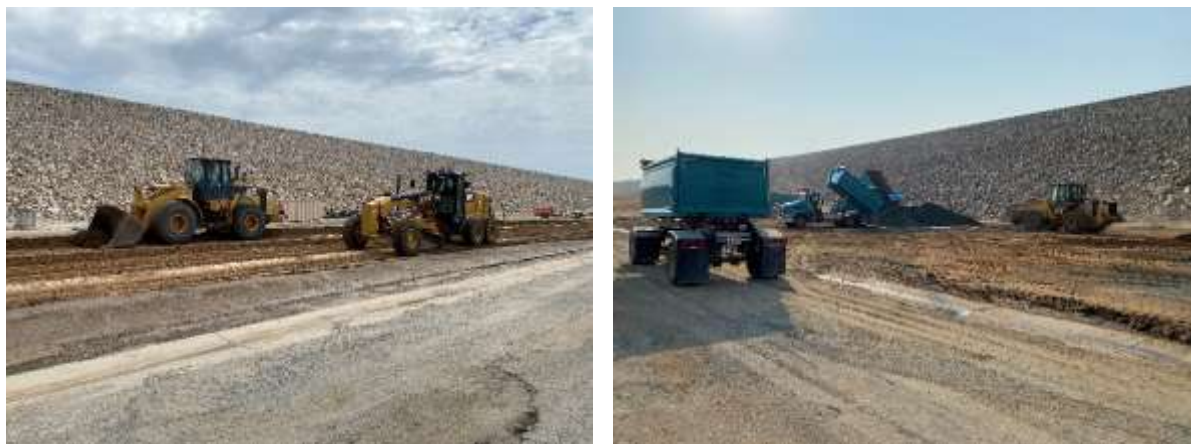
Motorgrader prepping subgrade (left) and receiving aggregate base material (right) at Lake Mathews
