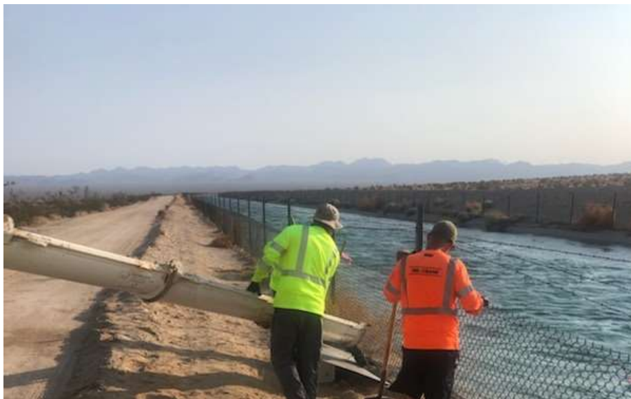
CRA staff filling voids with concrete slurry near the canal liner
