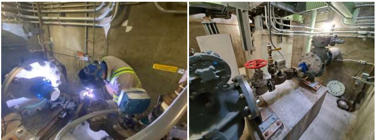
Staff welding bypass pipe (left) and completed installation of bypass line (right) at the De Soto Valve Structure
