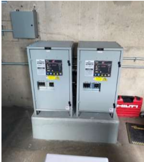
New station battery bank charger at Eagle Mountain pumping plant
