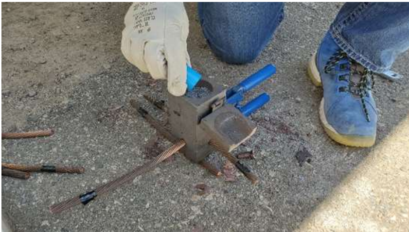
Electrical apprentice applying ignition powder to the graphite mold
