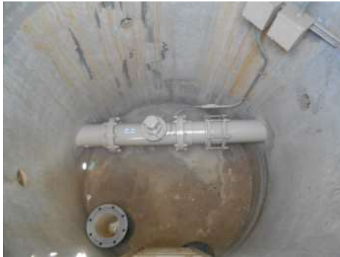
Perris Bypass Pipeline valve structure after coating
