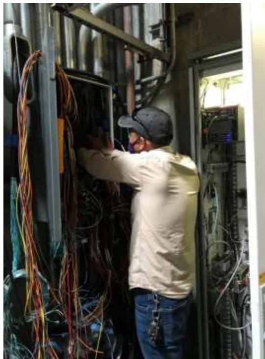
Staff relocating the RTU at the Jensen plant
