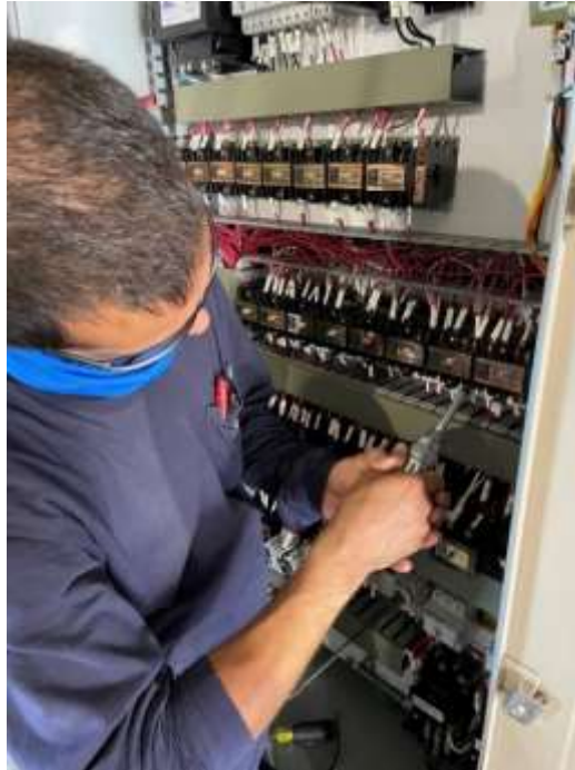
Staff ensures terminals are properly torqued at the Lake Mathews HEP
