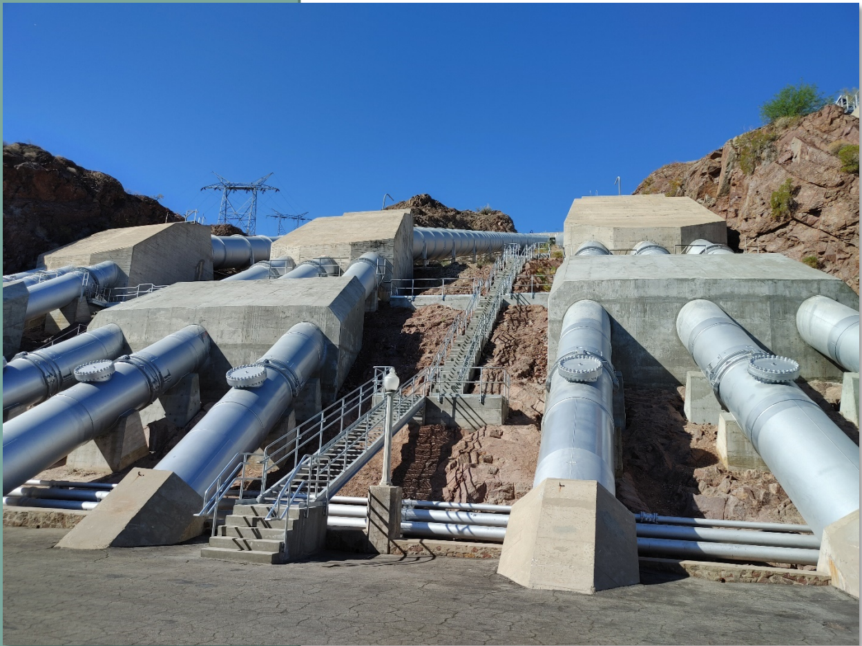
Completed concrete pipe supports, stairs, and handrailing at Intake Pumping Plant
