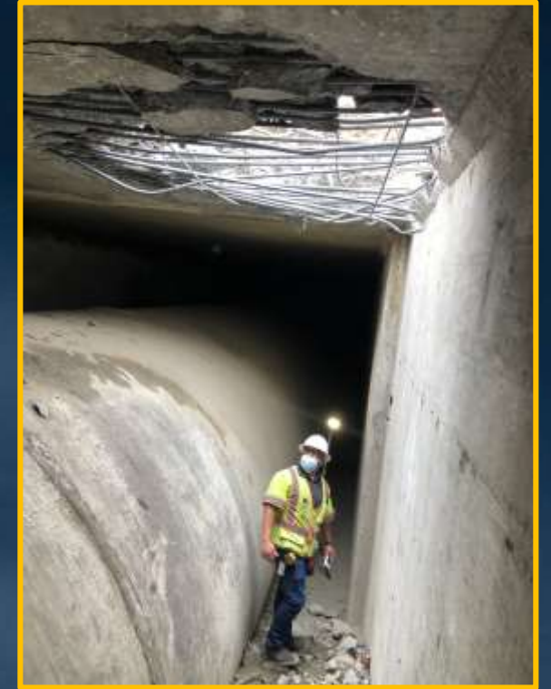
Upper Feeder beneath damaged protection structure
