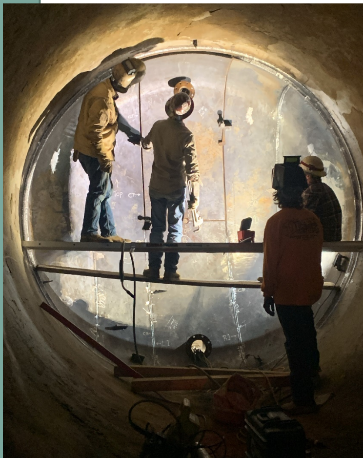
Welding of 133-inch bulkhead on Lakeview Pipeline
