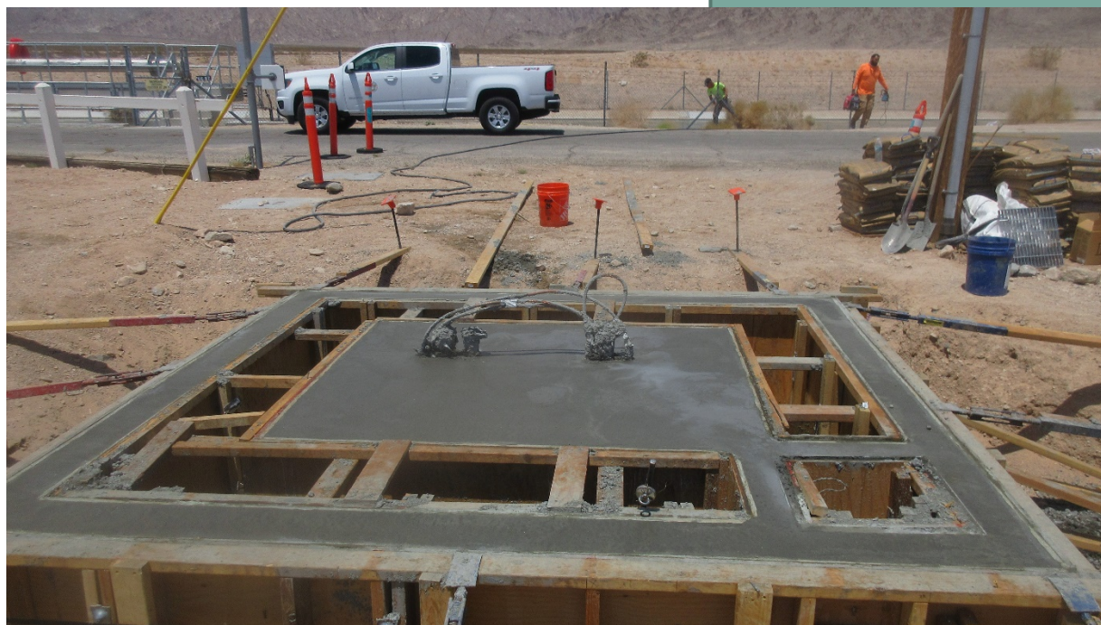
Construction of concrete transformer pad for radial gate at Iron Mountain Wasteway
