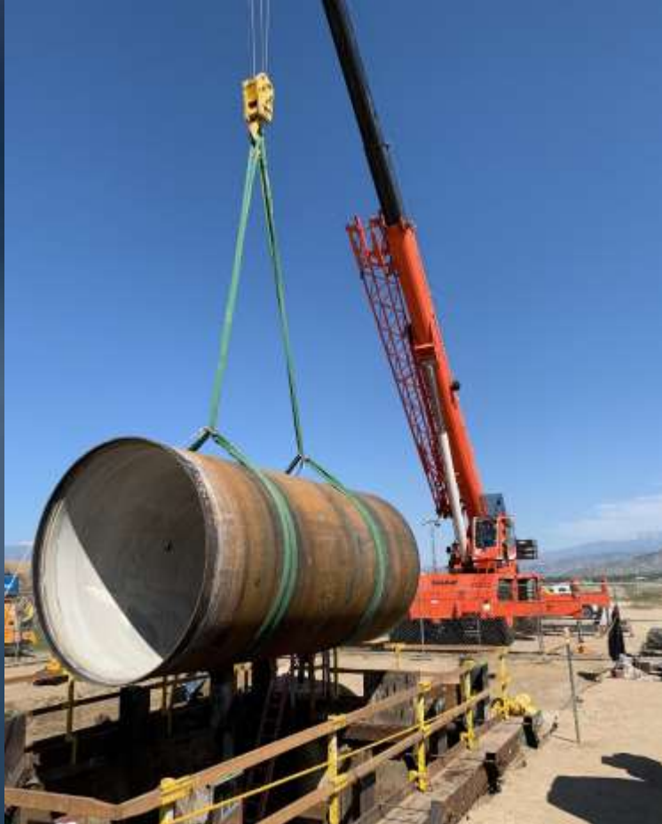
Lowering of steel liner for initial fit-up
