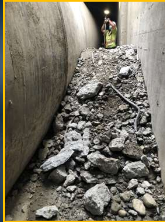
Upper Feeder beneath damaged protection structure
