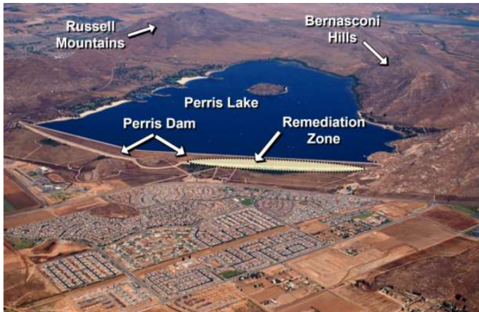
Seismic Remediation of Perris Dam Embankment – photo credit: DWR
