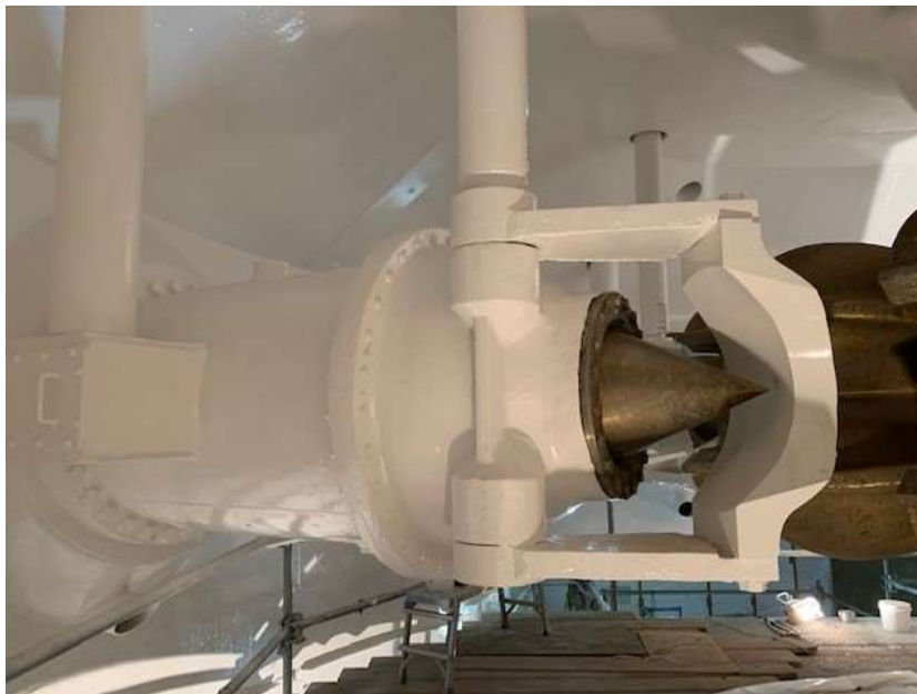
Needle valve after coating at the Sepulveda Canyon HEP
