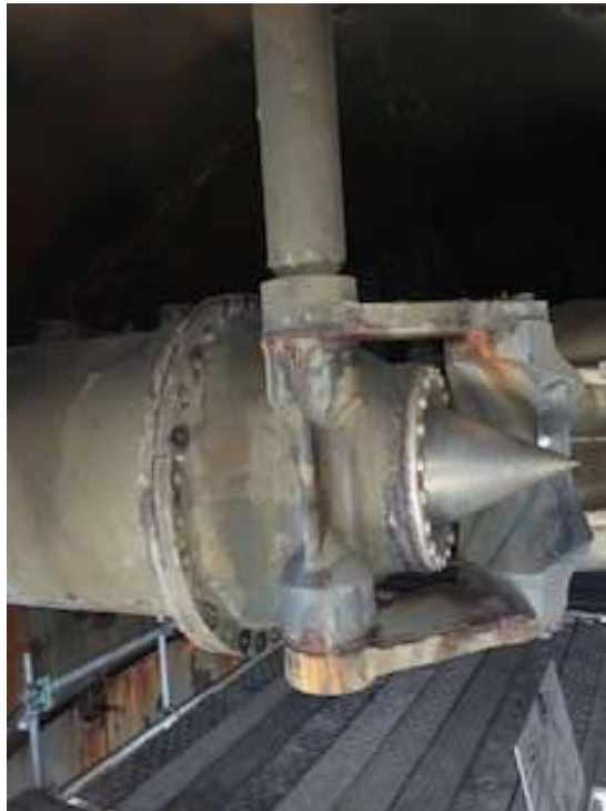
Needle valve before coating at the Sepulveda Canyon HEP
