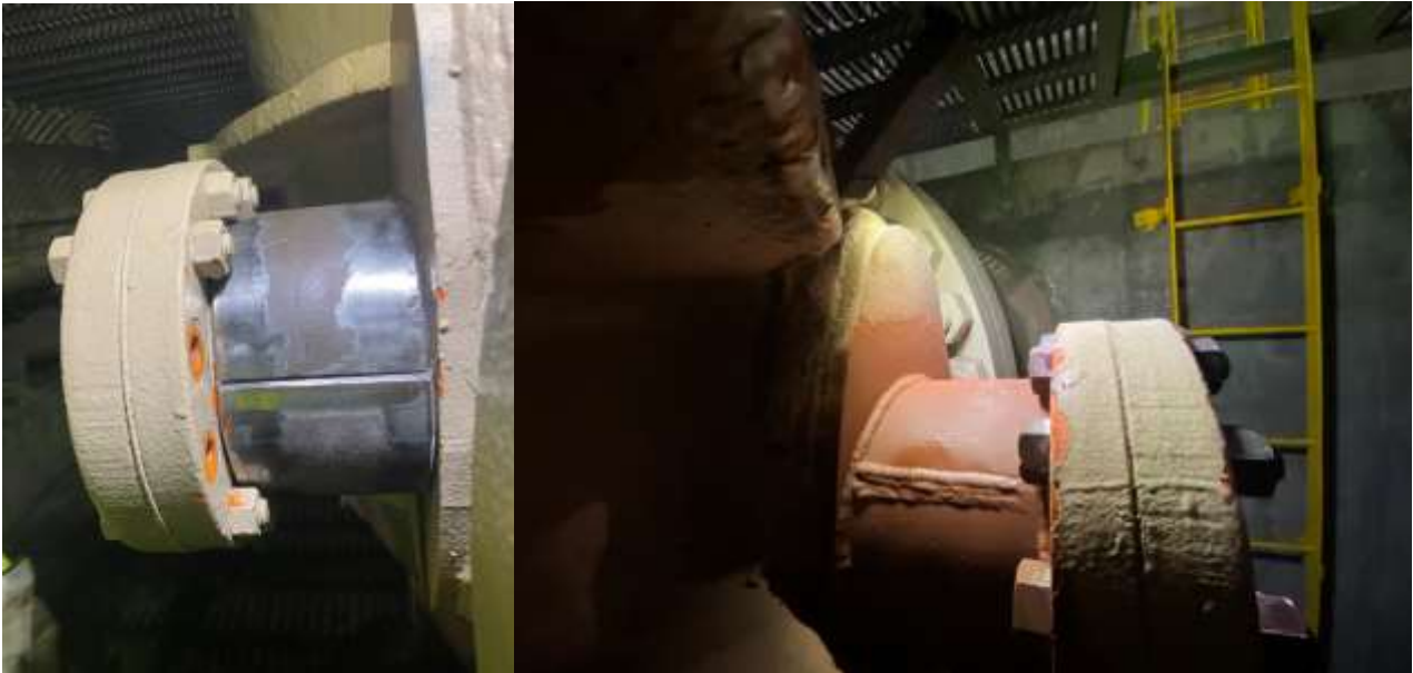
Welded patch plate at Santiago Creek PCS
