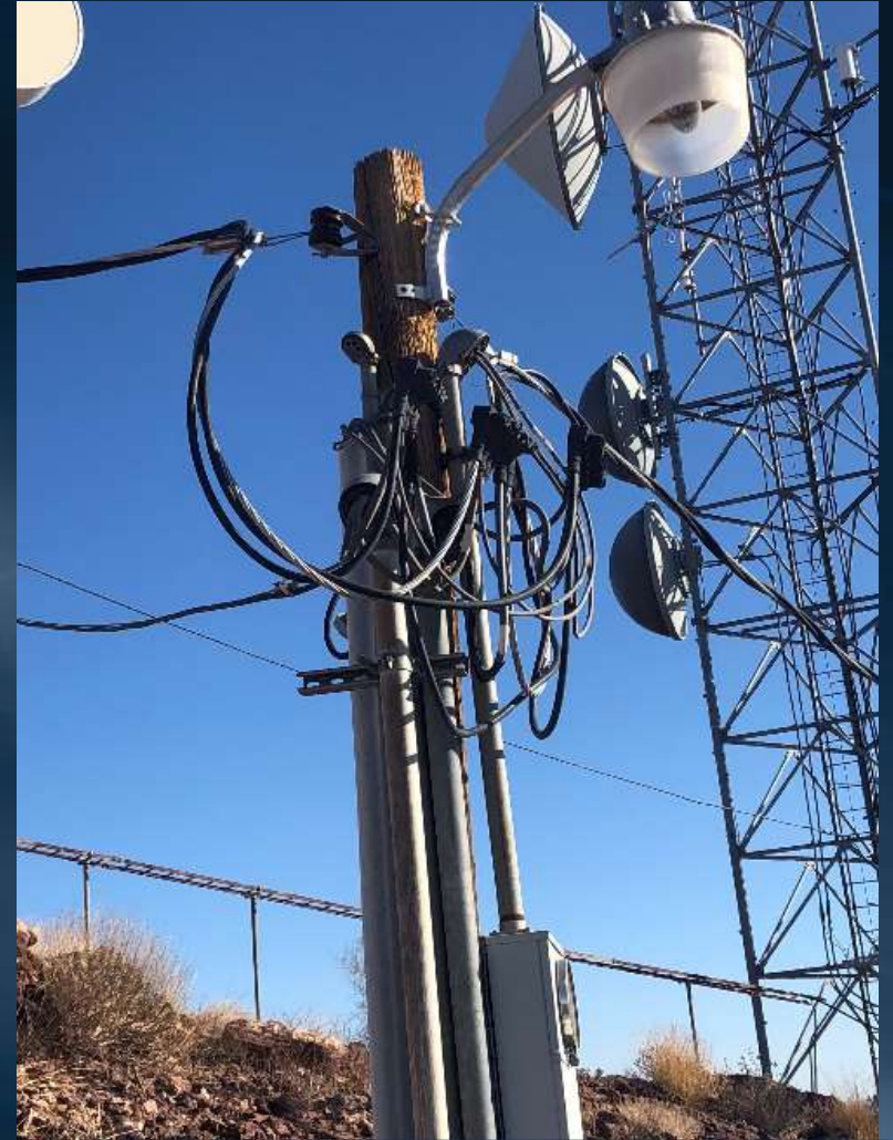
Overloaded Power Pole
