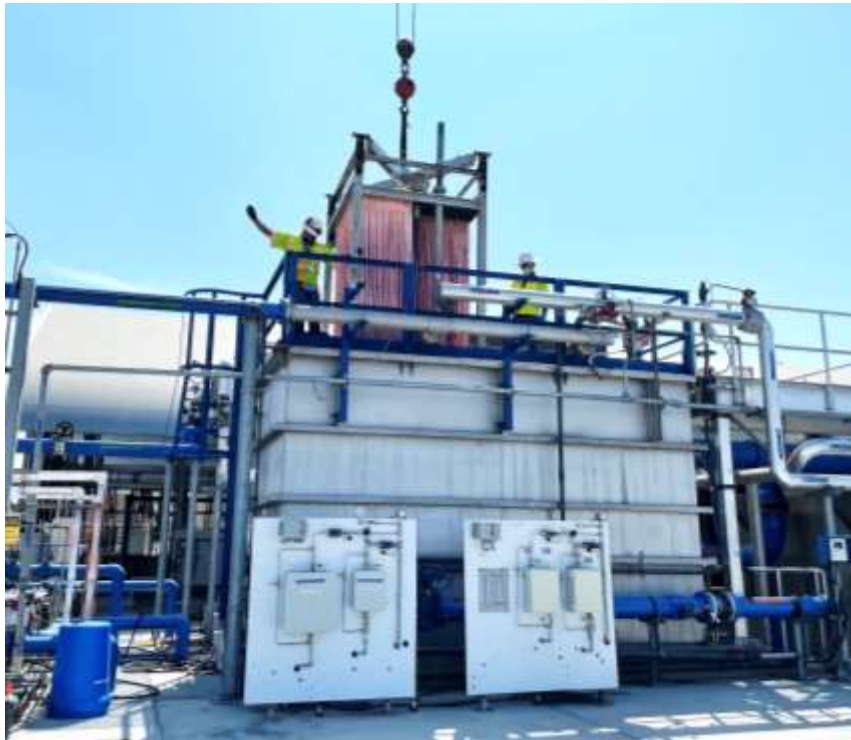
Staff signal the crane operator for MBR cassette removal from the tank at the demonstration facility
