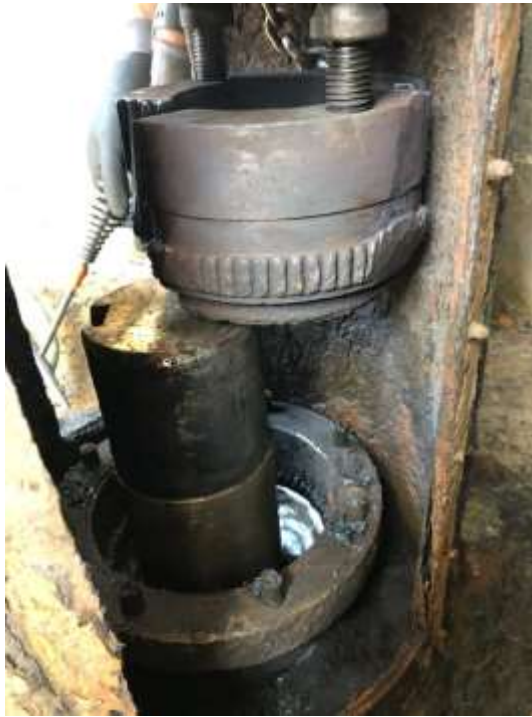
Inoperable valve coupling (left) and staff removing the valve coupling (right) at the Weymouth plant
