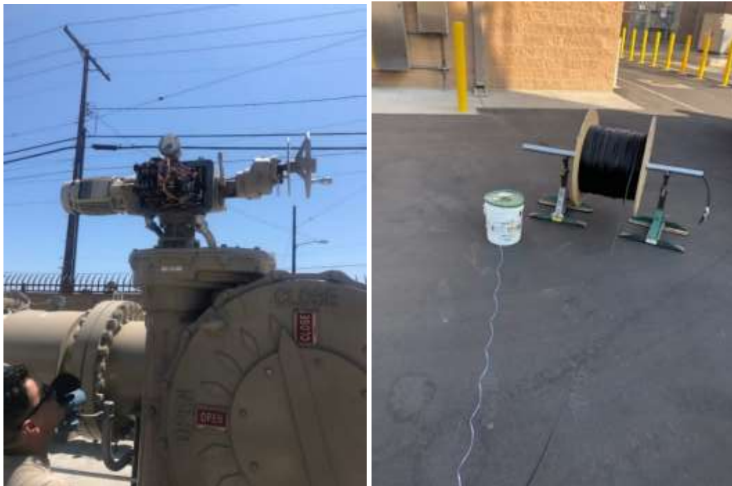
Control valve (left) and new potentiometer cable (right) at the Greg Avenue pump station
