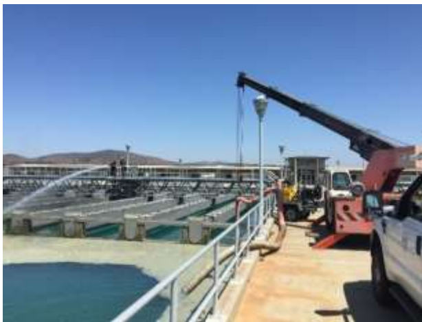
Staff removing material layer from a sedimentation basin (left) and dumping coal from the reclamation plant (right) at the Diemer plant
