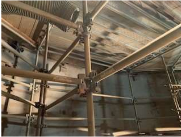
Scaffolding and ventilation containment setup for sandblasting and repairs in the tailrace chamber at the Sepulveda Canyon HEP
