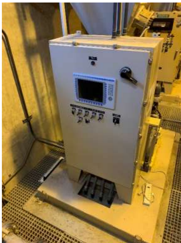
New HMI display panel installed for the dry polymer mixer at the Skinner plant
