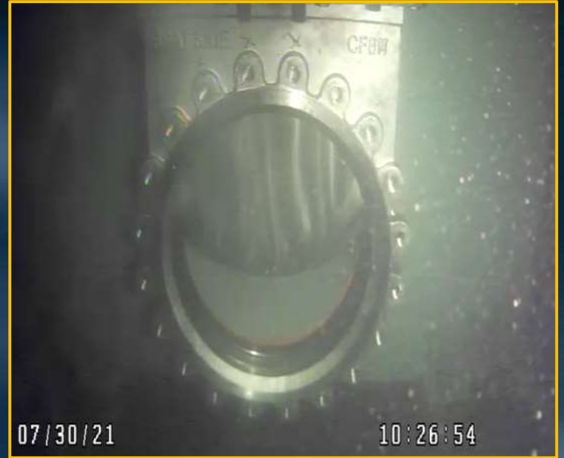
Knife gate valve in place – water side
