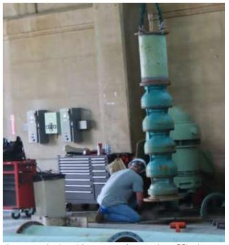
Staff removing a vertical turbine pump for repair at Hinds pumping plant
