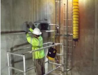
Staff threading conduit (left) and installing new conduit inside the structure (right) on San Diego Pipeline No.
