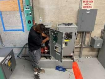
Staff placing new battery charger into position (left) and wiring new battery charger (right) at Hinds pumping plant
