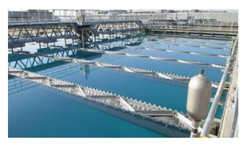
**West Basin and Filter Building Rehabilitation**—Newly installed walkway bridges and launders at the west basins (looking south-east over Basin 8)
