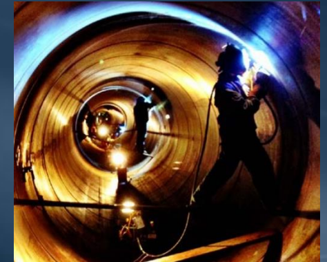
Welded Steel Pipe Joints
