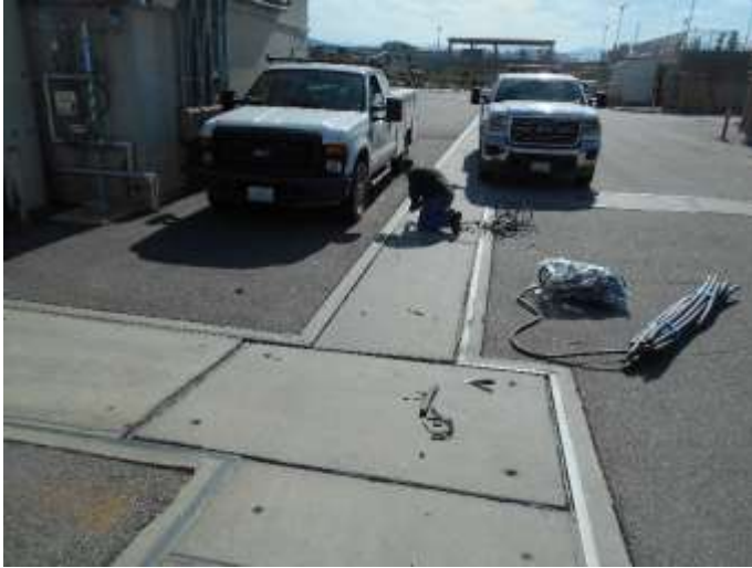
Staff during expansion joint replacement (left) and after replacement (right) around chemical process piping trench at Skinner plant
