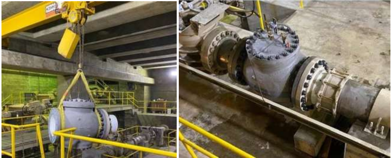
Refurbished globe valve being lowered and reinstalled at the Ramona PCS on the Middle Feeder
