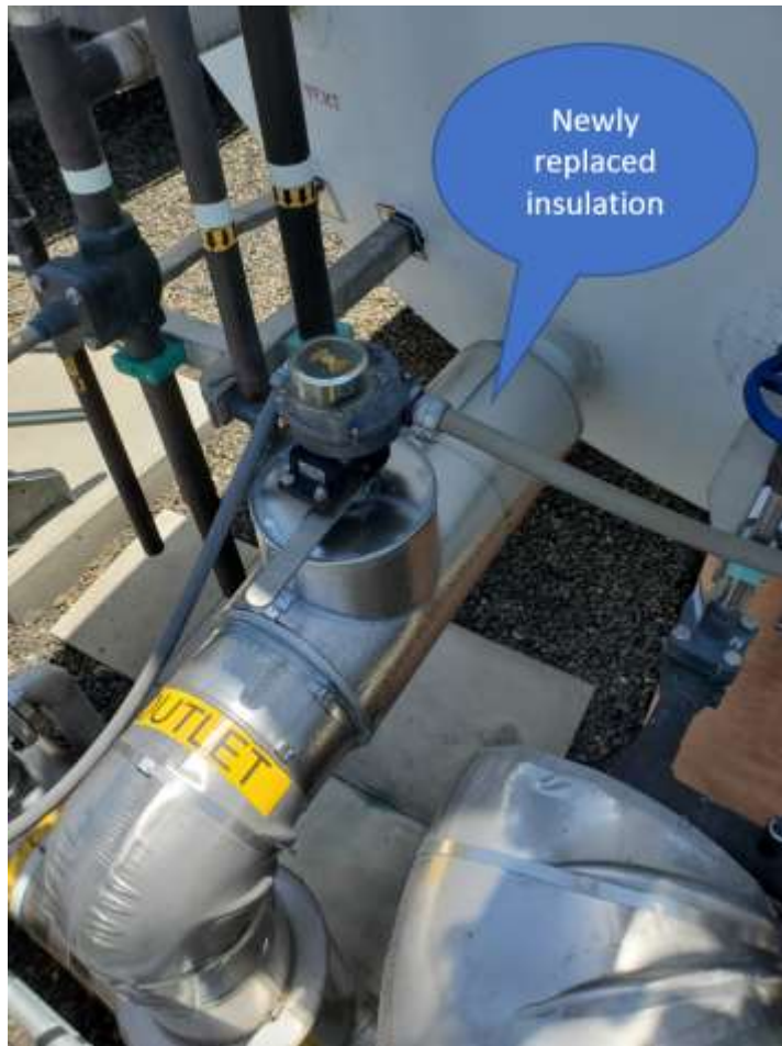
LOX feed line with newly replaced insulation at the Skinner plant
