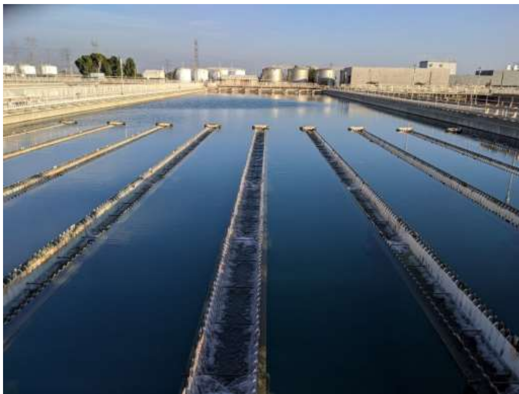
Sedimentation basin at the Jensen plant
