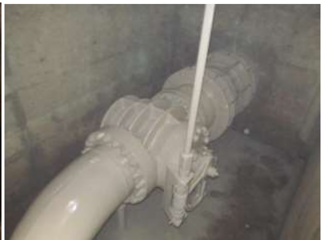
Turnout valve and meter structure before (left) and after coating (right) of OC-48 service connection
