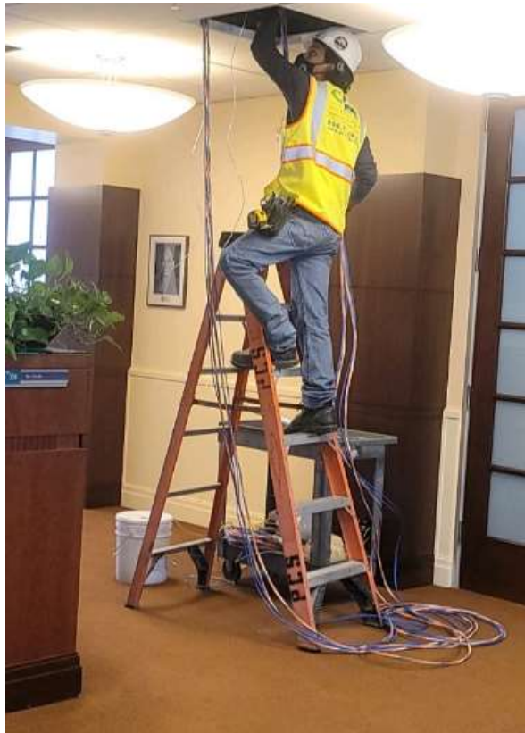
Headquarters Building Improvements—Contractor routing low voltage cables
