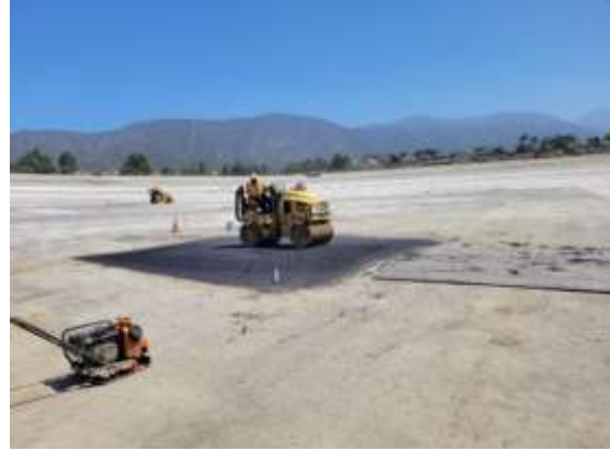
Staff completing the excavation and paving of repair patches inside Live Oak Reservoir
