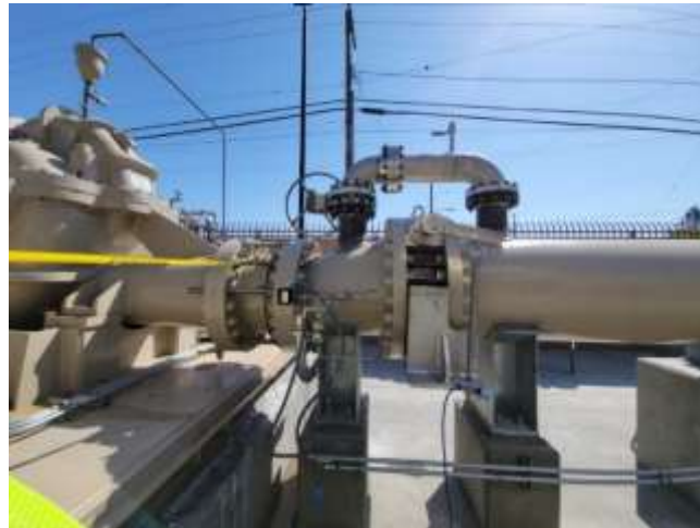
Installed bypass piping for Greg Avenue pump station
