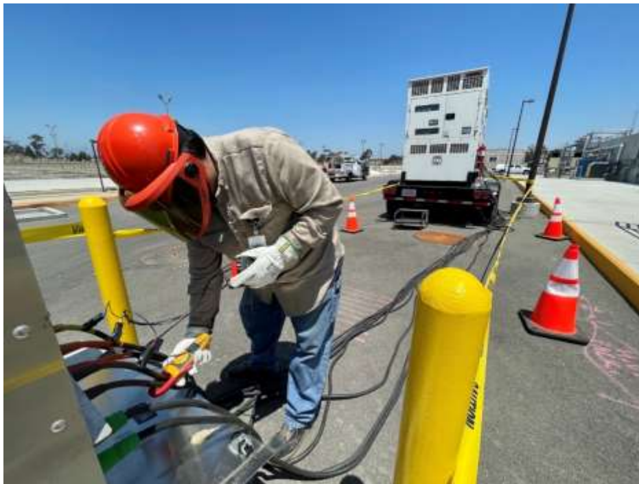
Staff confirm power supply through the portable generator during a scheduled electrical outage at the demonstration facility
