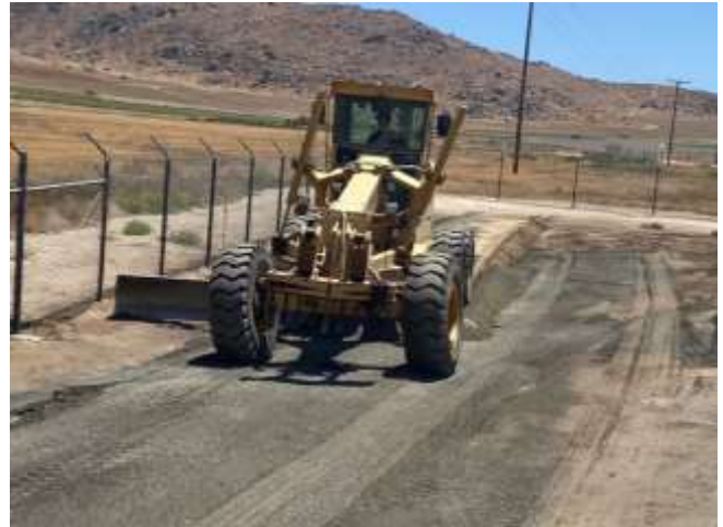
Staff repairing the slopes and perimeter fence line using a motor grader and dozer at Inland Feeder Pressure Control Structure PC-1
