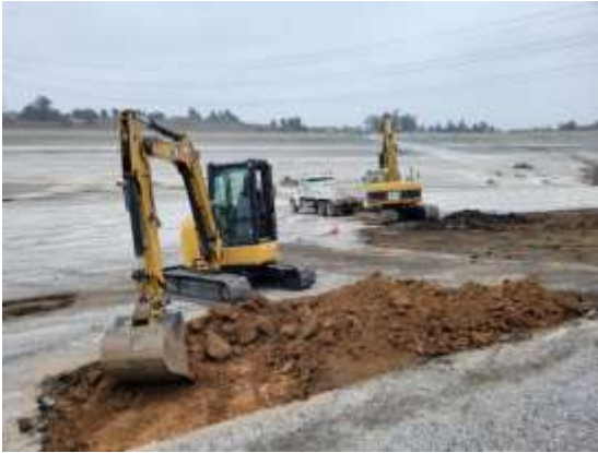
Staff completing the excavation and paving of repair patches inside Live Oak Reservoir
