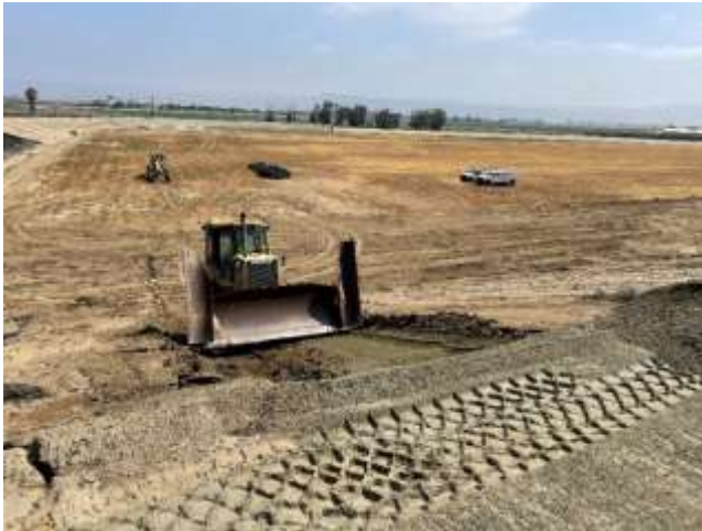
Staff repairing the slopes and perimeter fence line using a motor grader and dozer at Inland Feeder Pressure Control Structure PC-1
