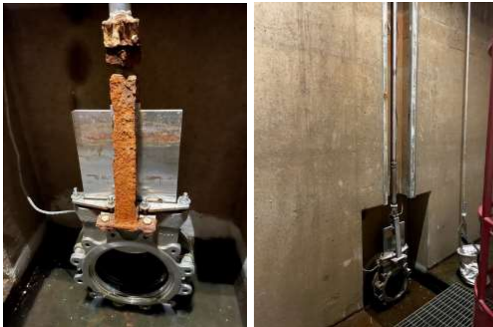
Sump drain valve extensions and operators before replacement (left) and after replacement (right) at the Wadsworth pumping plant
