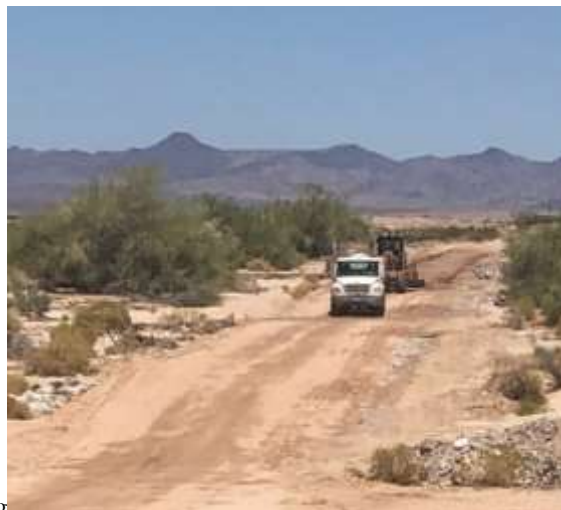
Staff repairing a CRA access road using a water truck to minimize dust
