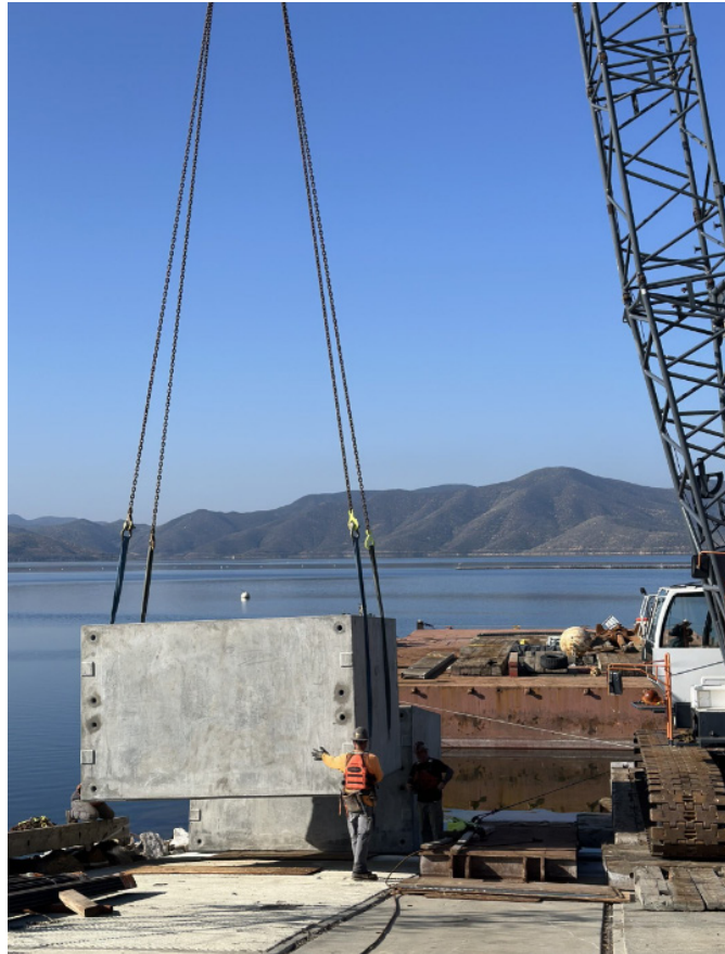
Diamond Valley Lake Wave Attenuator Replacement New Floating Wave Attenuator Module Delivery
