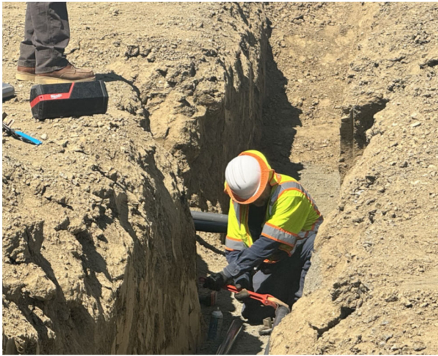
Staff installing electrical conduits for the heli-hydrant at the Diemer plant.
