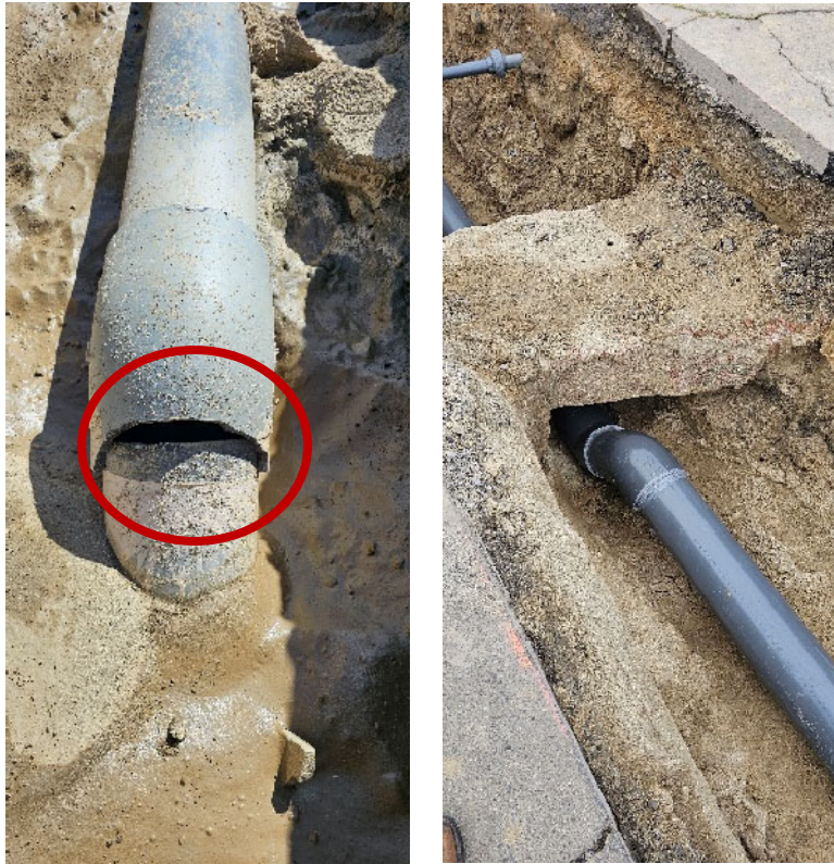
Broken 8-inch, 45-degree pipe joint (left) and repaired pipe and joint (right) in the Skinner area
