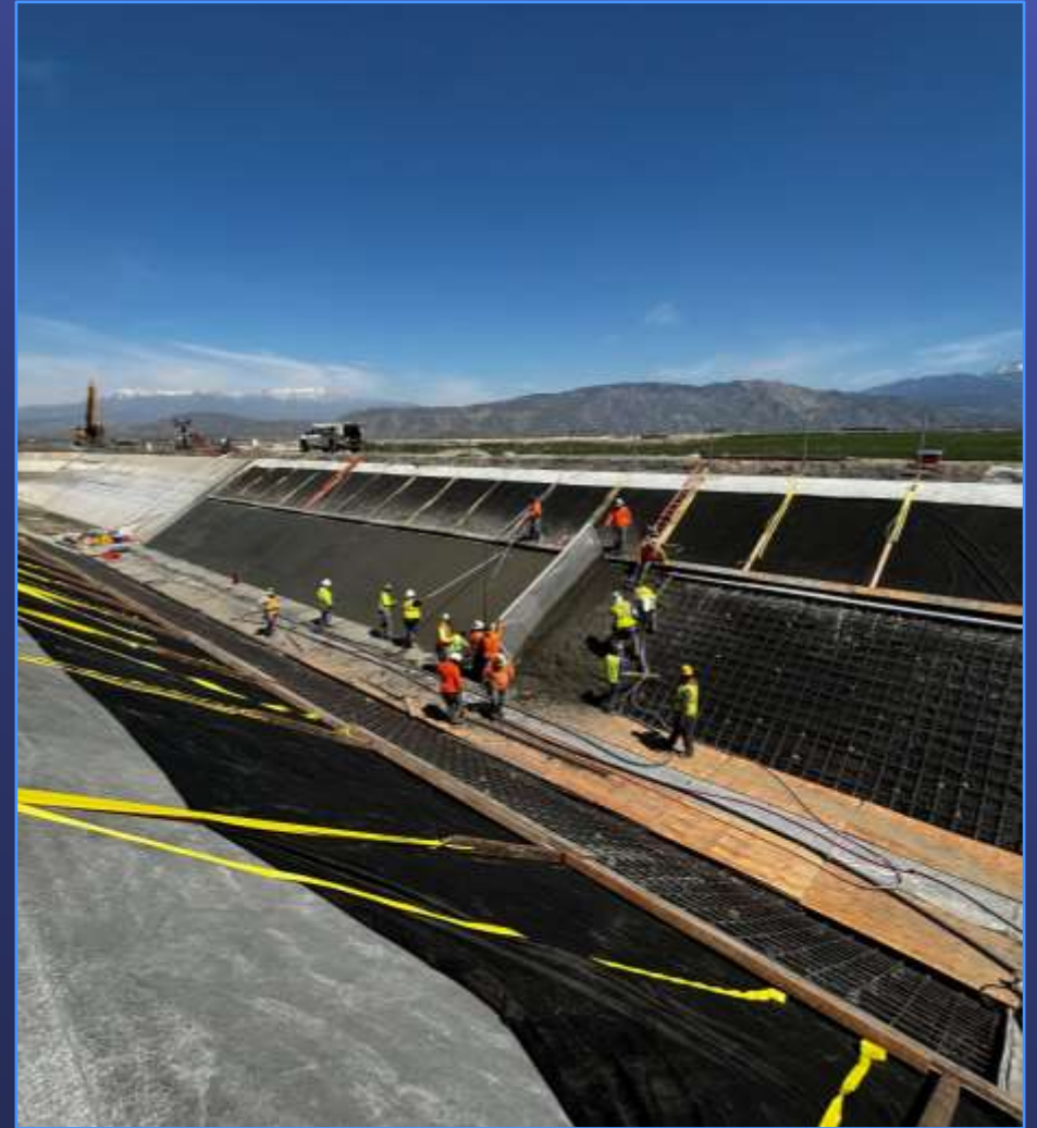
Contractor Placing Concrete for Canal Panels
