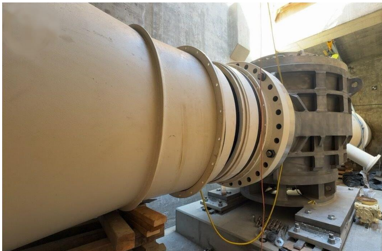
New 48-inch conical plug sectionalizing valve installation at valve vault 1859+80 in the City of Los Angeles
