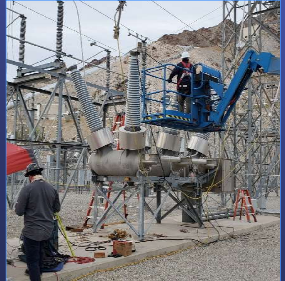
Staff Performing Electrical Maintenance on 230kV Circuit Breaker
