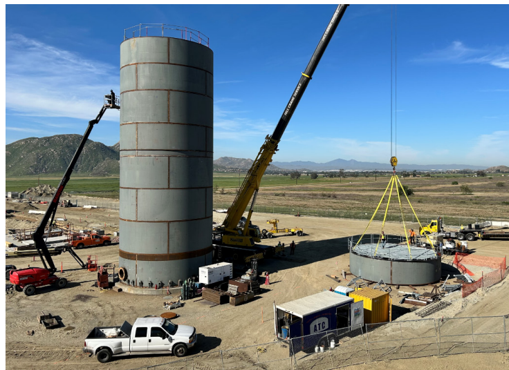
Inland Feeder-Badlands Tunnel Surge Protection – Top Ring for Surge Tank
