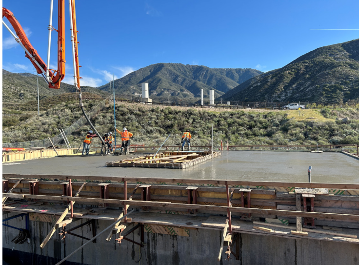
Inland Feeder Rialto Pipeline Intertie – Placing Valve Vault Concrete Deck
