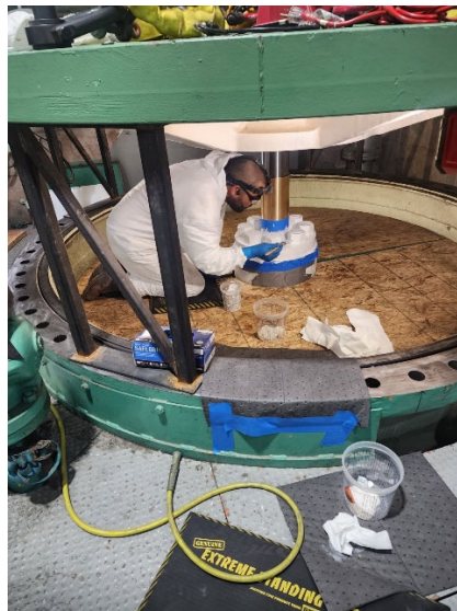
Discharge Valve coating applications at the Iron Mountain Pumping Plant
