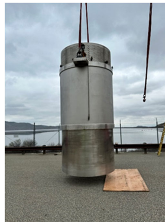
Assembly of DVL sleeve valve gate and inner sleeve
