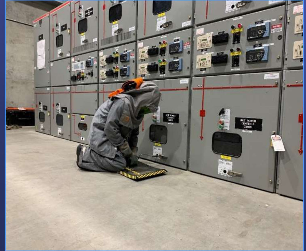
Staff Isolating Equipment for Maintenance at Skinner WTP
