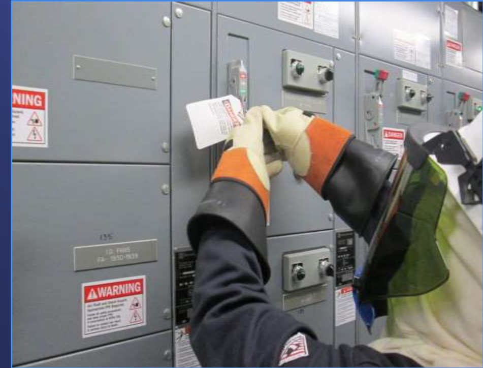
Labeling & Working with Live System
