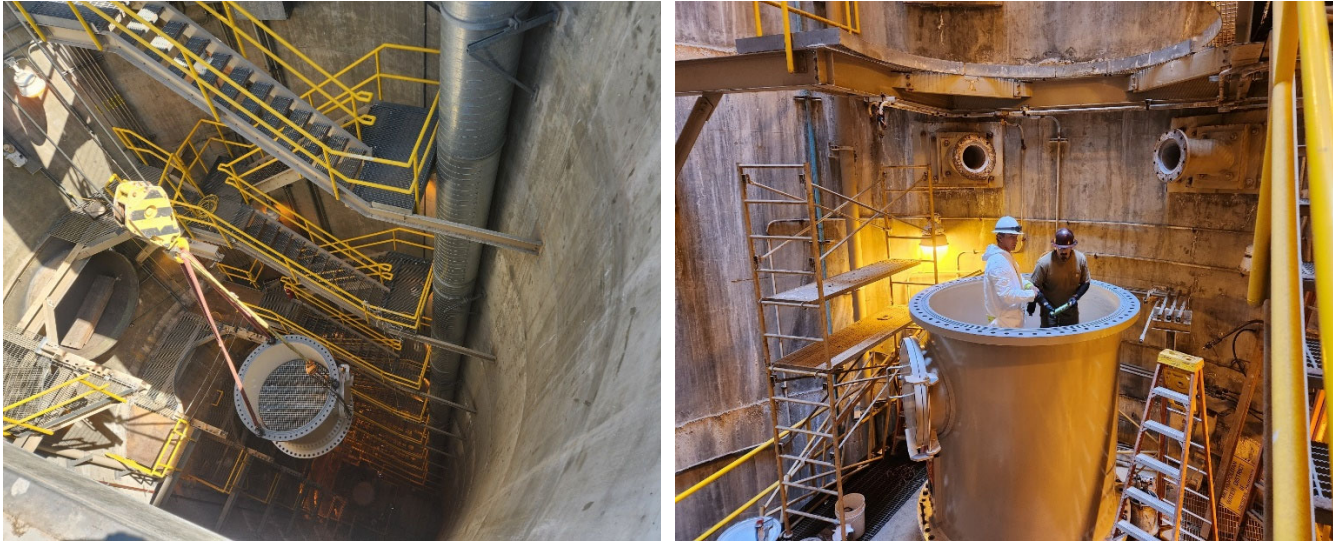
View of the 170-foot-deep shaft as a valve body piece is lowered into position (left) and staff preparing the flange face connection (right)
