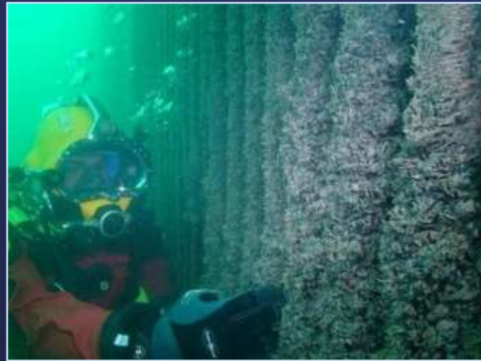
Colonized Intake Trash Rack
