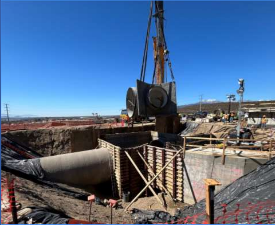
Installation of New Tee at Tie-In of Bypass Pipeline and Inland Feeder Pipeline
