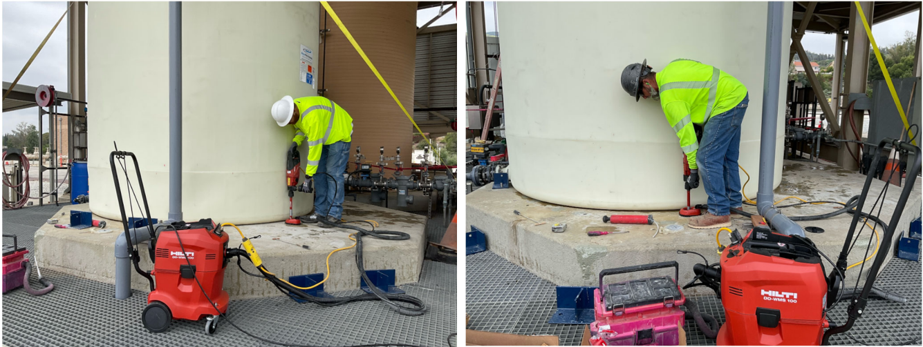
Staff core drilling chemical tank base for tie-down brackets at the Jensen plant.
