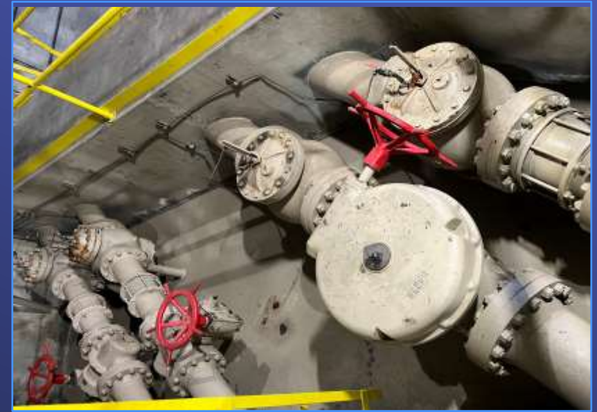
Aged Piping and Valve System
