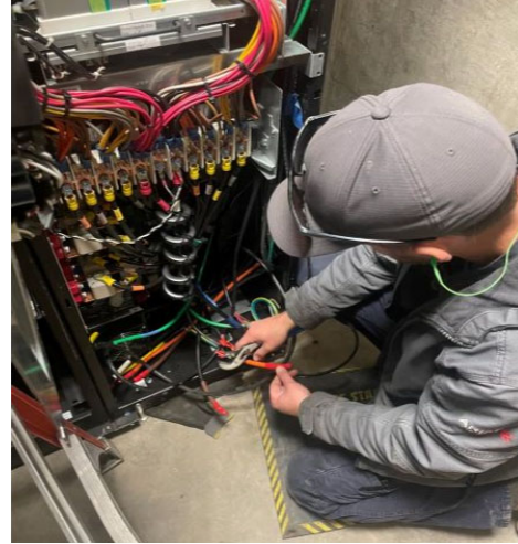
Staff moving new UPS unit into position (left) and making electrical connections (right) at San Dimas PCS.
