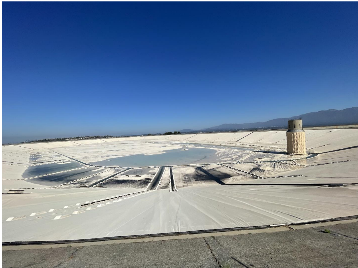
Reservoir floating cover overview at Garvey Reservoir
