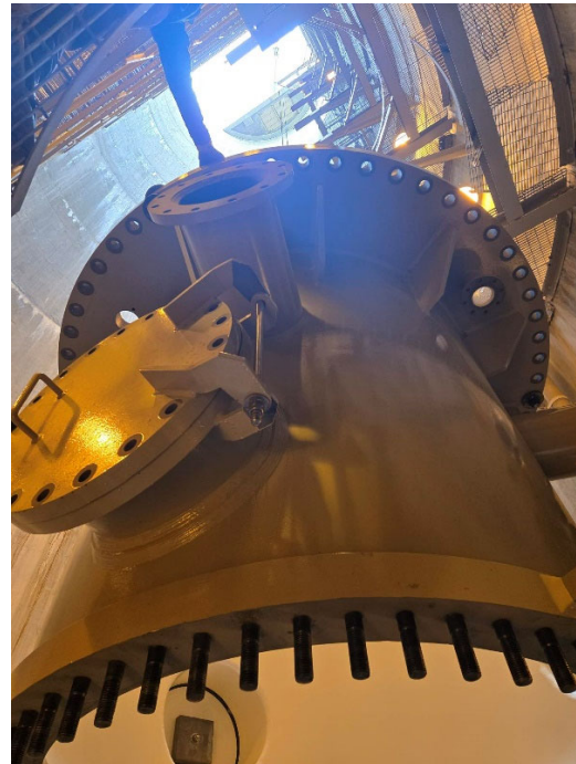
Staff lowering a 72-inch sleeve valve segment into the DVL Secondary Inlet shaft.
