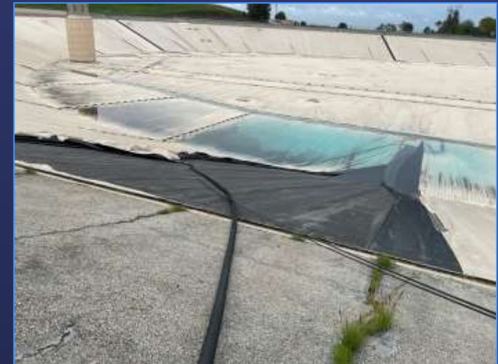
Cover Failure March 2025
