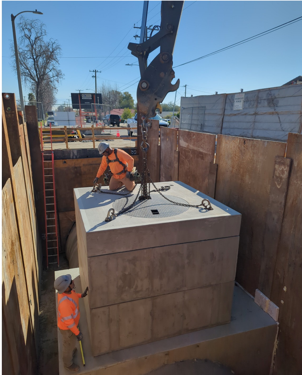
Rialto Pipeline Rehabilitation – Installation of Access Structure
