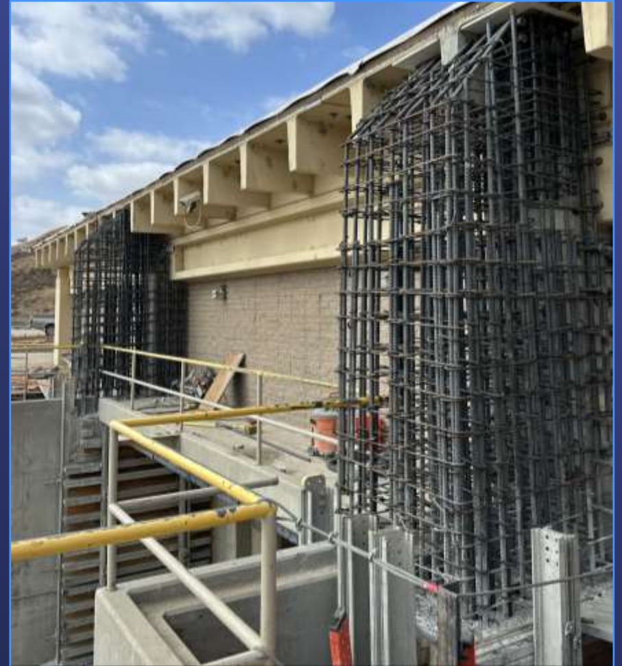
Column Strengthening of Foothill HEP/PCS
