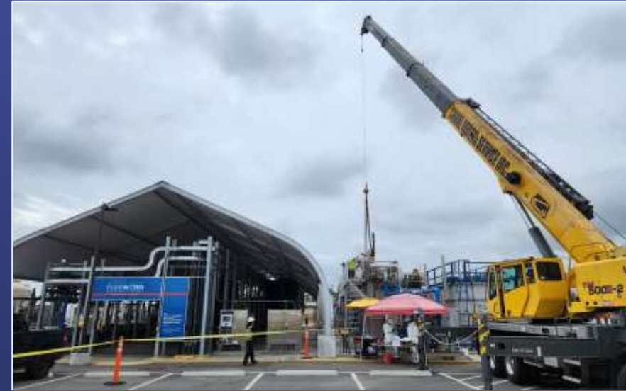
Crane Removing MBR for Inspection
