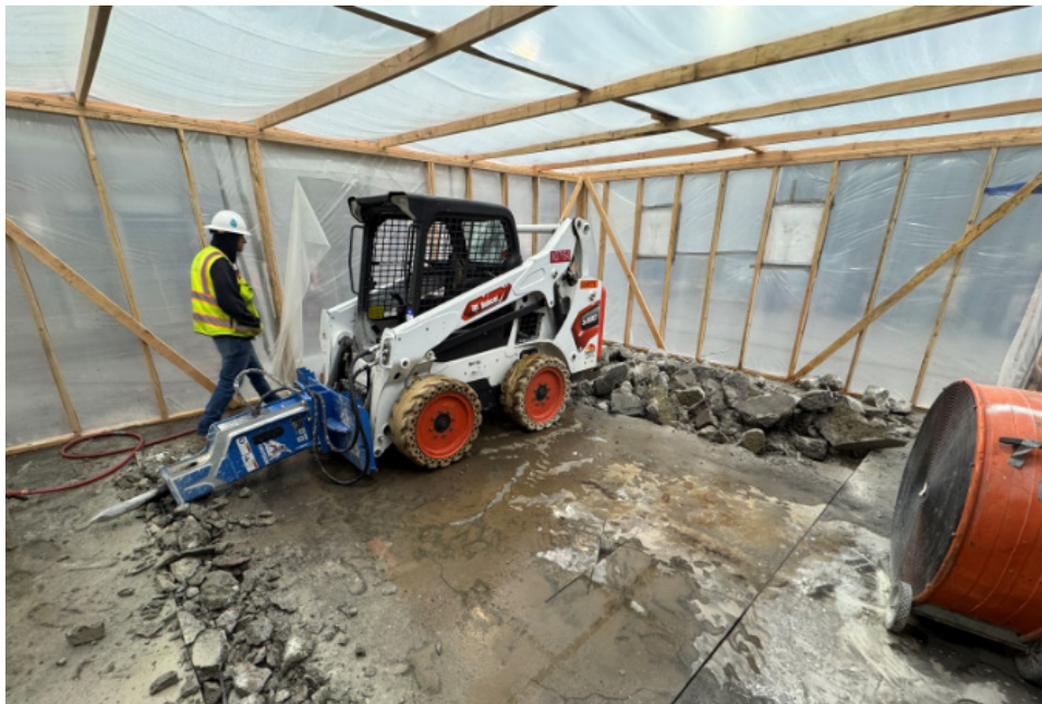
La Verne Shops Improvements —Slab Demolition for Vertical Band Saw Foundation at the La Verne Fabrication Shop
