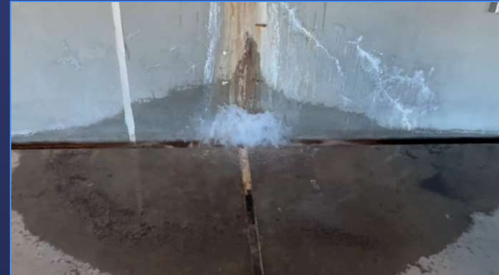
Expansion Joint Leak
