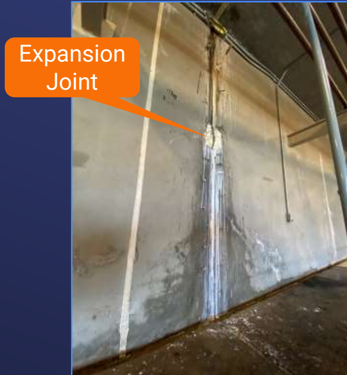
Expansion Joint Leak
