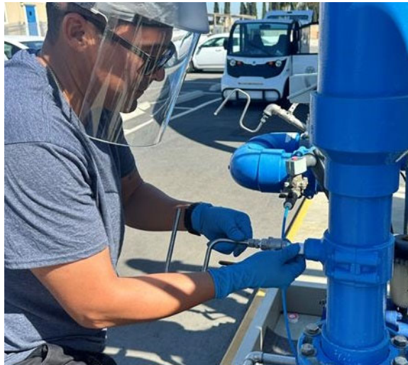
Staff installing a membrane bioreactor filtrate sampling tap at the Napolitano Innovation Center demonstration plant
