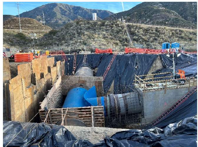
Contractor replacing a 35-foot section of 120-inch welded steel pipe (left) and installing the interconnection tee for the Rialto Pipeline to the Inland Feeder (right)
