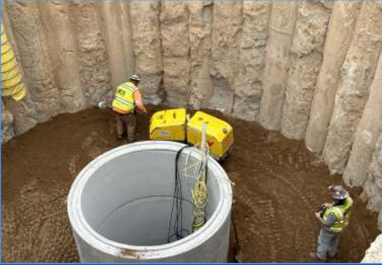
Compaction of Backfill in Southern Tunnel Shaft
