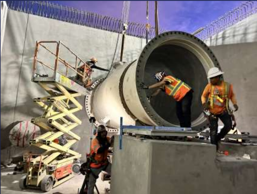
Valve Vault Pipe Installation
