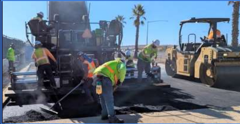
Paving Asphalt at Van Buren Blvd. City of Riverside
