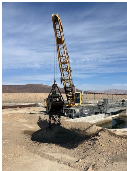
Canal sand trap cleaning at Eagle Mountain pumping plant
