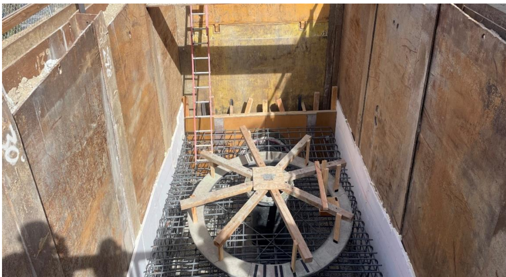
Stage 2 – concrete encasement forming and rebar installation for the pipe closure at an access site
