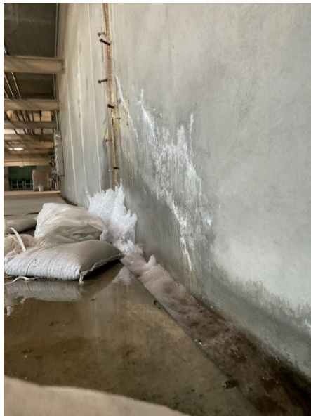
High leak flow (left) and reduced leak flow (right) in Weymouth ozone contactor effluent channel
