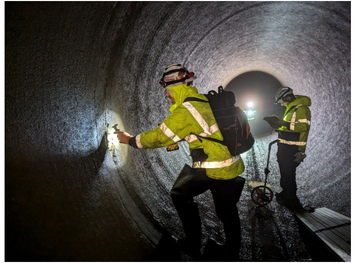
Dewatering at a blowoff (left) and staff performing inspection of welded steel pipe (right) for the Rialto Pipeline
