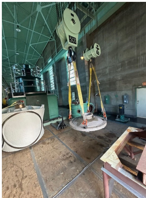
Gene Unit 1 discharge valve plug and headcover being transported for machine work
