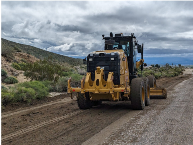
Motor grader performing routine maintenance along the CRA
