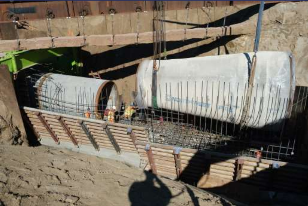
Pipe Fitting Placement
