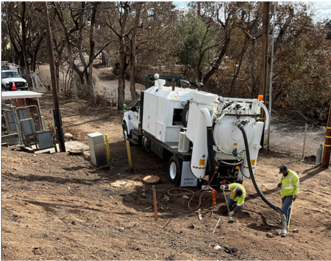
Staff operating vac truck to locate lines (left) and excavating for new interconnection feed line (right) at the Lake Reservoir site
