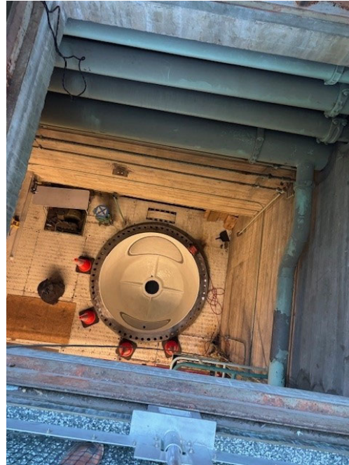
Gene Unit 1 discharge valve body after blasting and coating
