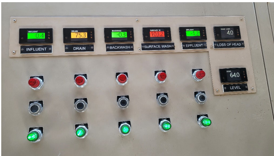
Control panel with new digital displays (left) and staff programming filter console display screens (right)
