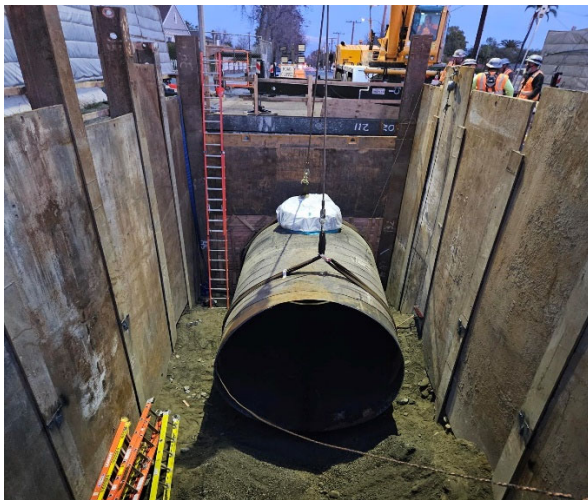
Contractor replacing a 35-foot section of 120-inch welded steel pipe (left) and installing the interconnection tee for the Rialto Pipeline to the Inland Feeder (right)
