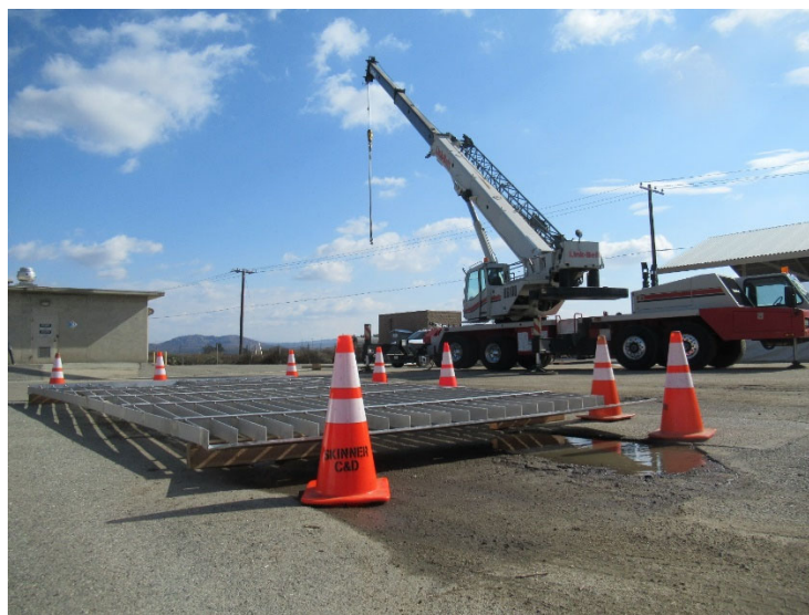
A section of stainless-steel grating after removal from the bypass structure
