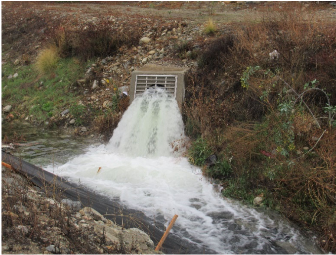
Dewatering at a blowoff (left) and staff performing inspection of welded steel pipe (right) for the Rialto Pipeline
