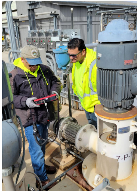
Staff observing vibration readings for a cooling water pump at the Mills plant
