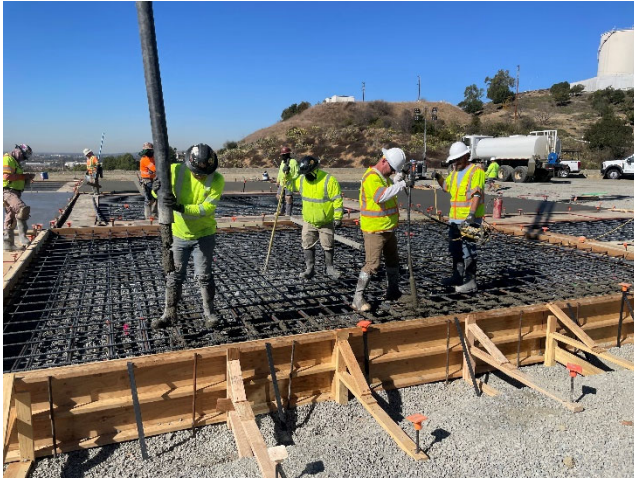
Staff placing concrete for the helicopter pad at the Diemer plant site
