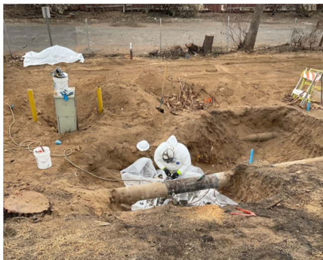
Staff performing coating abatement at the Lake Reservoir site
