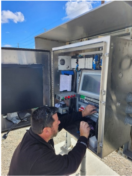
Staff performing final setup of new PLC (left) and new service connection flow meter, monitoring, and power cabinets after final installation (right)
