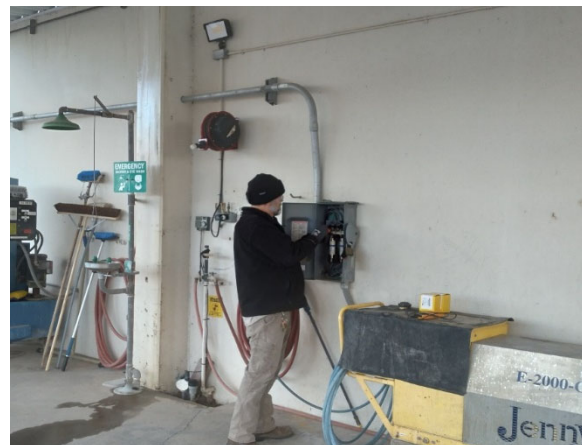
Fabricating and welding a new pipe tee (left) and installing a new transfer switch (right)
