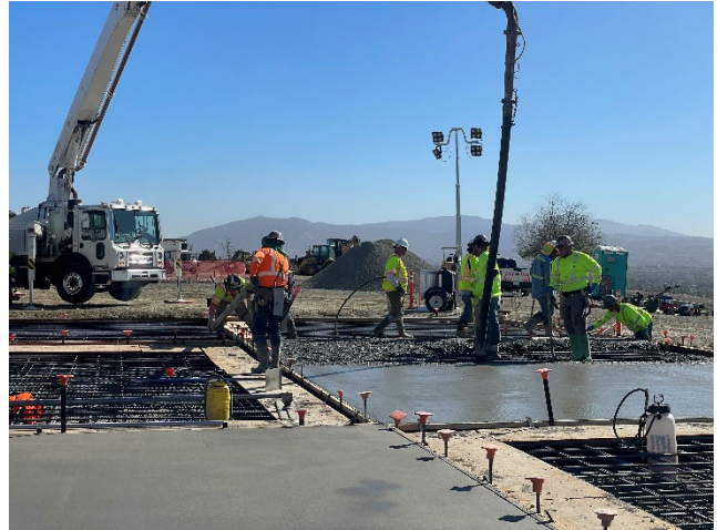
Staff placing concrete for the helicopter pad at the Diemer plant site
