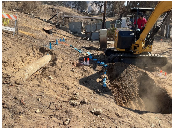
Staff operating vac truck to locate lines (left) and excavating for new interconnection feed line (right) at the Lake Reservoir site
