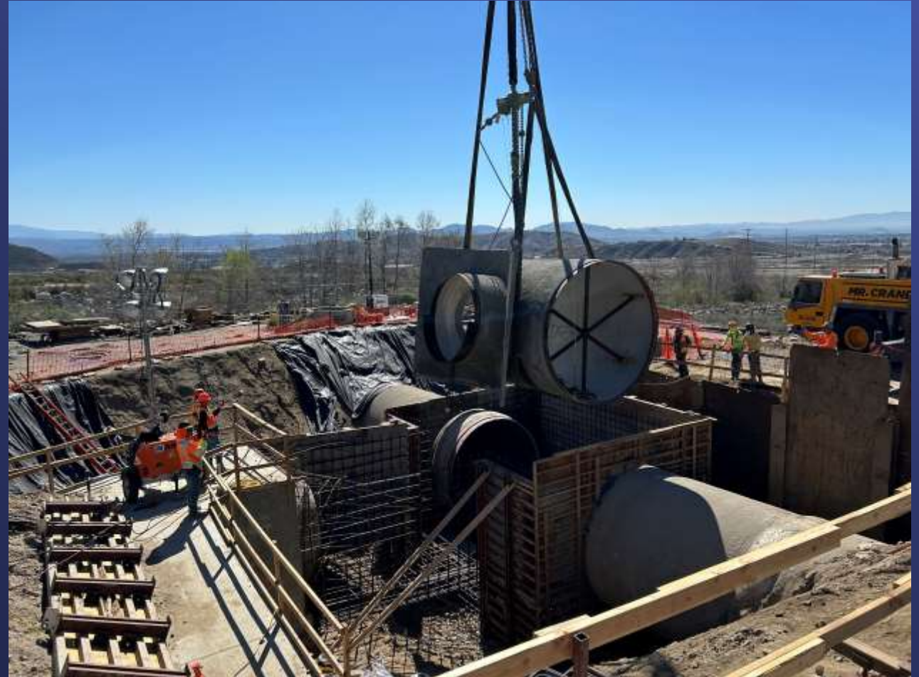
Installation of 96" Diameter Tee
