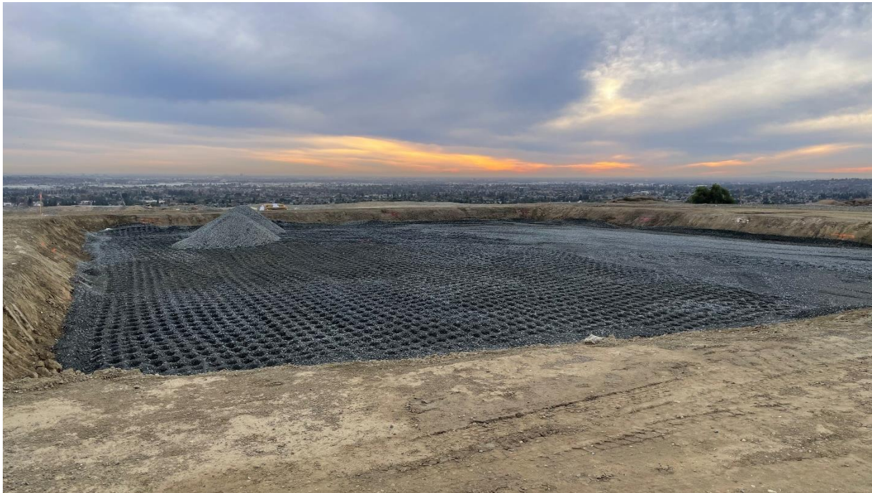
Helicopter landing pad at the Diemer plant – placing crushed aggregate for the pad subgrade
