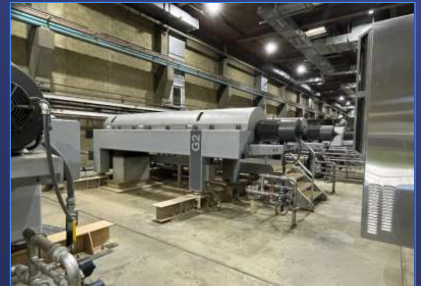
Centrifuges at OC Sanitation District
