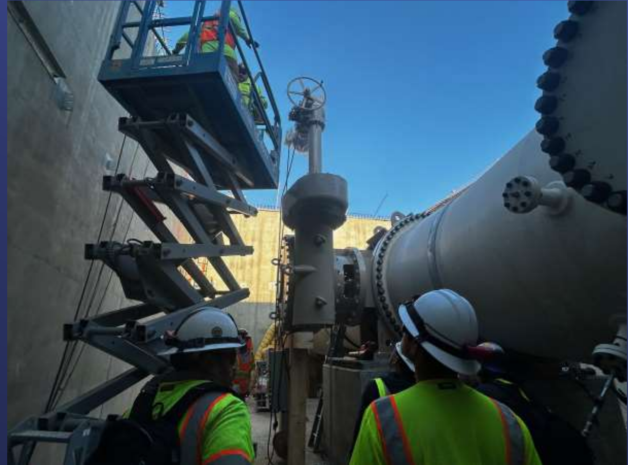
84-Inch Diameter Valve Fit Up
