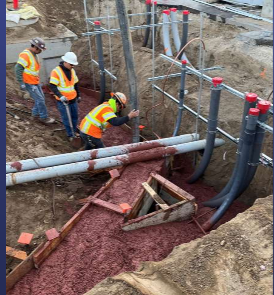
Electrical Duct Bank
