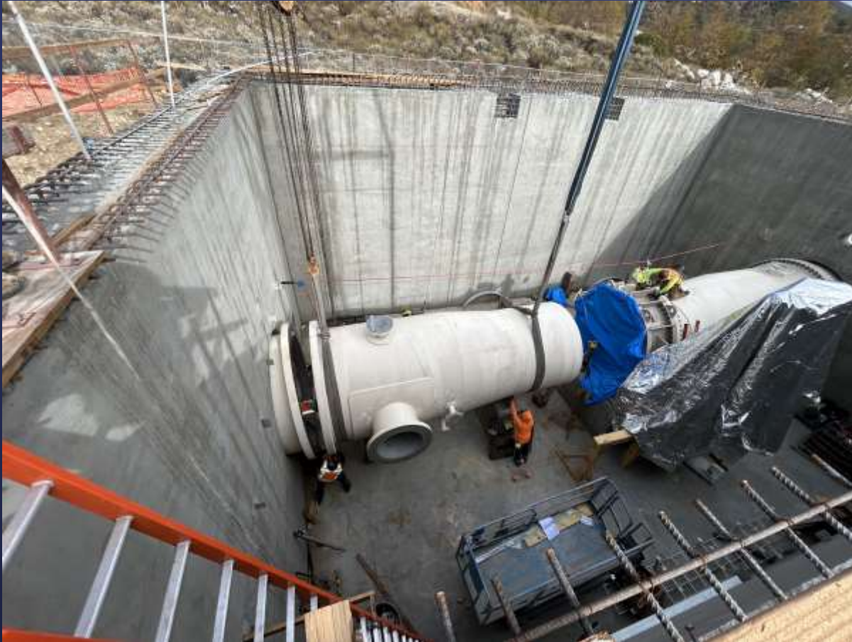
Pipe Reducer Installation
