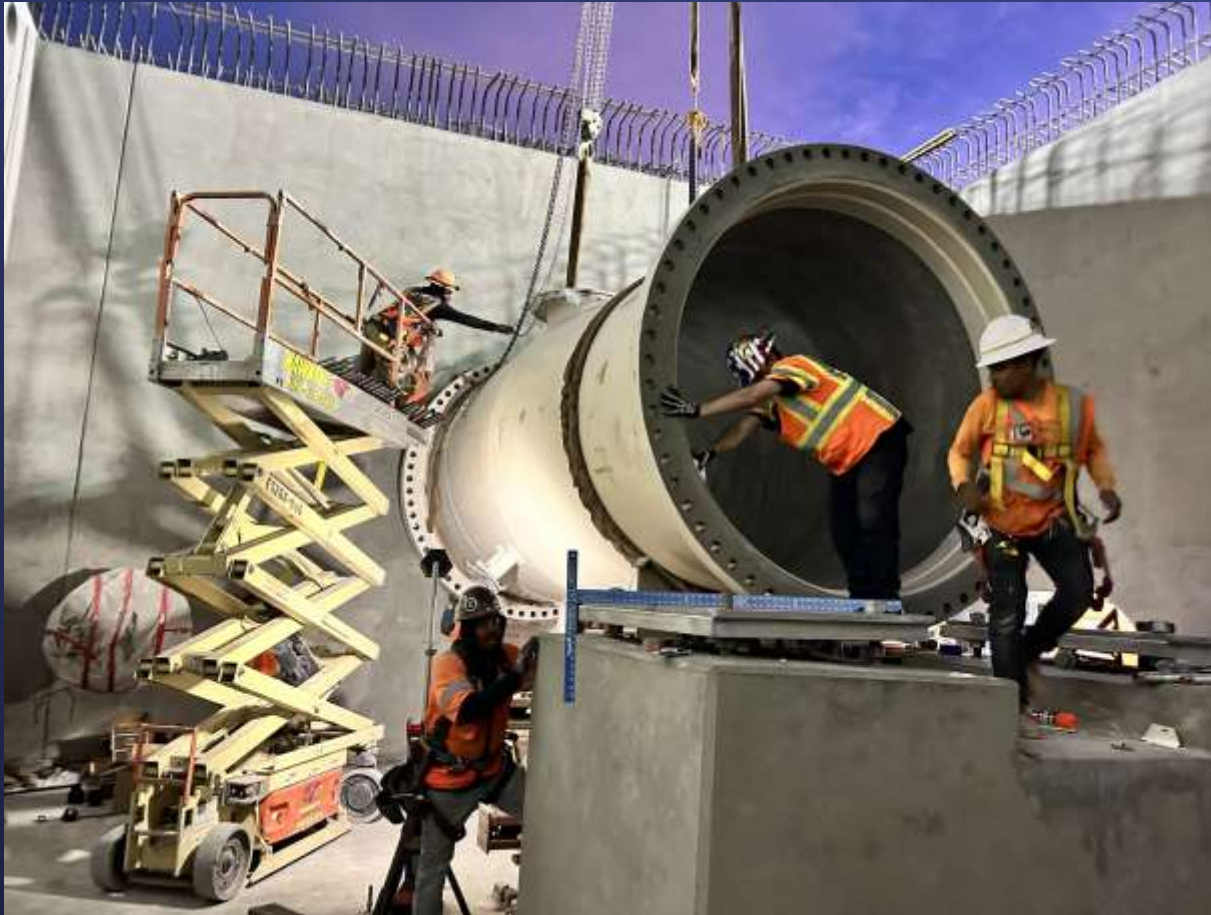
Valve Vault Pipe Installation
