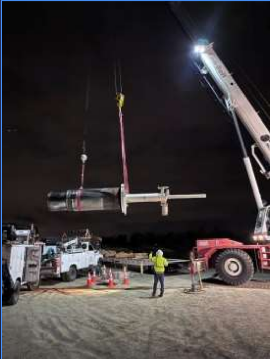
Sleeve valve assembly w/ actuator
