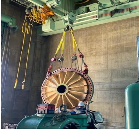
Discharge Valve Cover being removed.
