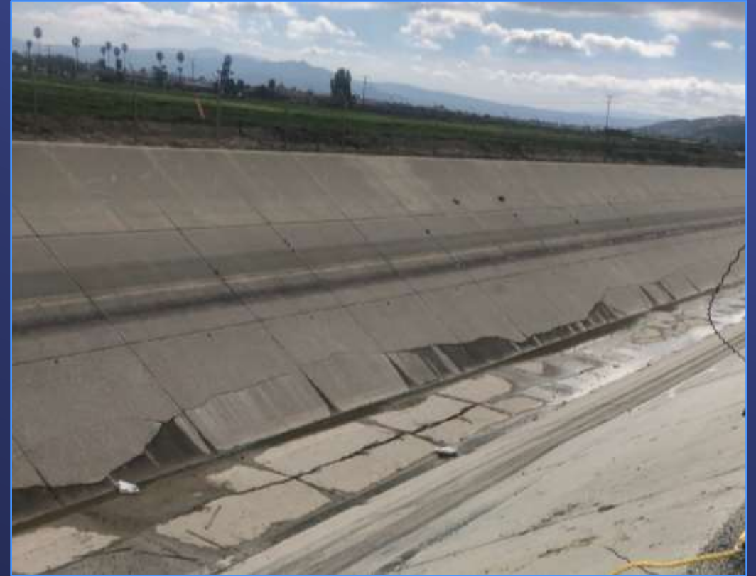
Damaged concrete liner
