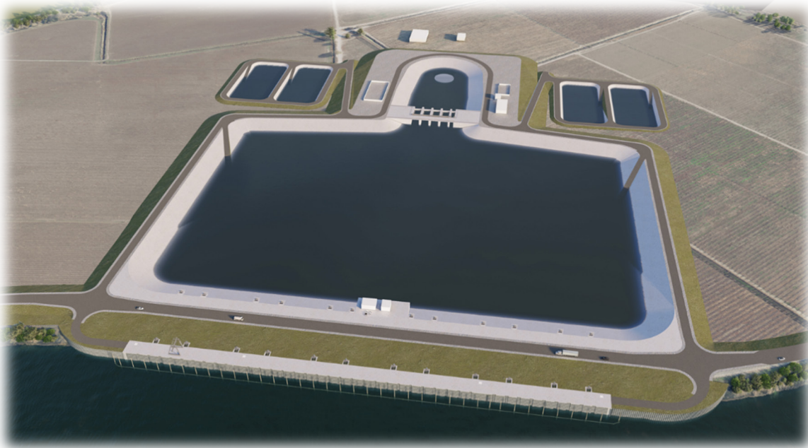
Figure 2-3. Conceptual On-bank Intake and Sedimentation Facilities
