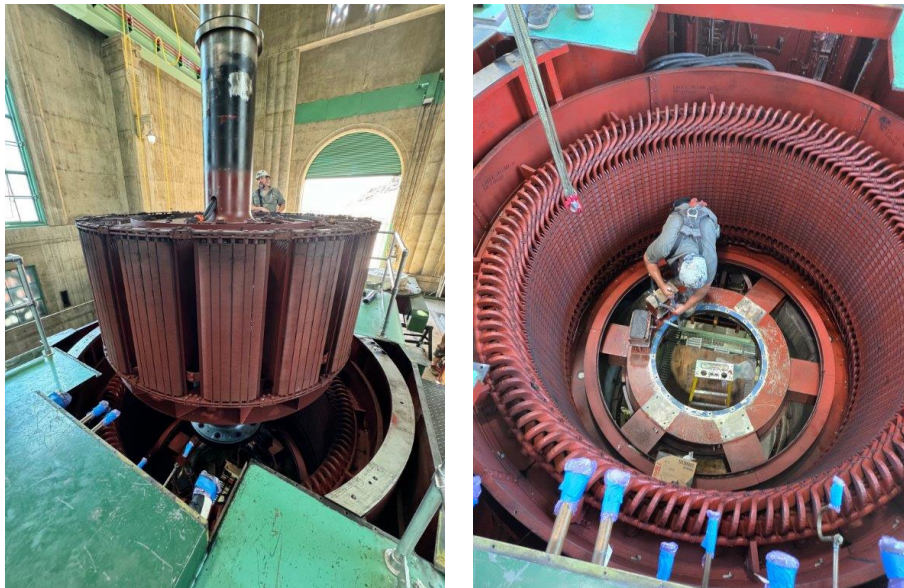
Removing the rotor and hydraulic jacks from Eagle Mountain Unit 9 stator
