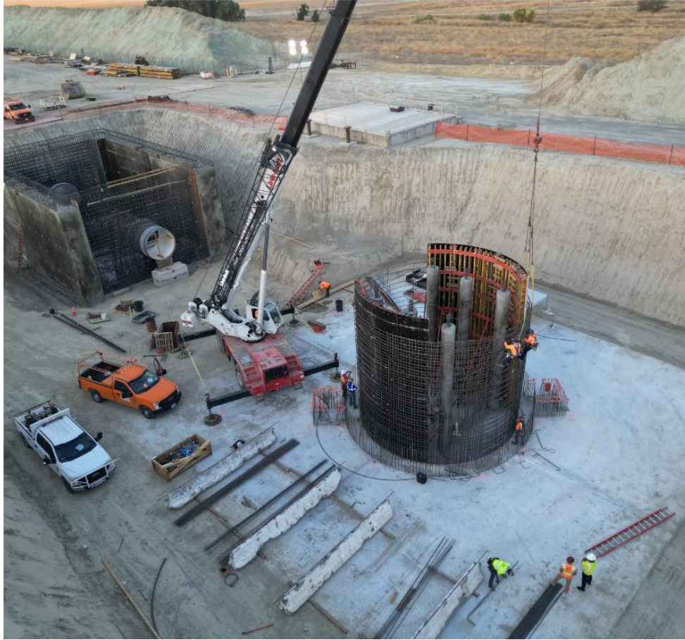
Inland Feeder - Badlands Tunnel Surge Protection – Installation of Rebar at the Surge Tank Foundation
