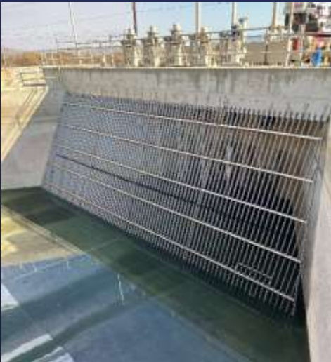
New Trash Rack East Lake Skinner Bypass
