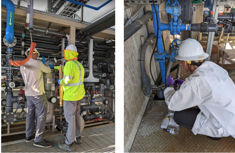
Staff replacing cartridge filters ahead of reverse osmosis system (left) and collecting samples during VOC spike testing (right)
