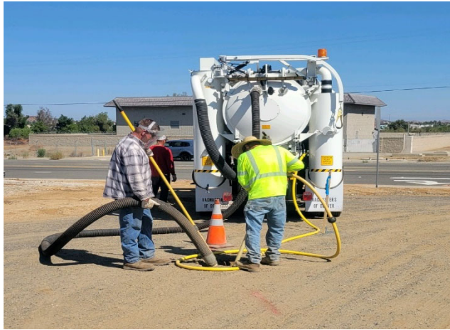
Potholing for existing utilities (left) and backfilling over new conduit for fiber optic cable (right)
