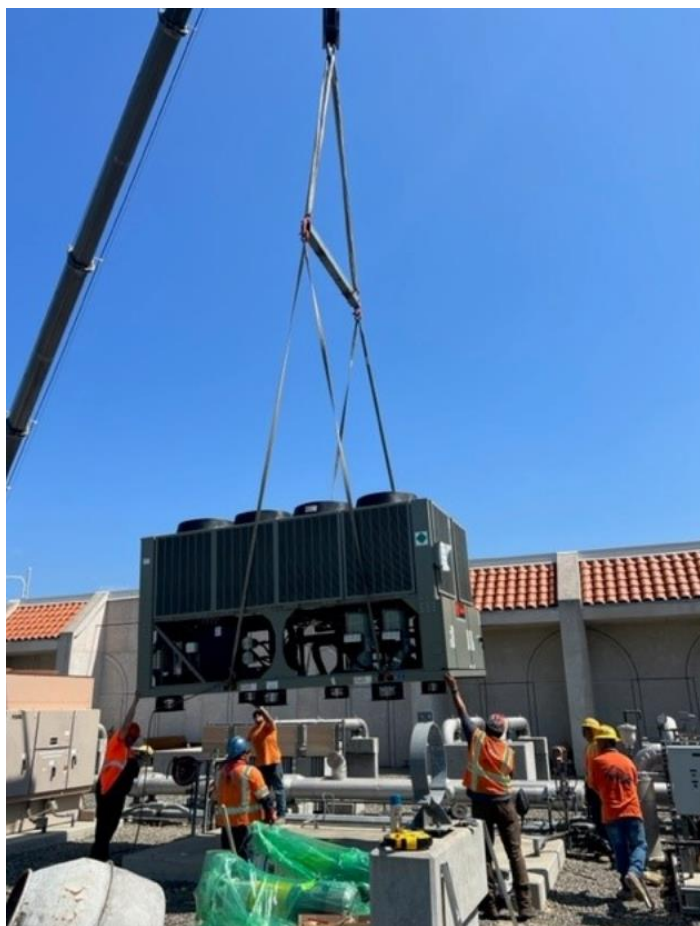
Service Connection OC -88 Chillers Replacement – Chiller Installation
