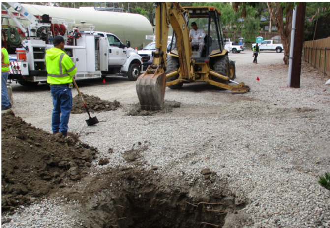
Excavating for percolation test pit (left) and conducting percolation test (right)
