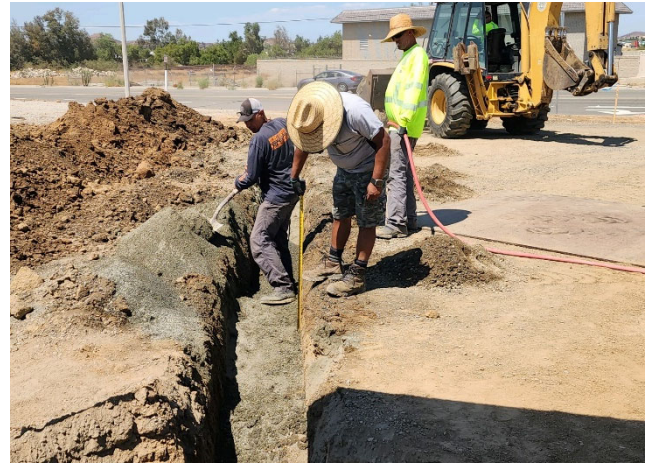
Potholing for existing utilities (left) and backfilling over new conduit for fiber optic cable (right)
