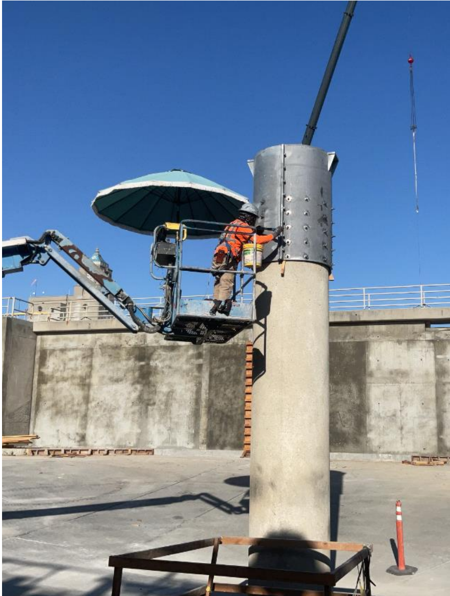
Weymouth Basins 5–8 and Filter Building No. 2 Rehabilitation – Installing the clarifier column cap at Basin 6, view to the west.
