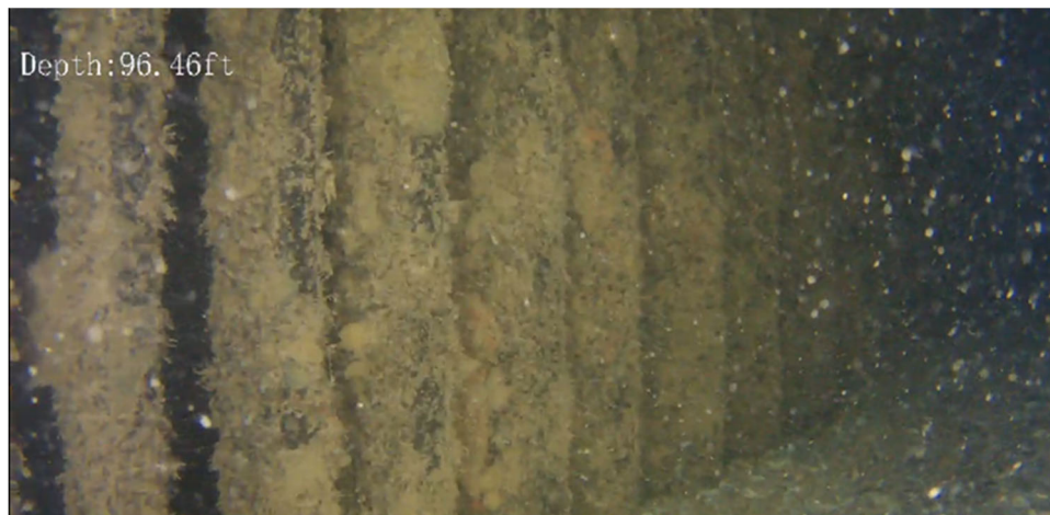
Inspection of valve inlet trash rack
