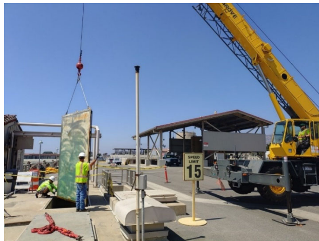
Mechanics removing filter effluent channel drop gate at the Weymouth plant
