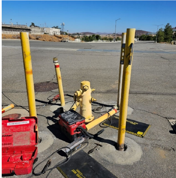
Replacement of bollards protecting fire hydrant with new, taller bollards for increased protection and visibility
