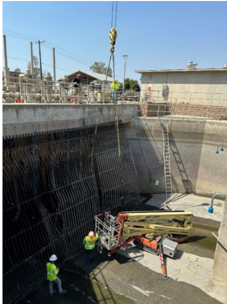
Staff installing a new trash rack at the East Lake Skinner Bypass
