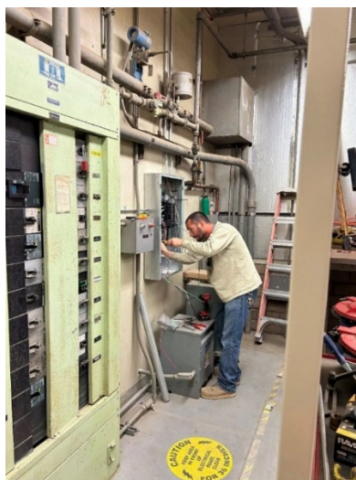
Staff replacing electrical distribution panel in the Mechanical, Electrical, and Fleet shop at the Skinner plant
