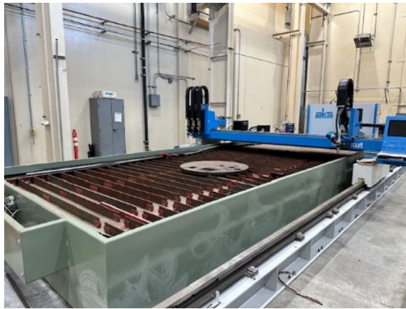
New Plasma Arc Cutting System Installation In-Progress
