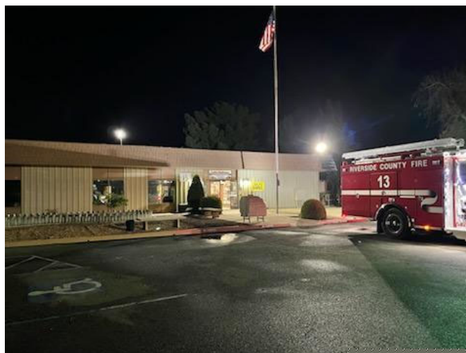
Tin Fire at Lake Mathews Administration Building
