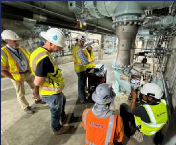
Testing Refurbished Effluent Valve at Filter 41
