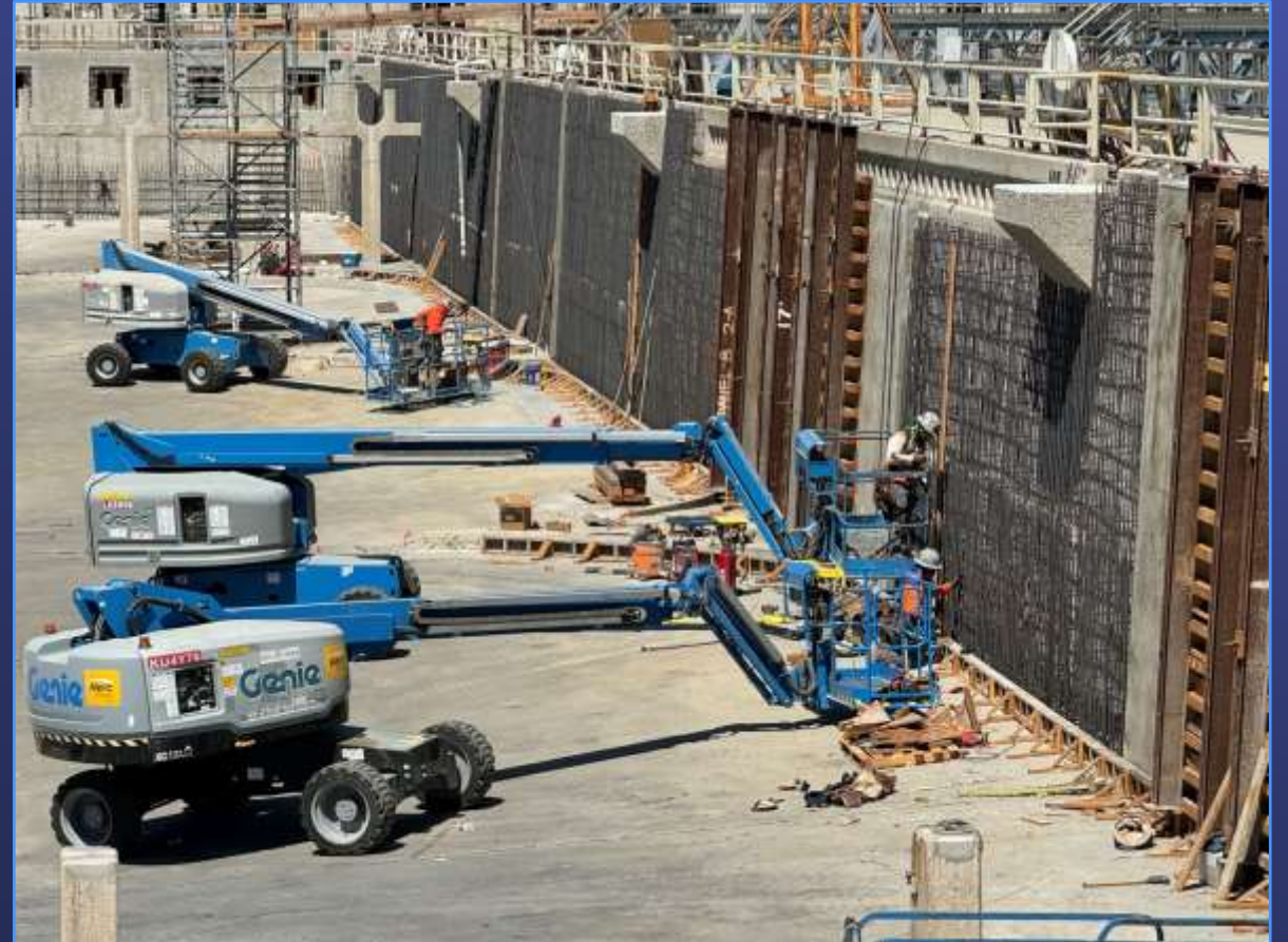
Preparing Walls for Formwork at Basin 6
