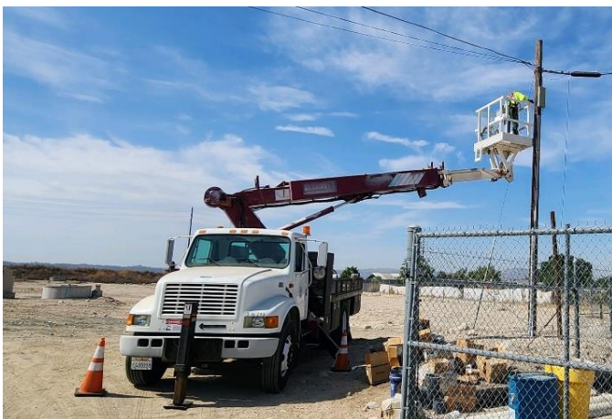
Installing a pull rope for the new fiber optic cable
