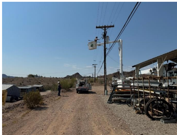
Staff replacing a 2300/480V transformer at the Gene pumping plant
