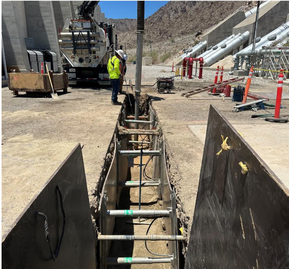
CRA Storage Buildings—Julian Hinds FMS 8 inch HDPE Fire Water Line Trench Hydro Excavation
