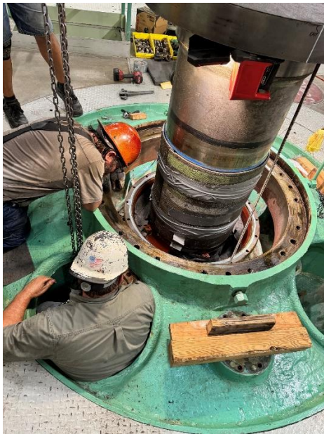
Staff disassembling a pump at the Eagle Mountain pumping plant
