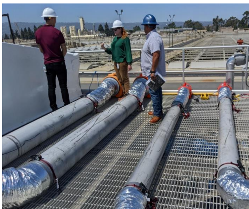
Installation of bioreactor materials in preparation for acetone spiking test at the NIC
