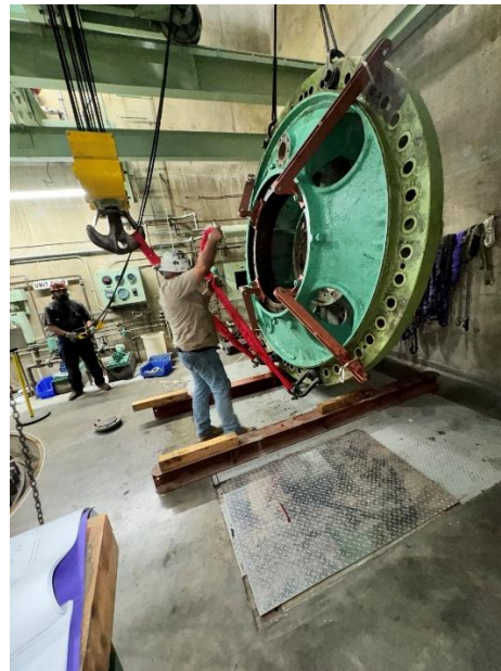
Staff disassembling a pump at the Eagle Mountain pumping plant
