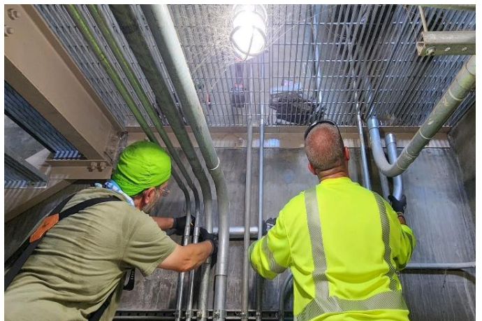
Routing conduit inside the structure
