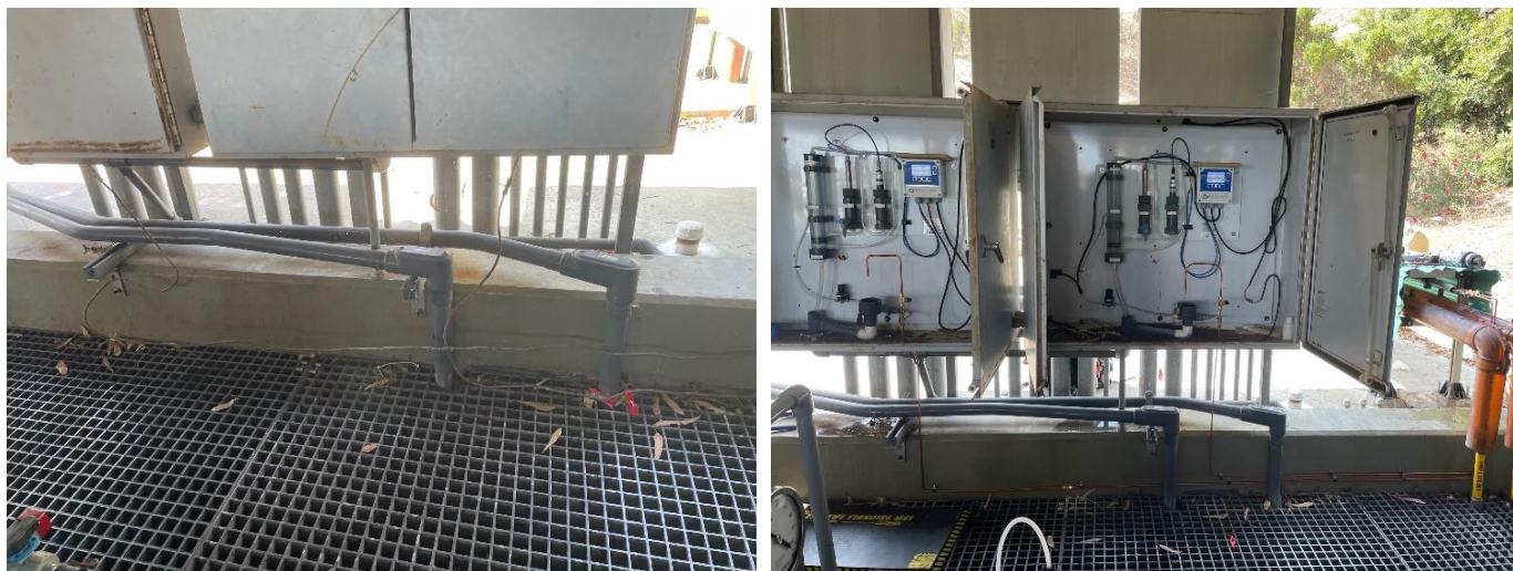
Garvey Reservoir tank farm water quality analyzers
