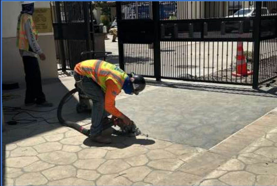
Saw-cutting a Concrete Joint Near Gate 4
