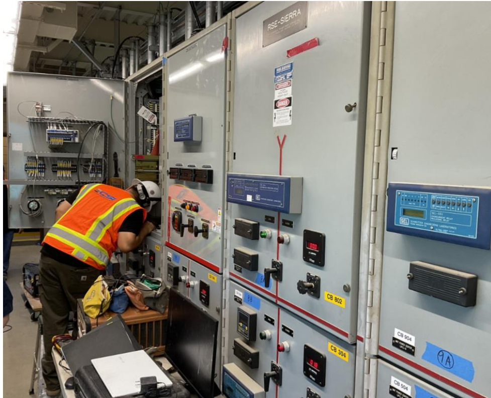
Mills Electrical Upgrades—ORP Switchgear New Door Testing
