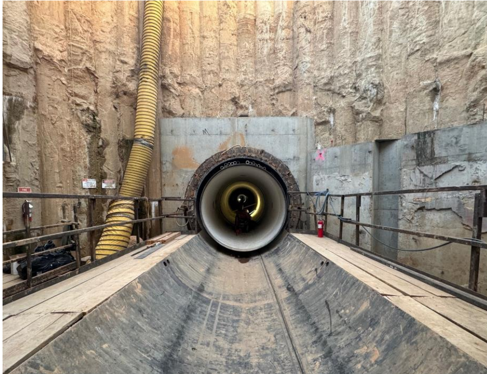
Perris Valley Pipeline Tunnels—Drive 2 Carrier Pipe Installation
