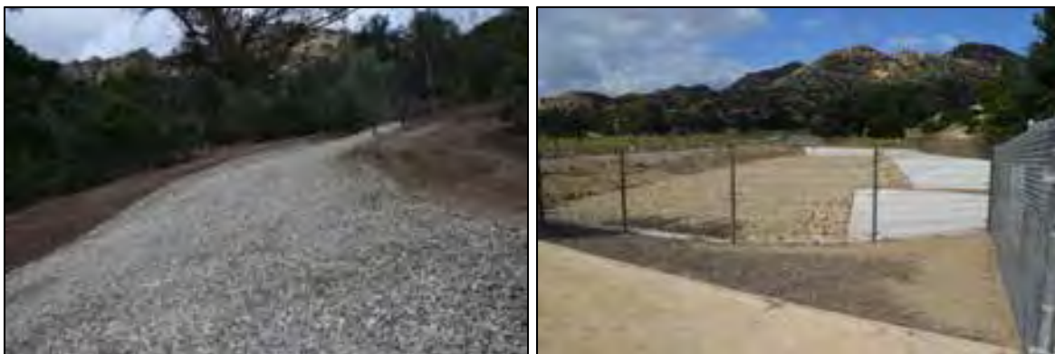
Figure 5 - Stone Lined Stream and Park Detention Basin
