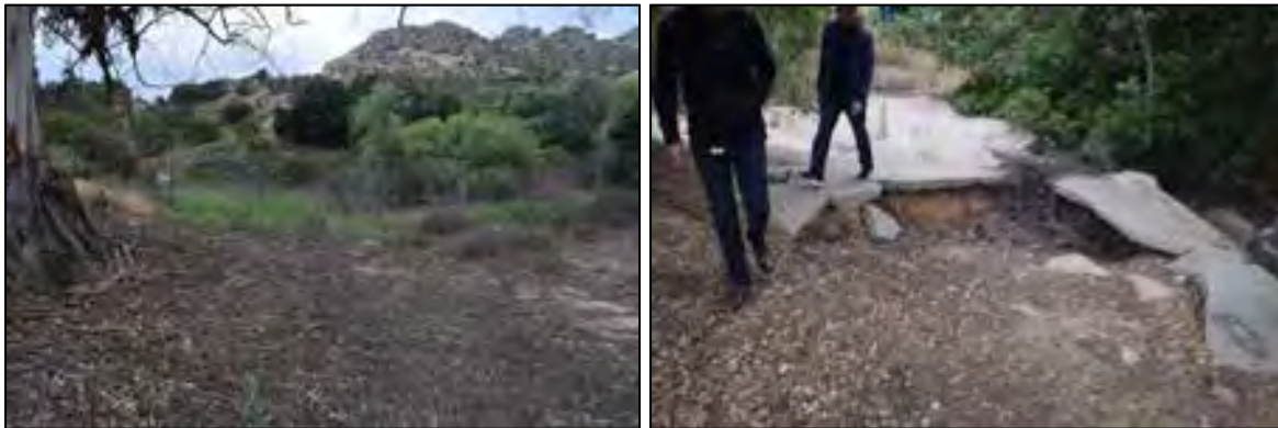
Figure 4 - Earthen Flood Control Basin and Broken Spillway
