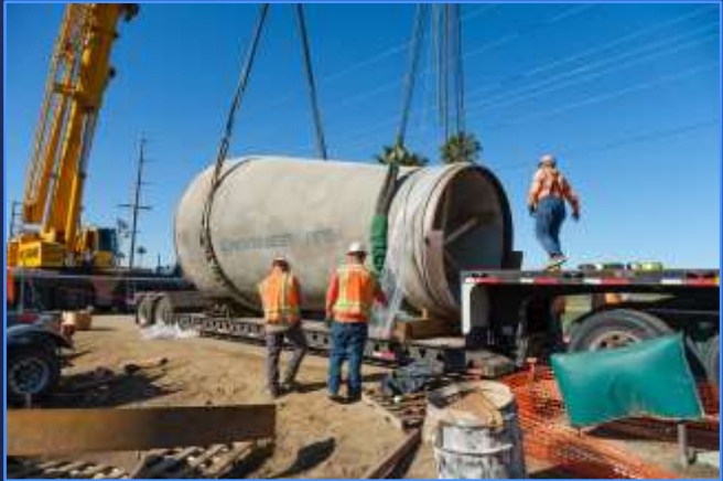
A Section of the Bypass Pipeline Being Installed
