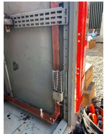
Installation of new buss
