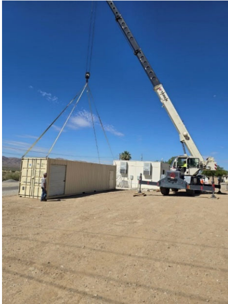
Installation of storage and office buildings at Hinds pumping plant
