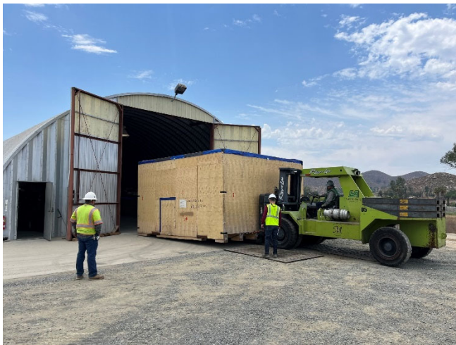
Delivery and storage of three 84-inch butterfly valves with actuator (each weighing 60,000 pounds)
