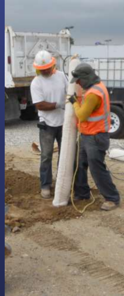
Anode Installation
