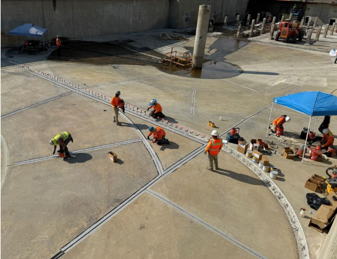
Weymouth Basins 5–8 and Filter Building No. 2 Rehabilitation—Installing Joint Sealant at Basin 5
