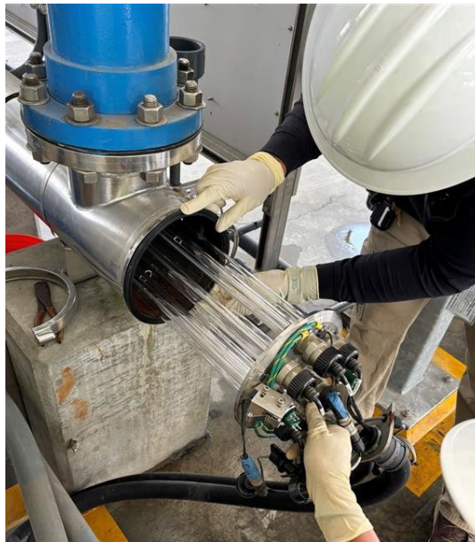
Staff replacing UV lamps for the advanced oxidation system at the PWSC NIC demonstration plant
