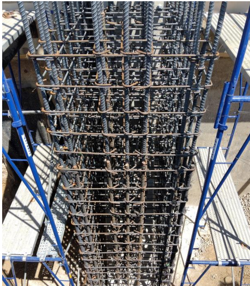
Foothill Hydroelectric Plant and Control Building Seismic Upgrade— Rebar Placement at Hydroelectric Plant Column
