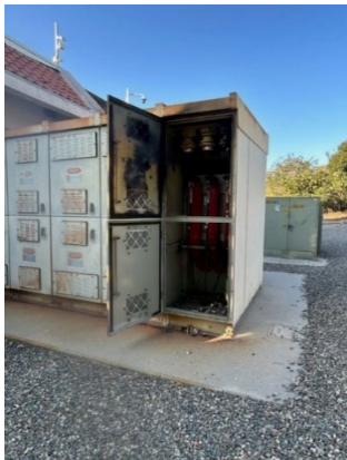
Failed surge arrester on incoming power line
