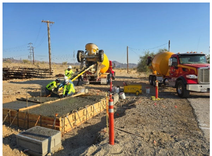
Staff placing concrete at the Eagle Mountain village
