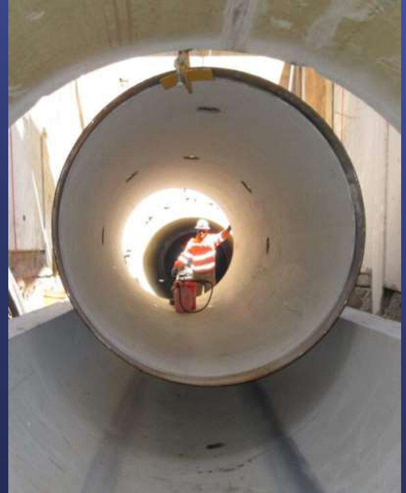
Allen-McColloch Pipeline Relining
