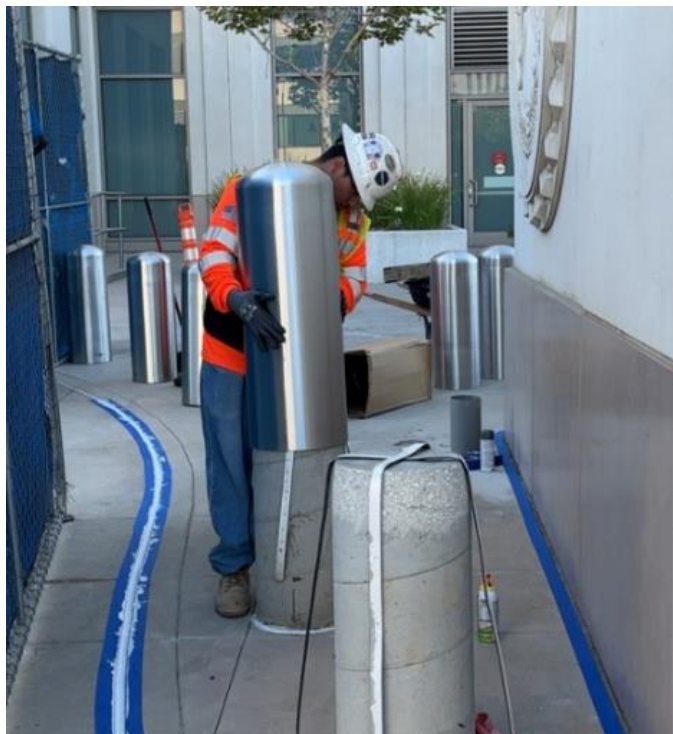
Headquarters Physical Security Upgrades—Stainless Steel Cover Installation on Bollard at Building Entrance
