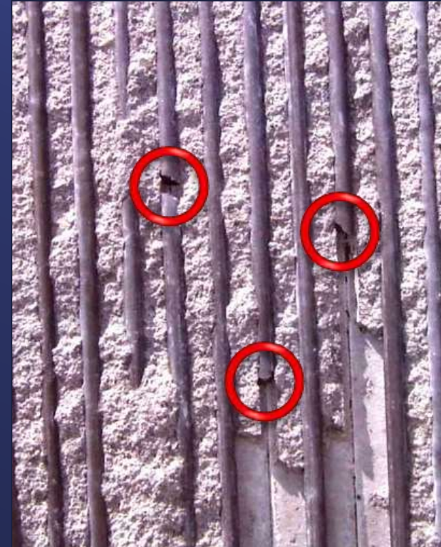
Broken Prestressing Wires
