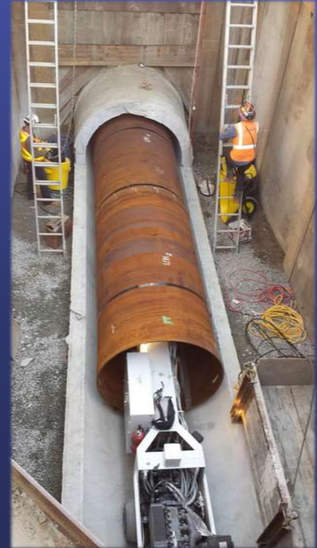
Second Lower Feeder Relining
