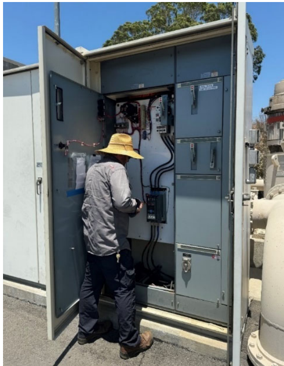
Staff installing electrical soft starters for Lake Skinner Outlet Tower chlorine pumps
