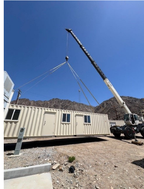
Installation of storage and office buildings at Hinds pumping plant
