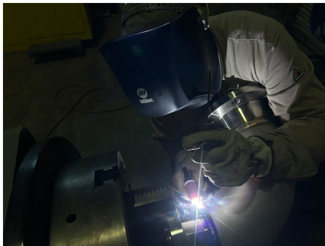
Staff TIG welding stainless steel piping for the chiller system at Eagle Mountain
