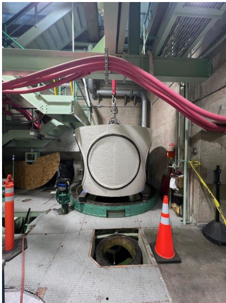
Staff removing a discharge valve plug for inspection and testing at Iron Mountain pumping plant
