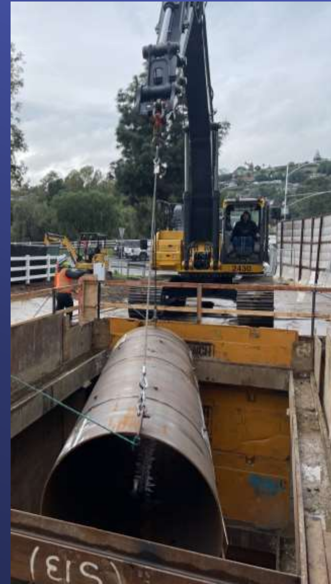
Second Lower Feeder Relining
