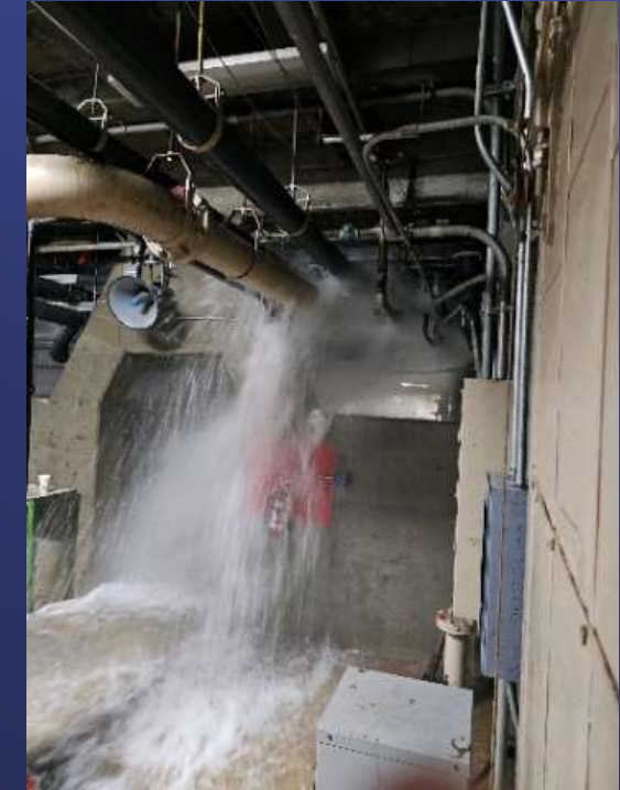
Weymouth Domestic Water Line Leak June 2024
