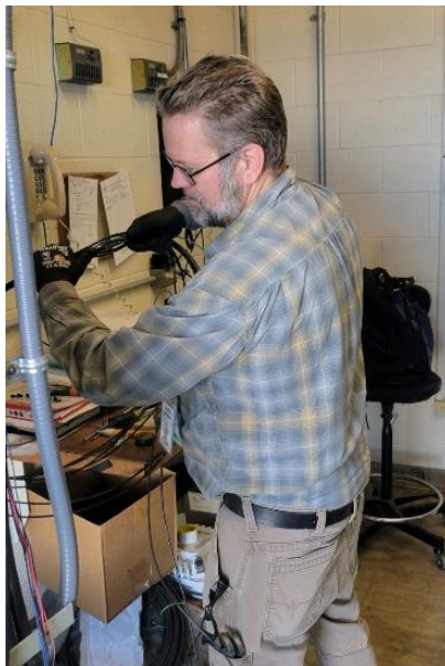
Staff installing the new rectifier system at the Detention Peak communications site
