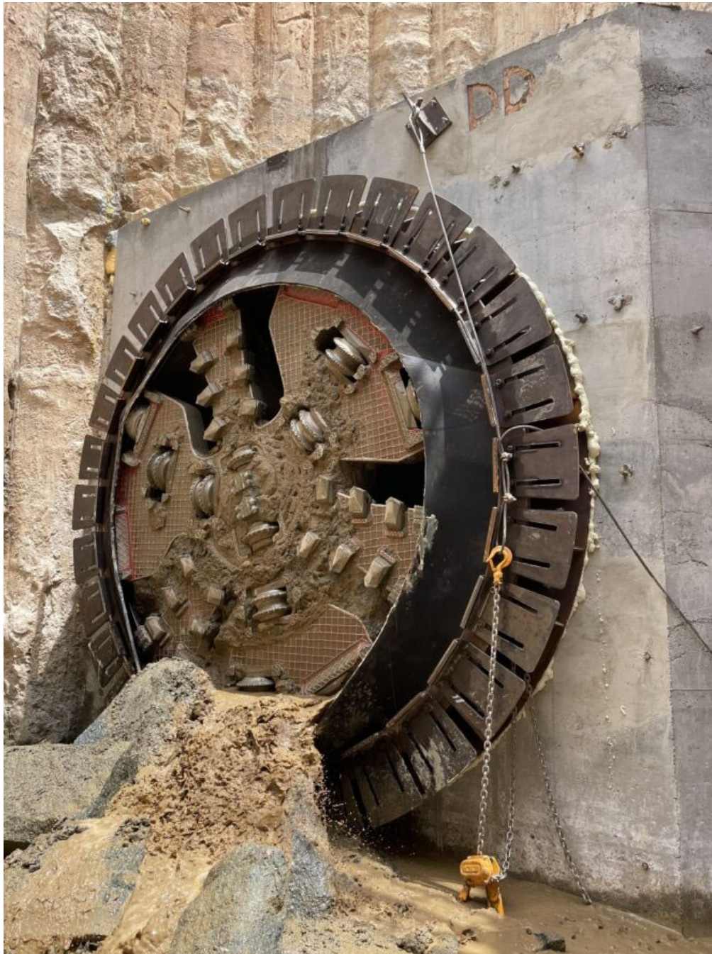
Perris Valley Pipeline—Hole-through TBM at second shaft
