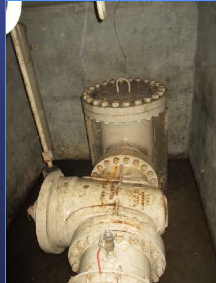
Existing deteriorated blow-off valve, typical of six
