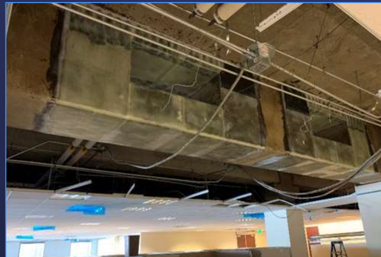
Interior Beam with Fiber Reinforced Polymer (FRP)
