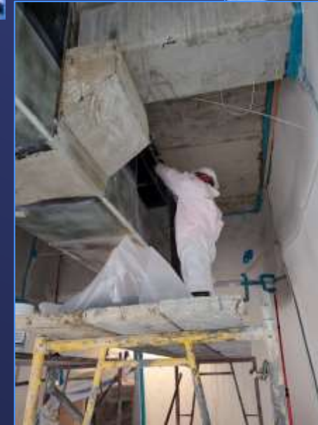
Interior Beam with Fiber Reinforced Polymer (FRP)
