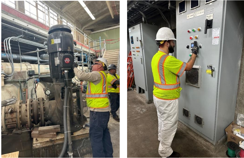
Terminating cables and programming the new ASDs to control pumps at the Weymouth plant
