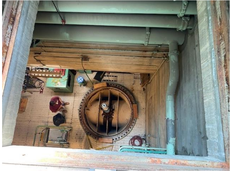
Discharge Valve repair at Gene pumping plant
