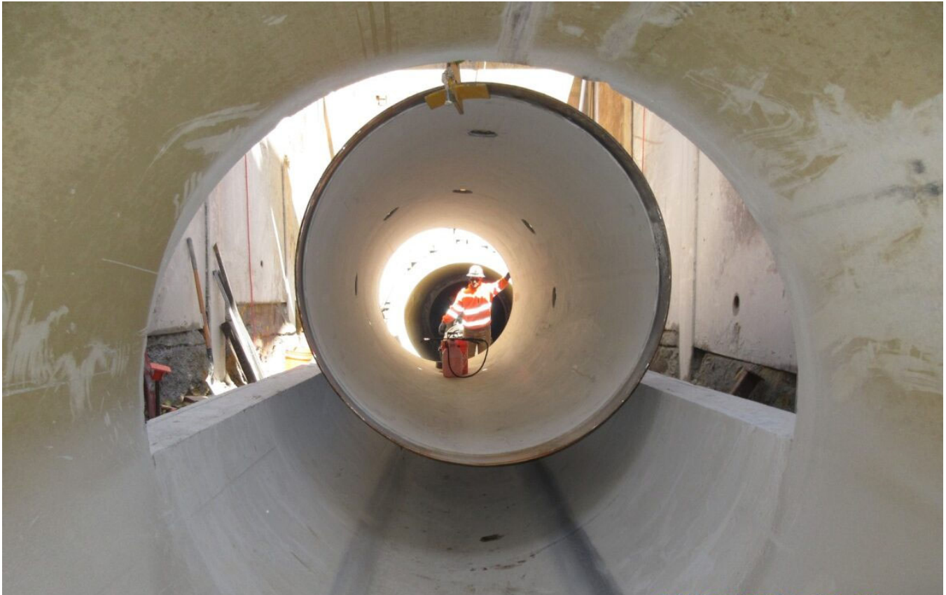
Allen-McColloch Pipeline Urgent Relining—New pipe liner installation
