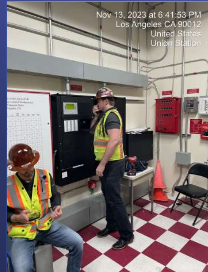
Testing New Fire Alarm System
