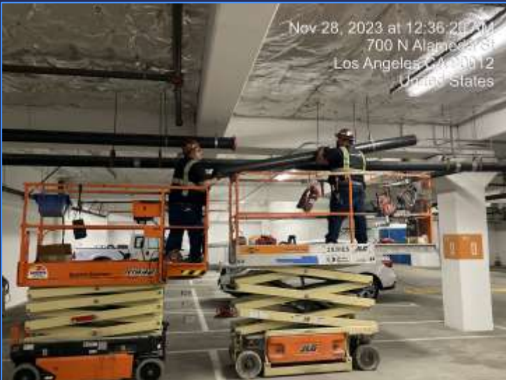
Fire Sprinkler Level P1 Replacement (Completed: 2024)
