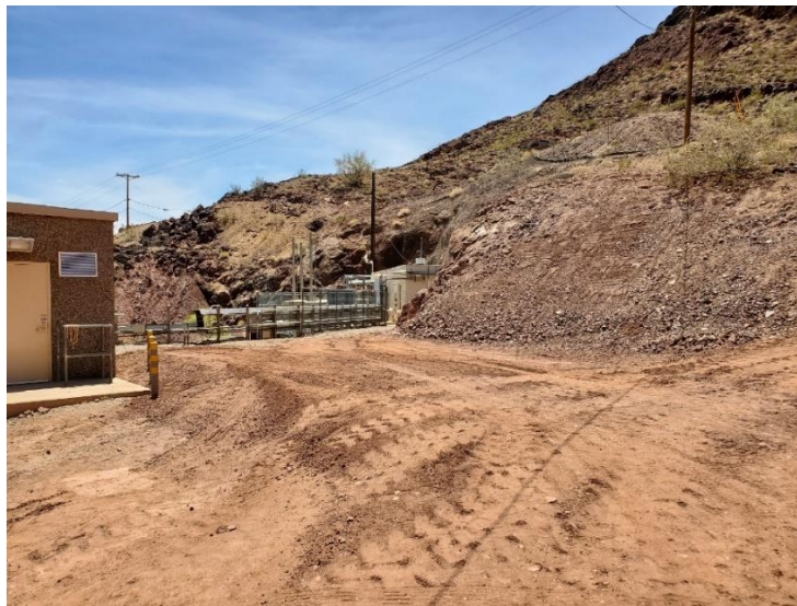
New crane pad for better access to perform maintenance
