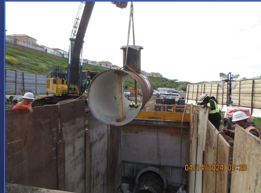
Installation of Closure Pipe
