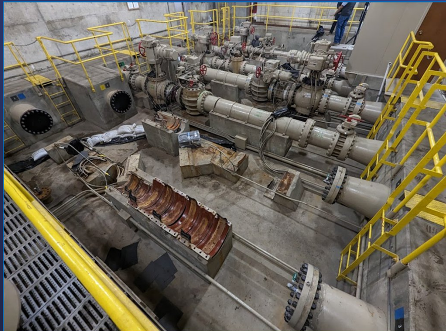
Covina Pressure Control Structure - Valve Replacement
