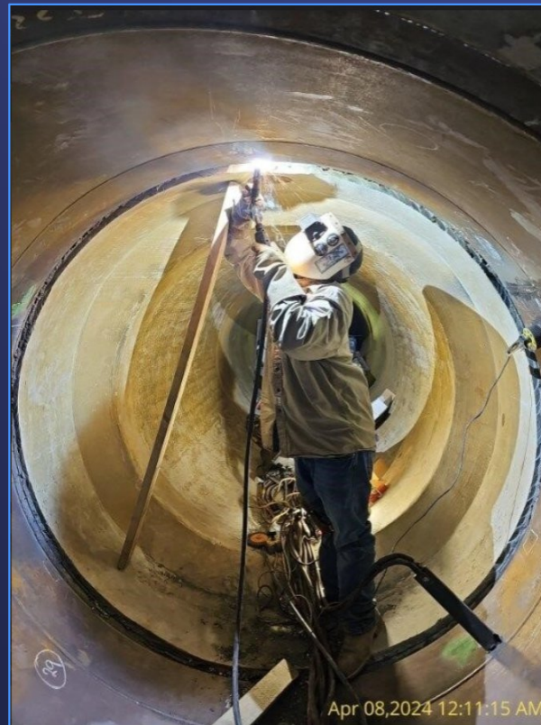
Circumferential Welding of Steel Pipe
