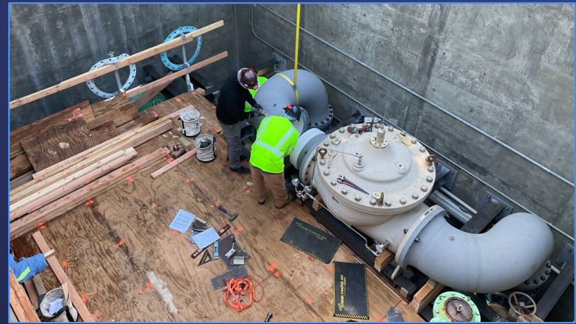
Installing PRV Near OC-88
