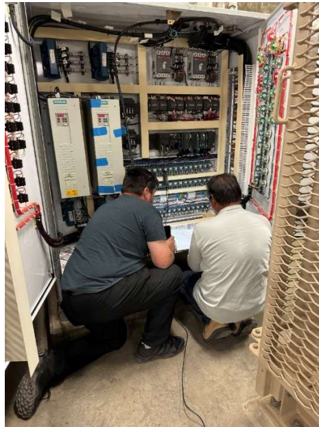
Staff repairing instrumentation PLC for the fish screens at DVL
