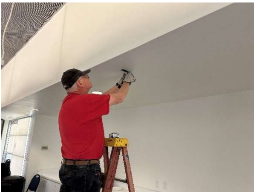
Staff installing a new cut-in box (left) and electrical conduit (right)
