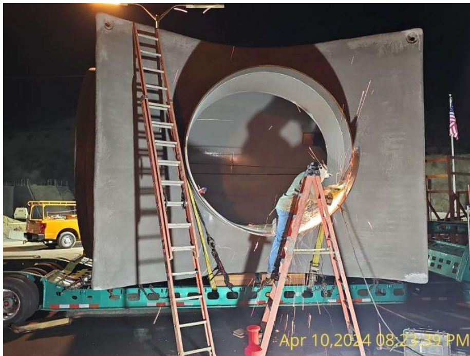
Wadsworth Pumping Plant Bypass—Welding Buttstrap for the Tee Section
