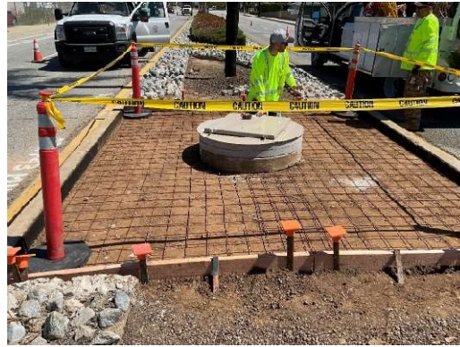
Staff excavating concrete slab area (left) and reinforcing wire installation (right) to enhance safe access at a Middle Feeder structure
