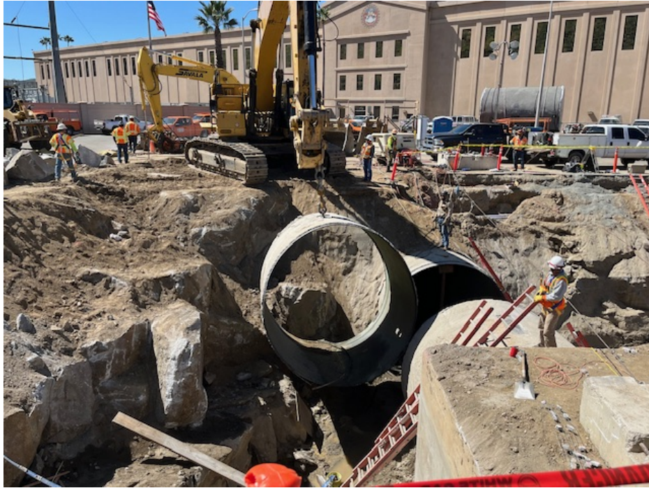
Wadsworth Pumping Plant Bypass—moving Section of Pumphouse Conduit
