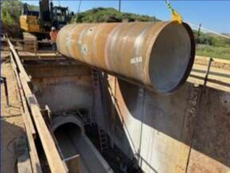
Lowering new liner pipe into existing PCCP pipe
