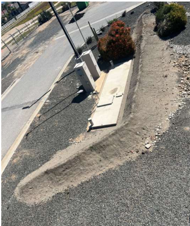
New berm built to prevent water intrusion into the vault
