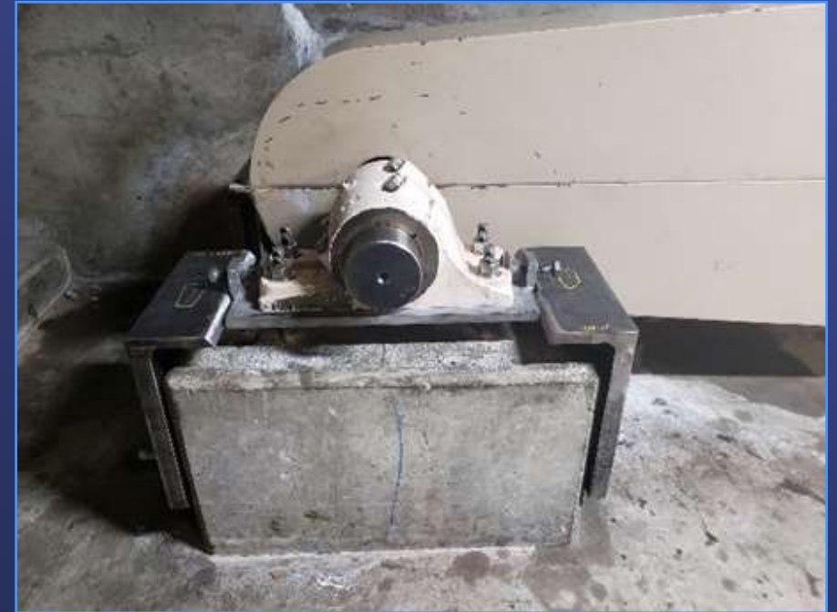
Structural reinforcement at bearing completed at Basin 10
