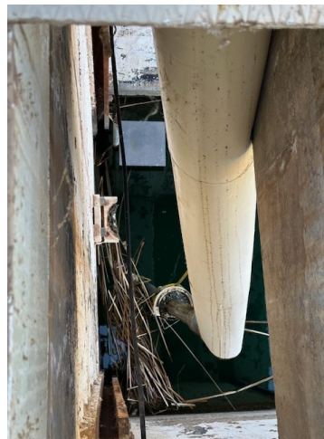
Damaged gate shaft (left and center) and as-found actuator assembly (right) for the gate at Copper Basin
