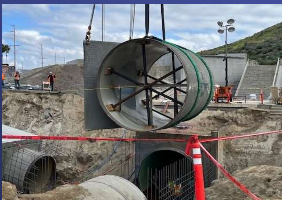
Wadsworth PP Tee Installation
