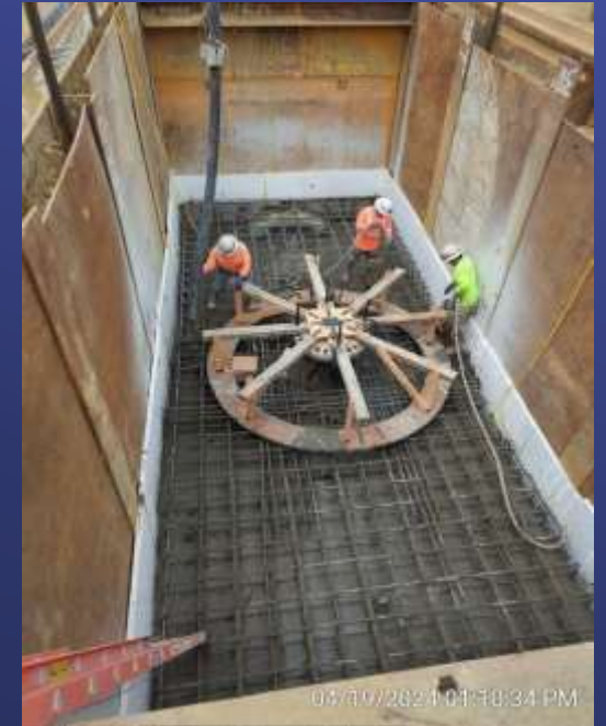
Concrete placement at new access location
