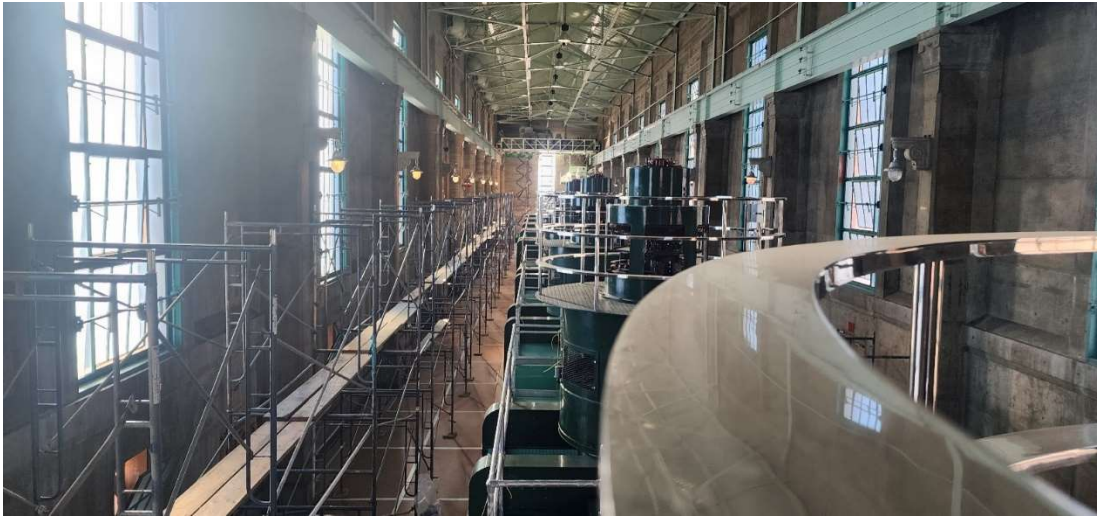
Motor room main crane replacement at Intake pumping plant
