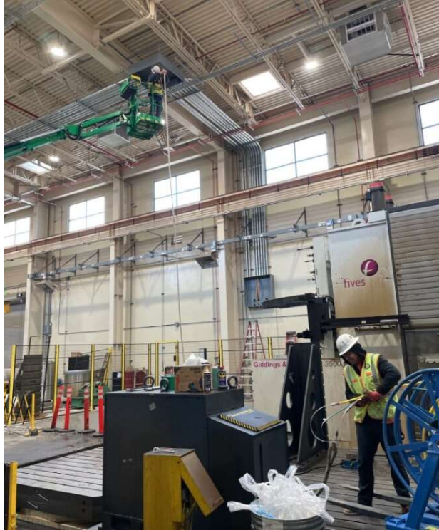
La Verne Shops – Installation of Electrical Conduits
