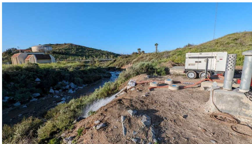
Staff dewatering the AMP to prepare for relining work
