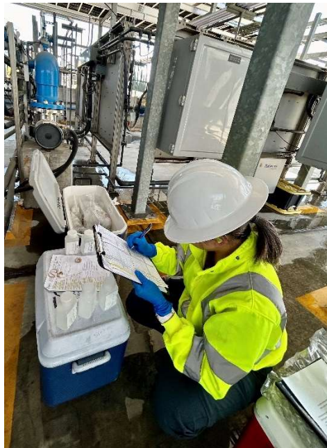
Staff collect samples to evaluate performance of the MBR-based treatment train at the NIC demonstration plant
