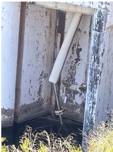
Damaged gate shaft (left and center) and as-found actuator assembly (right) for the gate at Copper Basin
