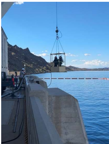
Divers being lowered in the water to dredge galleries (left), removed debris (center), and the repaired buoy line (right) at Intake pumping plant
