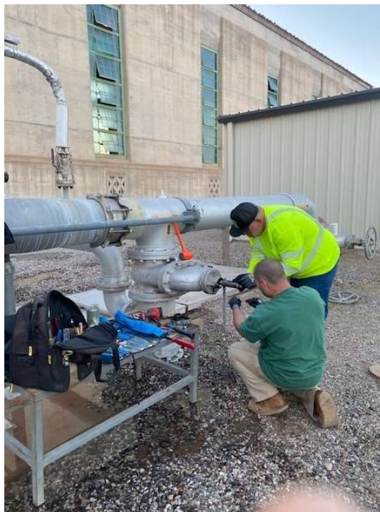
Staff repairing a circulating water valve at Gene pumping plant
