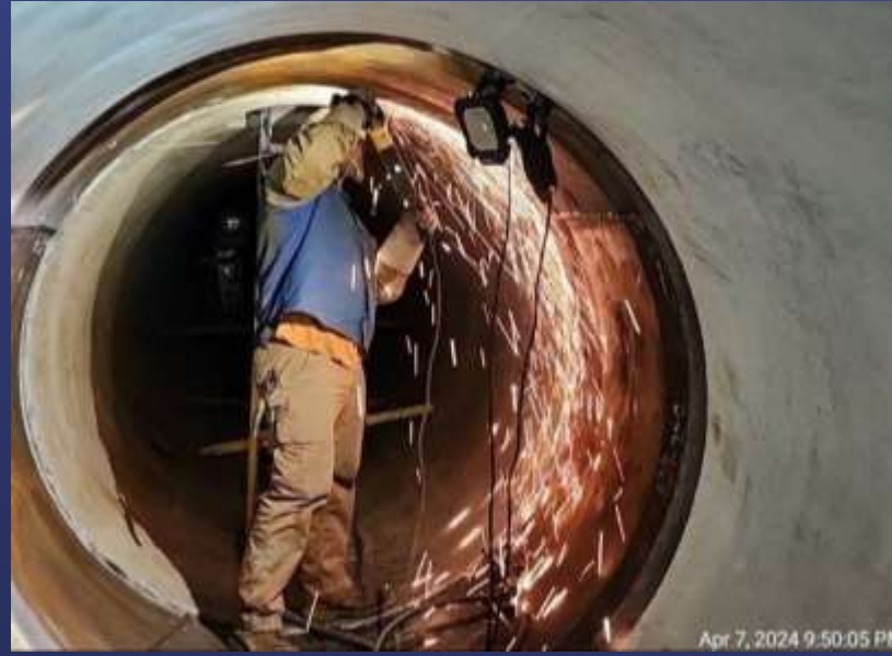
Welding new steel liner pipe
