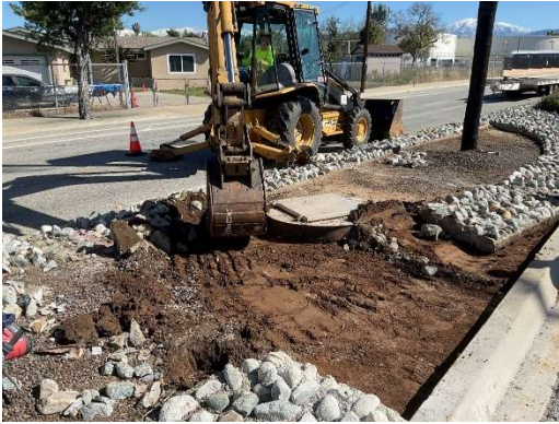
Staff excavating concrete slab area (left) and reinforcing wire installation (right) to enhance safe access at a Middle Feeder structure
