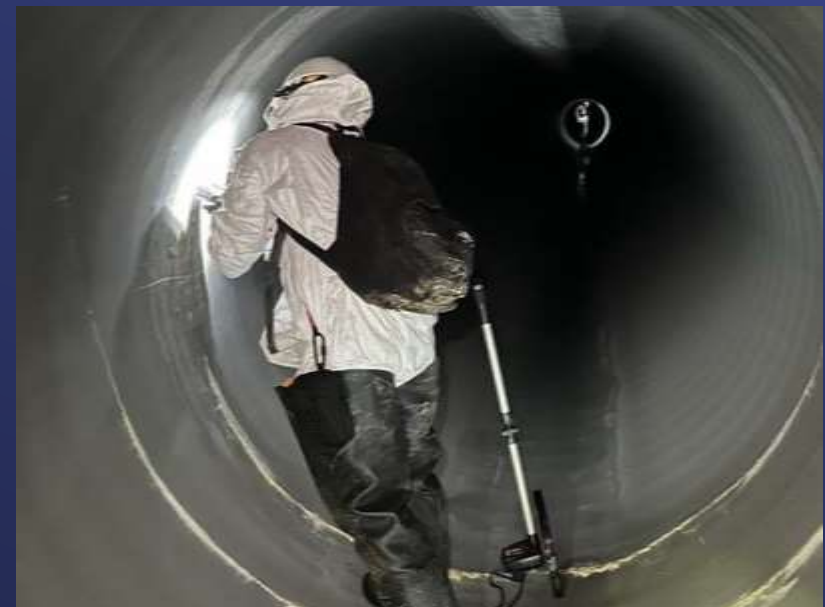
Second Lower Feeder Coating
