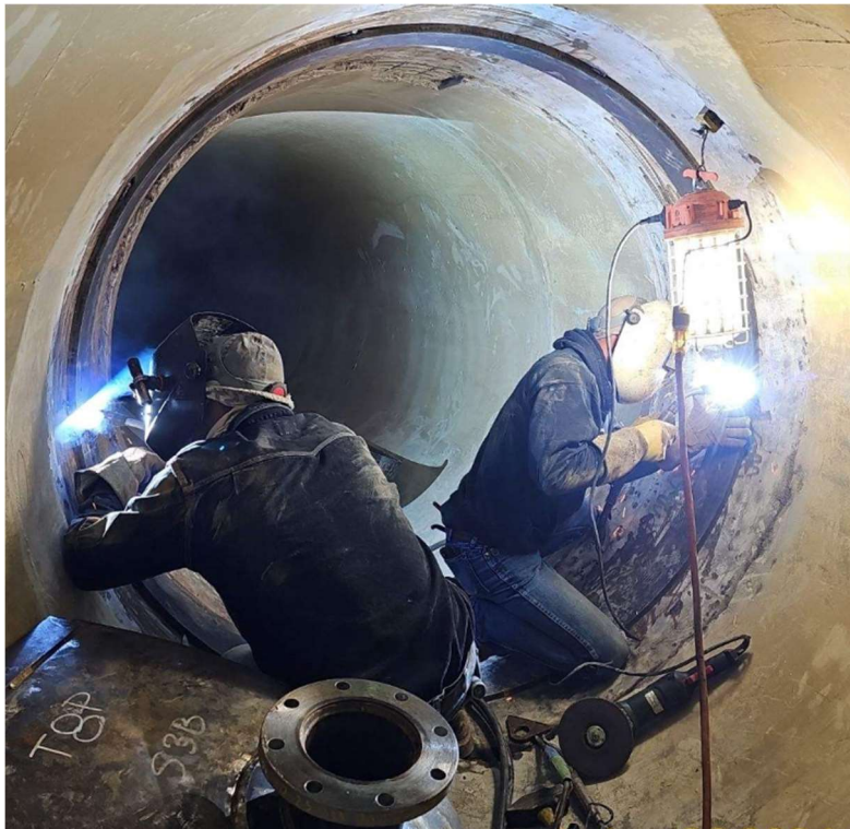
Allen-McColloch Pipeline Urgent PCCP Rehabilitation—Welding of Steel Band for Bulkhead
