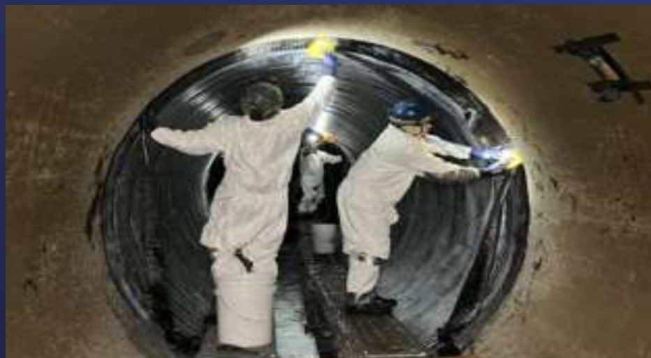
Sepulveda Feeder Carbon Fiber Lining
