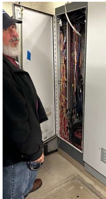
Staff opening vaults and cabinets to identify fiber optic cables
