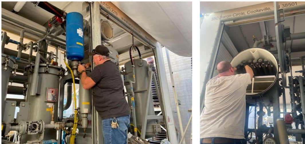
Staff maintaining the oil purification unit prior to operation
