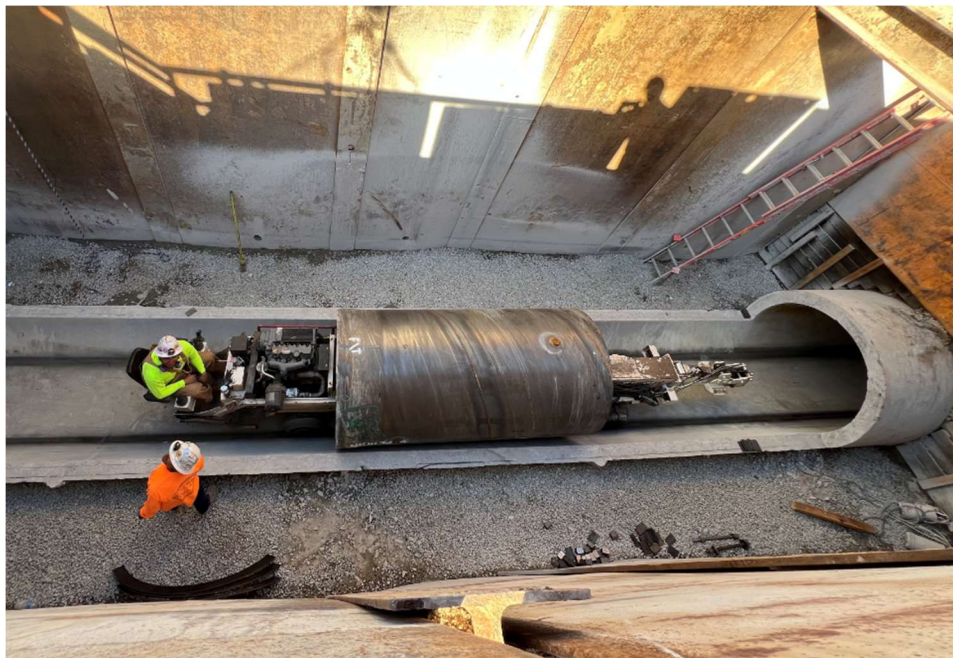
Allen-McColloch Pipeline Urgent PCCP Rehabilitation–Installation of Liner Pipe
