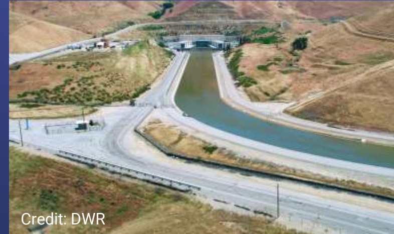
Edmonston Pumping Plant
