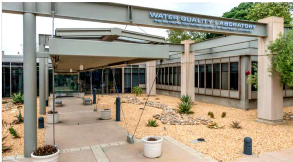
Main Entrance to Water Quality Laboratory Building
