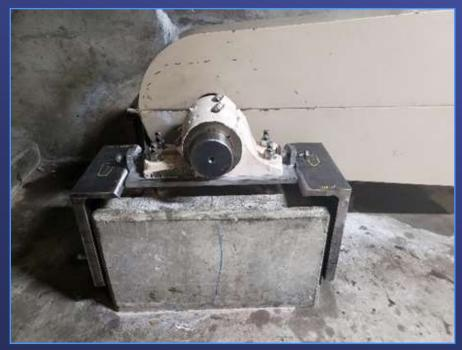
Structural reinforcement at bearing completed at Basin 10
