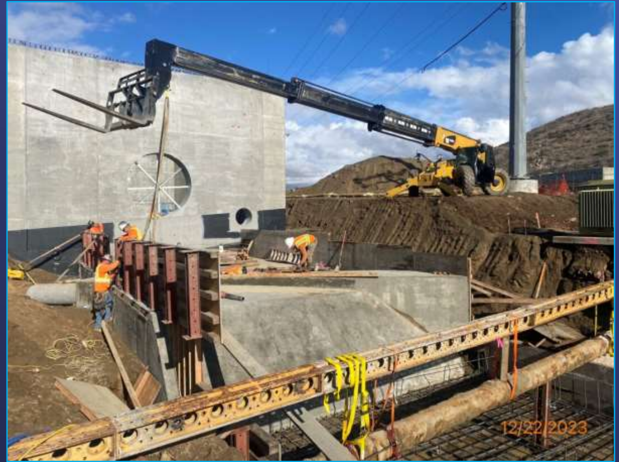
Wadsworth Bypass Pipeline
