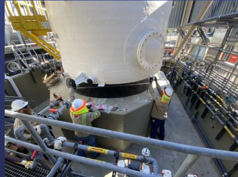
Garvey Reservoir Hypochlorite Tank Installation
