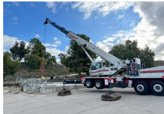
Inside view with scaffolding installed (left) and 100-ton crane setup for lid removal (right) at OC-88 valve structure along the AMP
