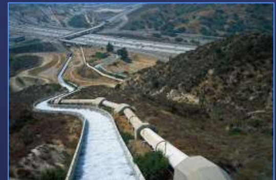
Los Angeles Aqueduct
