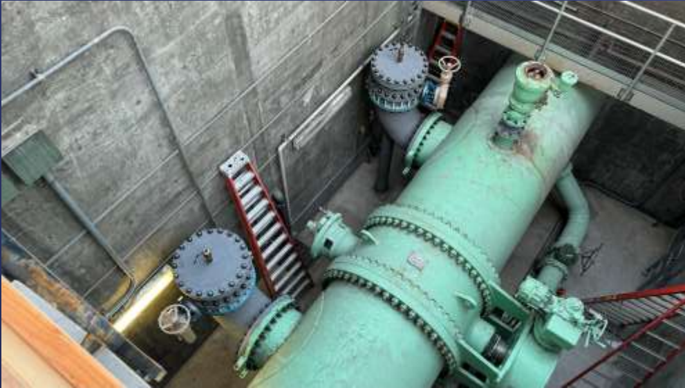
66-inch Valve Vault prior to installation of Cla Valve
