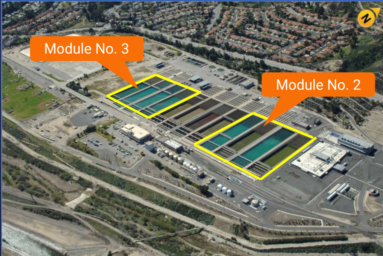
Jensen Modules 2 & 3 Sedimentation Basins
