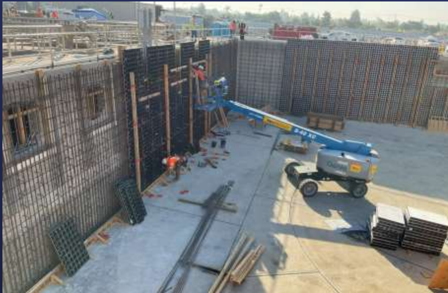
Weymouth Basins 5-8 – Wall Strengthening
