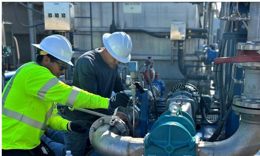
Staff repairing a pump at the Napolitano Innovation Center demonstration plant
