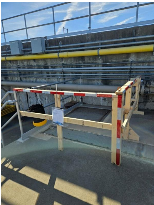
Temporary handrail and gratings installed for worker safety
