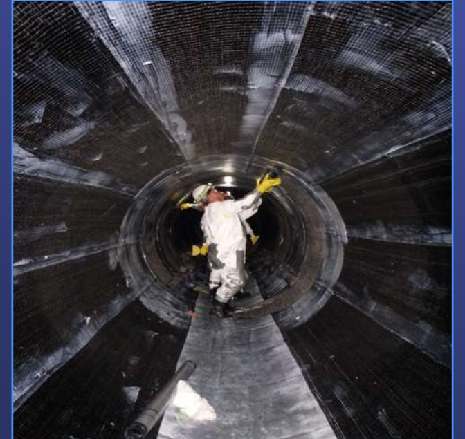
Carbon Fiber Rehabilitation Second Lower Feeder
