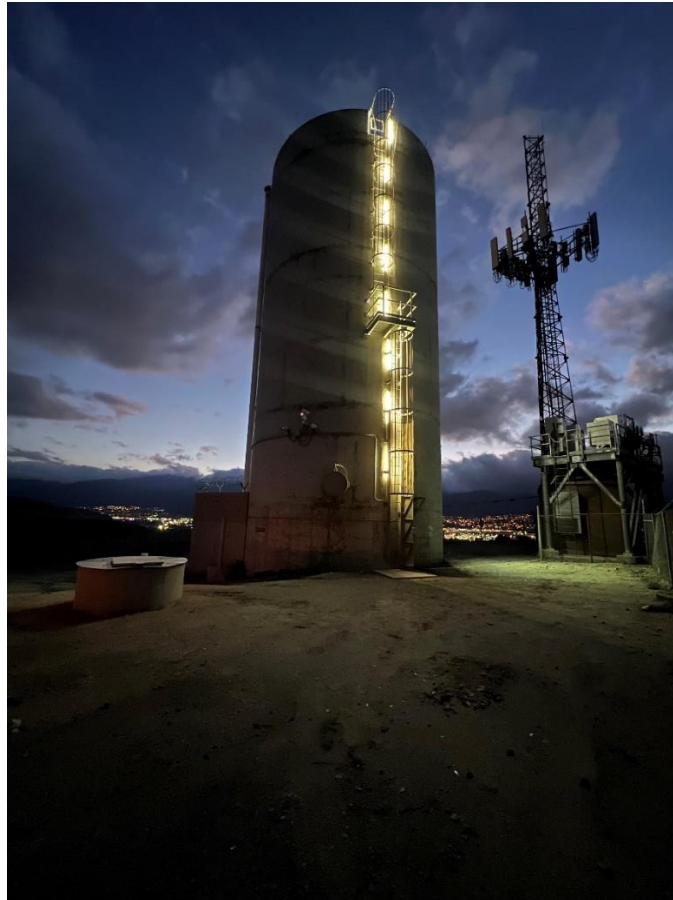
Temescal Hydroelectric Plant tower lit up with the sun setting in the west
