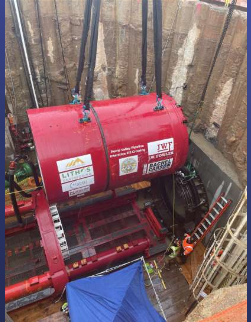
TBM Lowered into Launch Shaft
