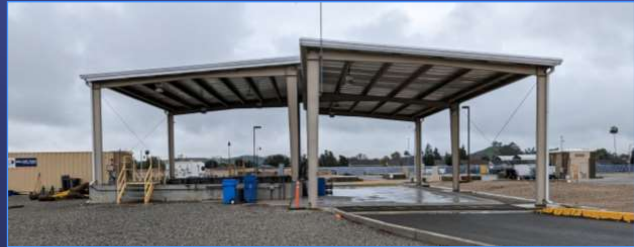
Existing Decommissioned Sulfuric Acid Tank Farm
