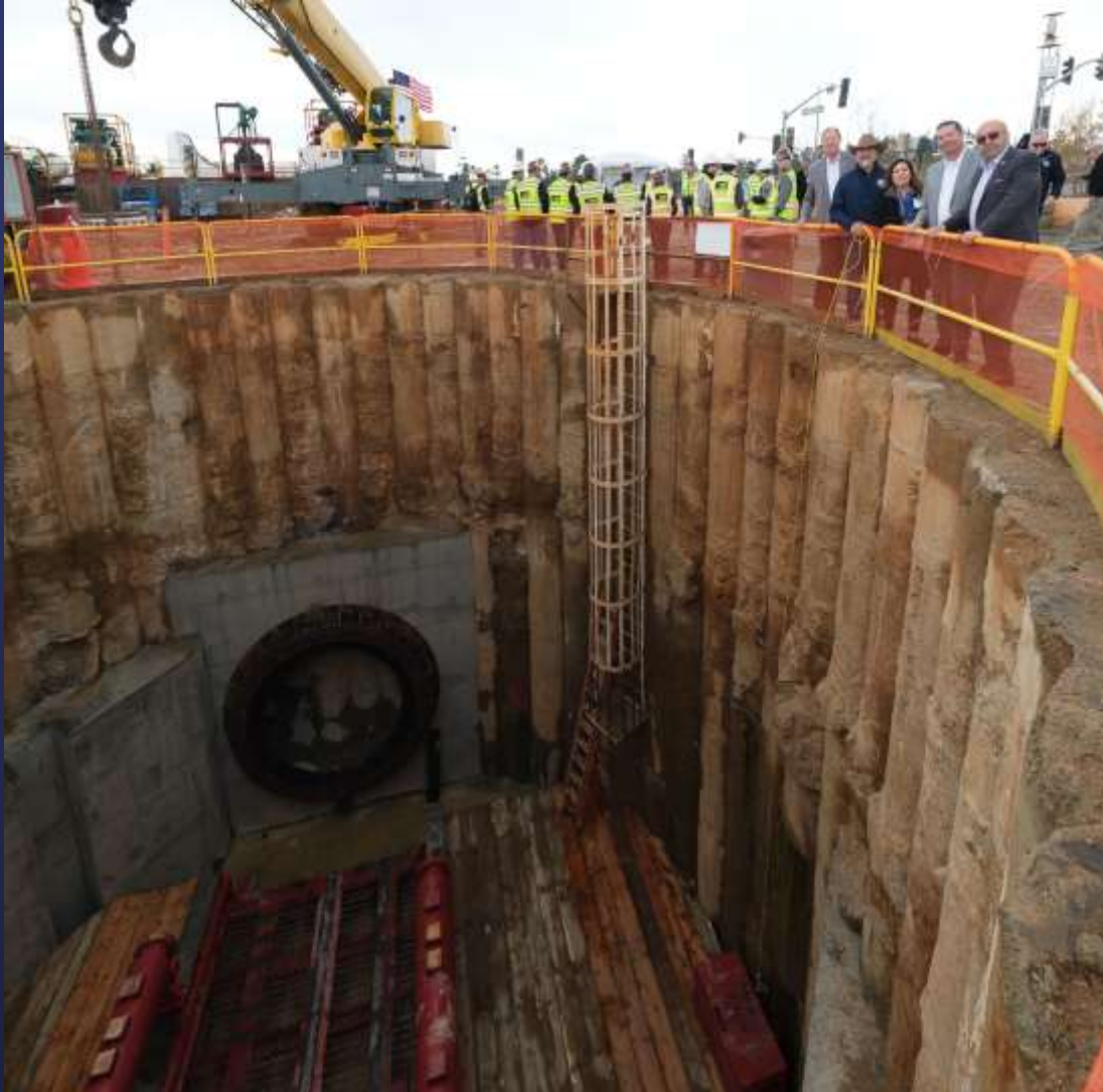
Tunnel Launch Shaft
