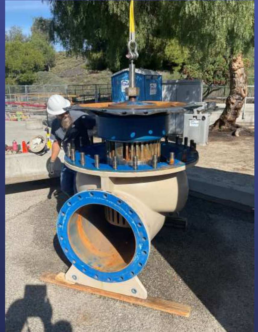
Inspection of 24-inch Cla Valve
