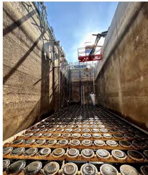
New foam skimming equipment is installed in the aerobic tank at the demonstration plant
