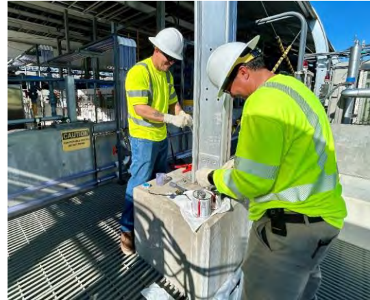
Staff fits PVC piping for new chemical feed lines at the demonstration plant
