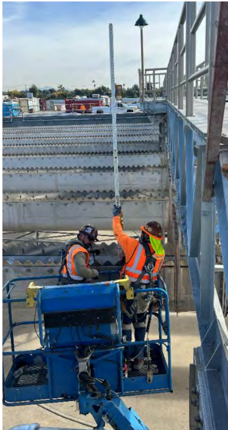
Weymouth Basins 5–8 and Filter Building No. 2 Rehabilitation—Basin 7 Weir plate installation
