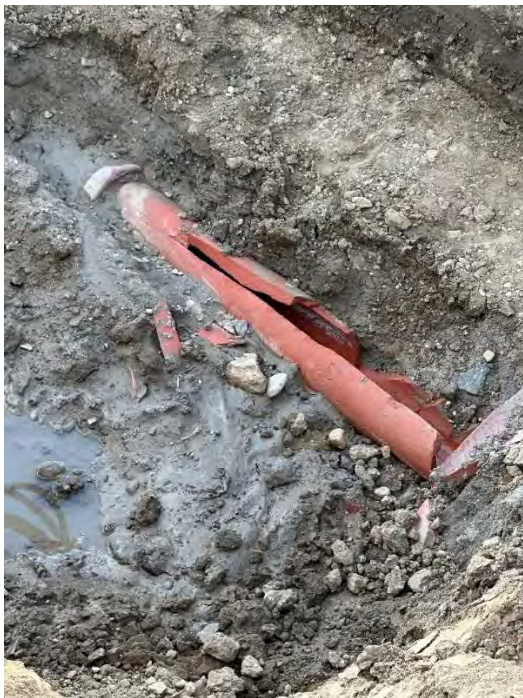
Damaged sewer line at Diemer plant
