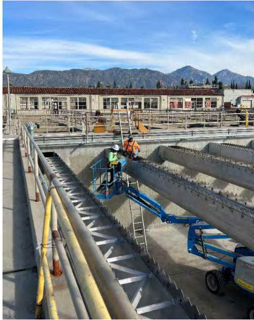
Weymouth Basins 5–8 and Filter Building No. 2 Rehabilitation—Launder and weir installation
