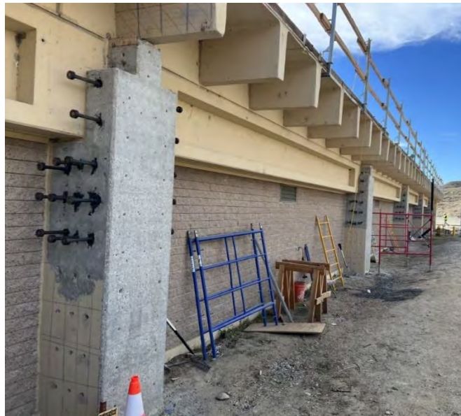
Foothill Hydroelectric Power Plant —Installation of Seismic Reinforcing
