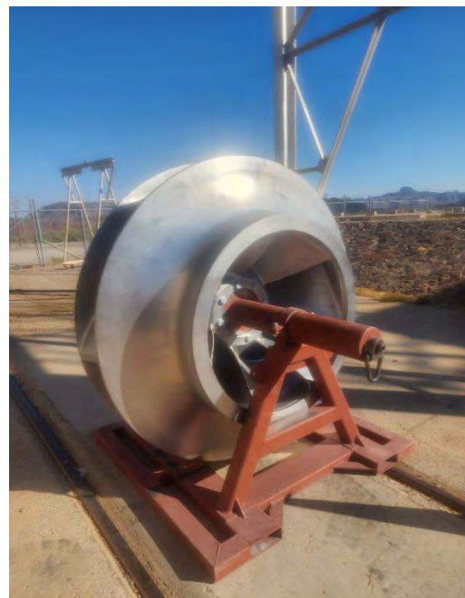
Main pump impeller cleaning and repair at Eagle Mountain pumping plant
