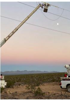
Broken static line (left) and staff splicing the static line (right) on the 230kV CRA transmission system
