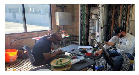
Staff land wires for installation of new remote terminal unit (RTU)
