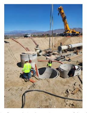
Staff removing flanges during dewatering process of the Inland Feeder
