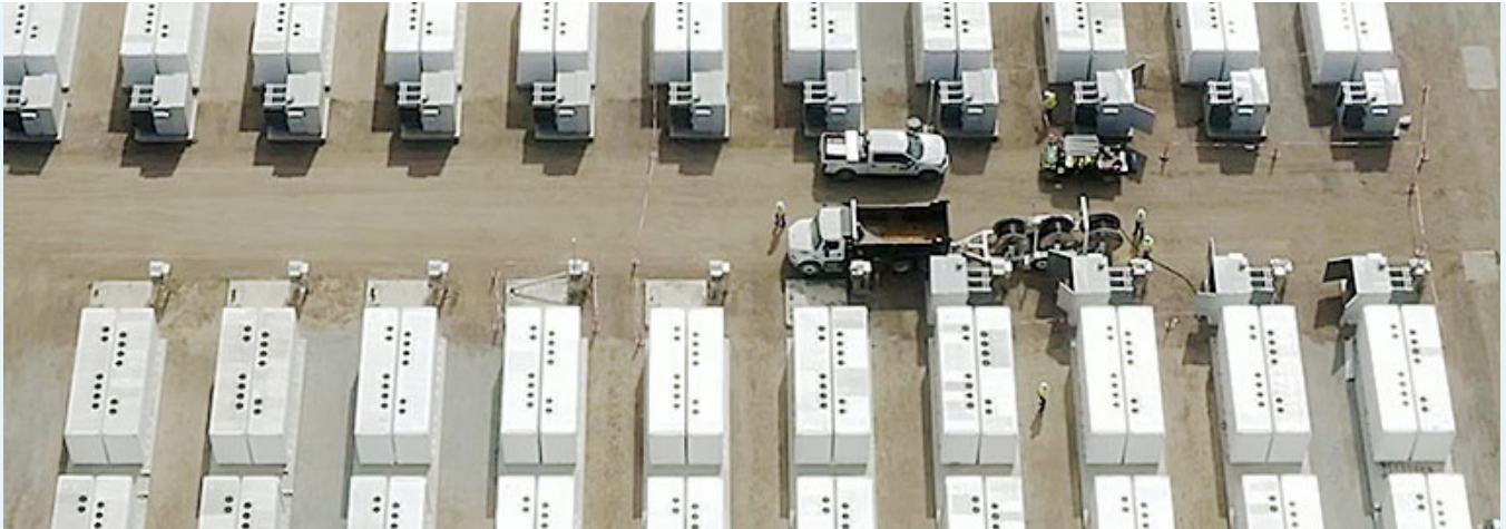
Photo of PG&E's Elkhorn Battery in Monterey County, a 182.5 MW battery energy storage system that is one of the largest utility-owned, lithium-ion battery energy storage systems in the world.
