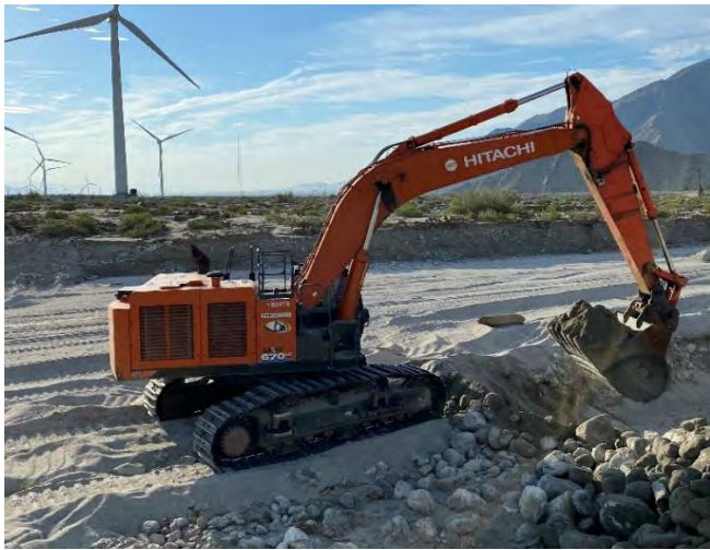
Excavator (left) and dozer (right) working to restore canal berms leading to the Whitewater groundwater recharge facility
