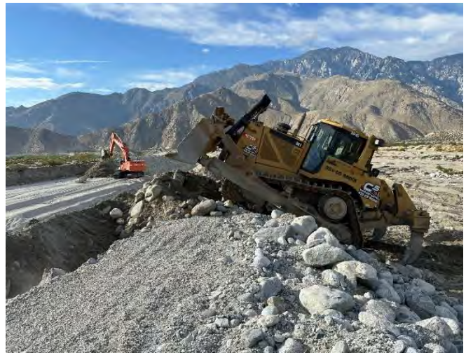
Excavator (left) and dozer (right) working to restore canal berms leading to the Whitewater groundwater recharge facility
