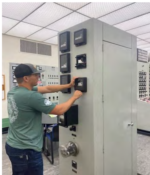
Staff testing and calibrating a protection relay for a 9,000 HP motor at a CRA pump plant
