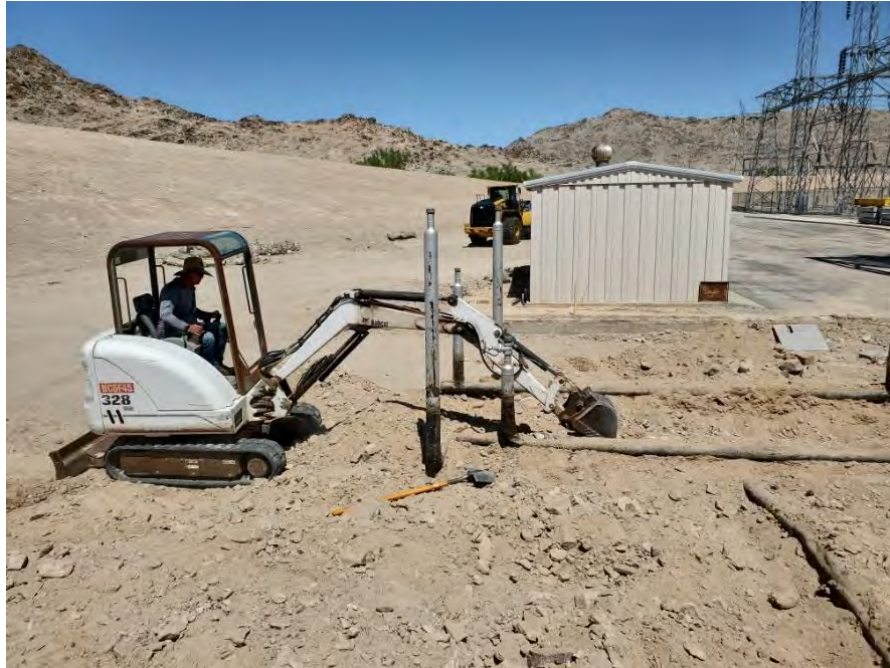
Staff demolishing an obsolete piping system at a CRA pump plant
