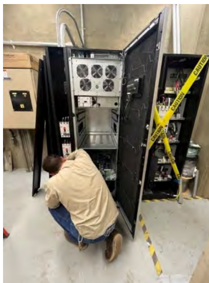
Skinner staff installing 50 kVA UPS unit at Red Mountain Hydroelectric Power Plant
