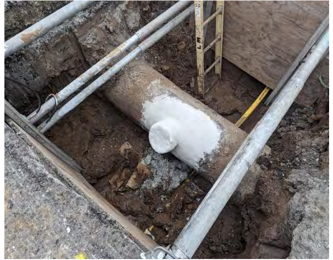
Flushing to disinfect pipeline (left) and mortar cap (right) post-repair on the Compton Lateral
