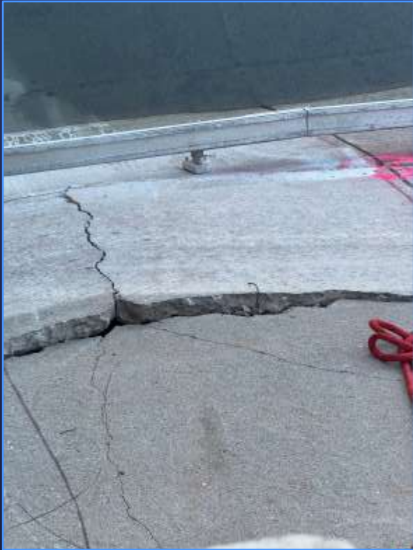
Example of buckled concrete canal panels
