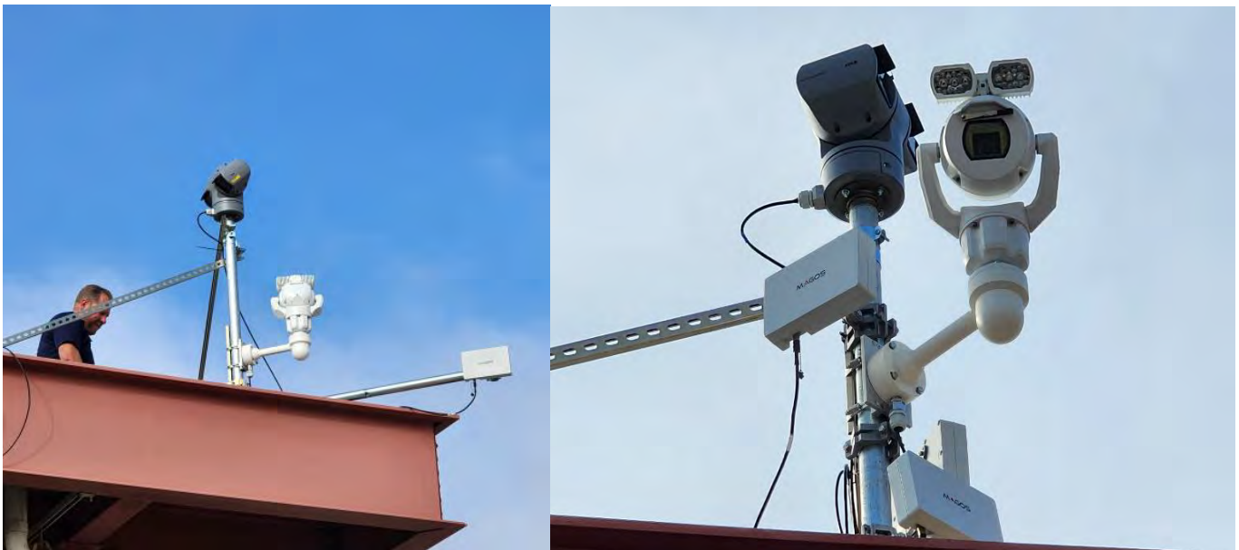
Jensen's pilot project includes innovative, ground-based radar systems
